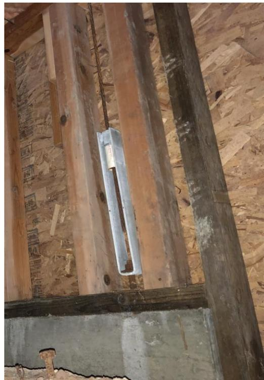
Figure 9. – Typical holddown in crawlspace
