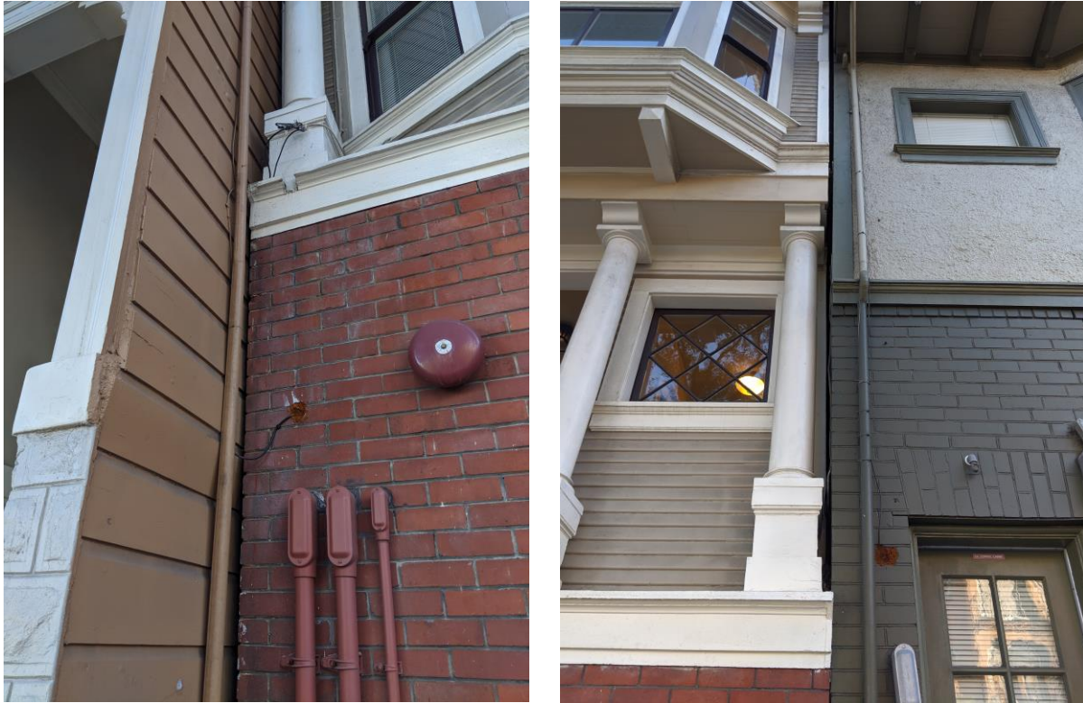
Figure 6 - Building Separation to the North (Left) and South (Right)
