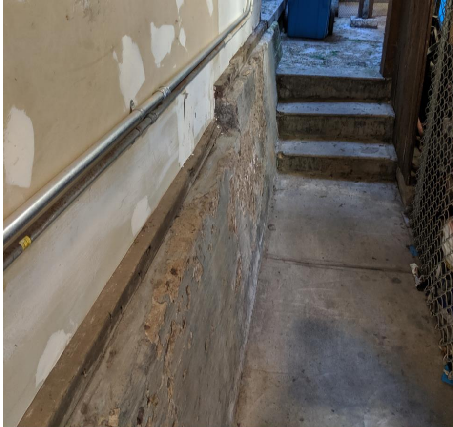
Figure 12 - Concrete Stem Wall on North Side of Building
