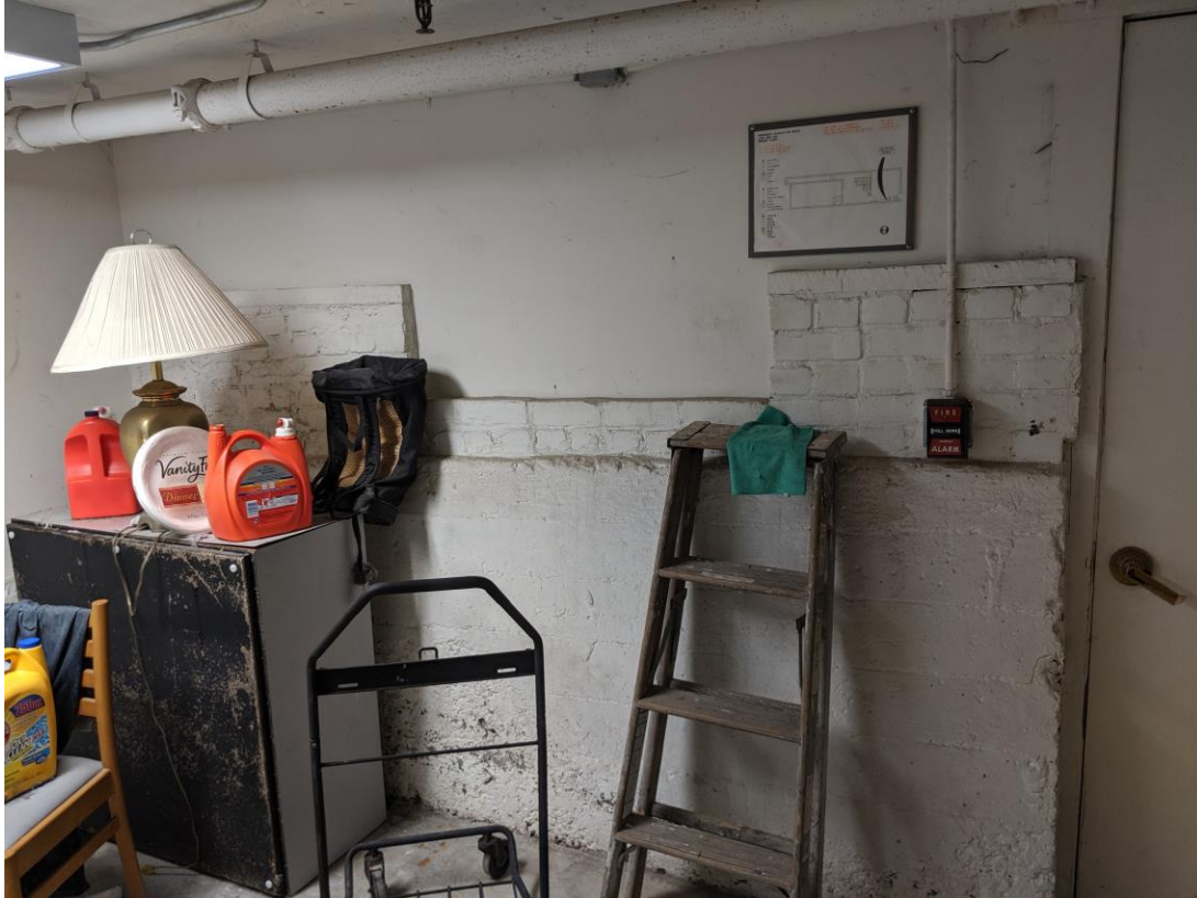
Figure 9 - Area of Brick Wall Over Concrete Stem Wall in Basement
