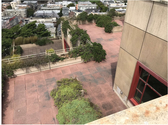
5 th floor & 4 th floor south terraces
