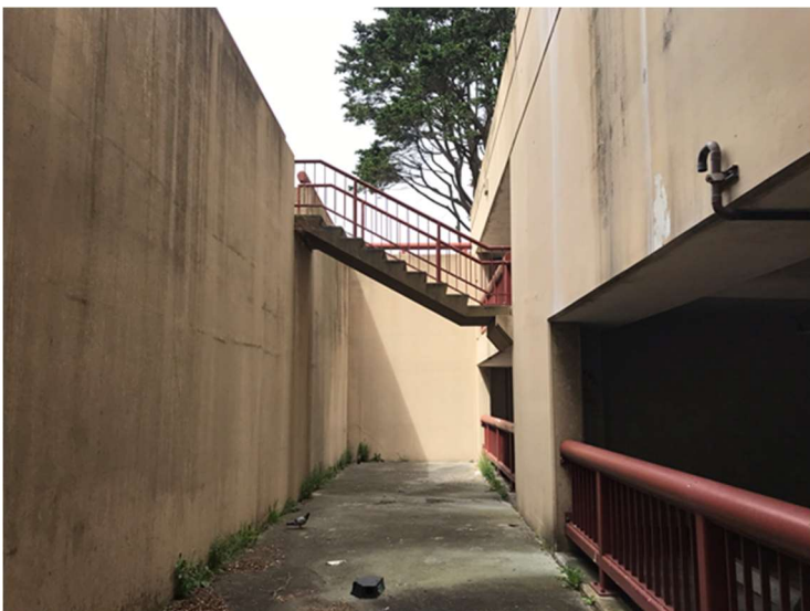
West side areaway at parking levels E & F
