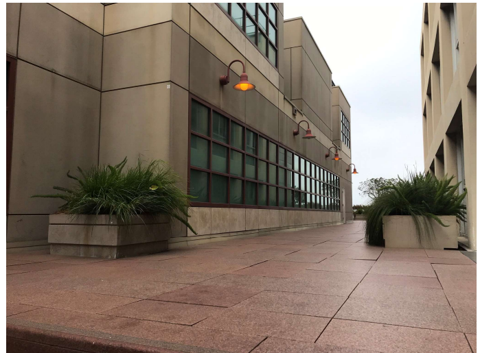
Partial east elev. & 4 th floor terrace (Millberry building at right)
