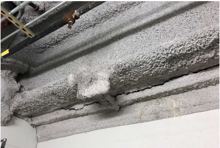
Out-of-plane wall anchor at north CMU wall
