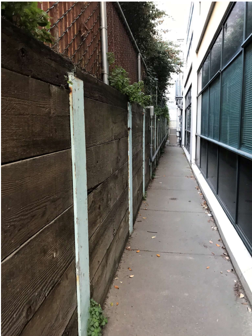
Retaining wall at west property line
