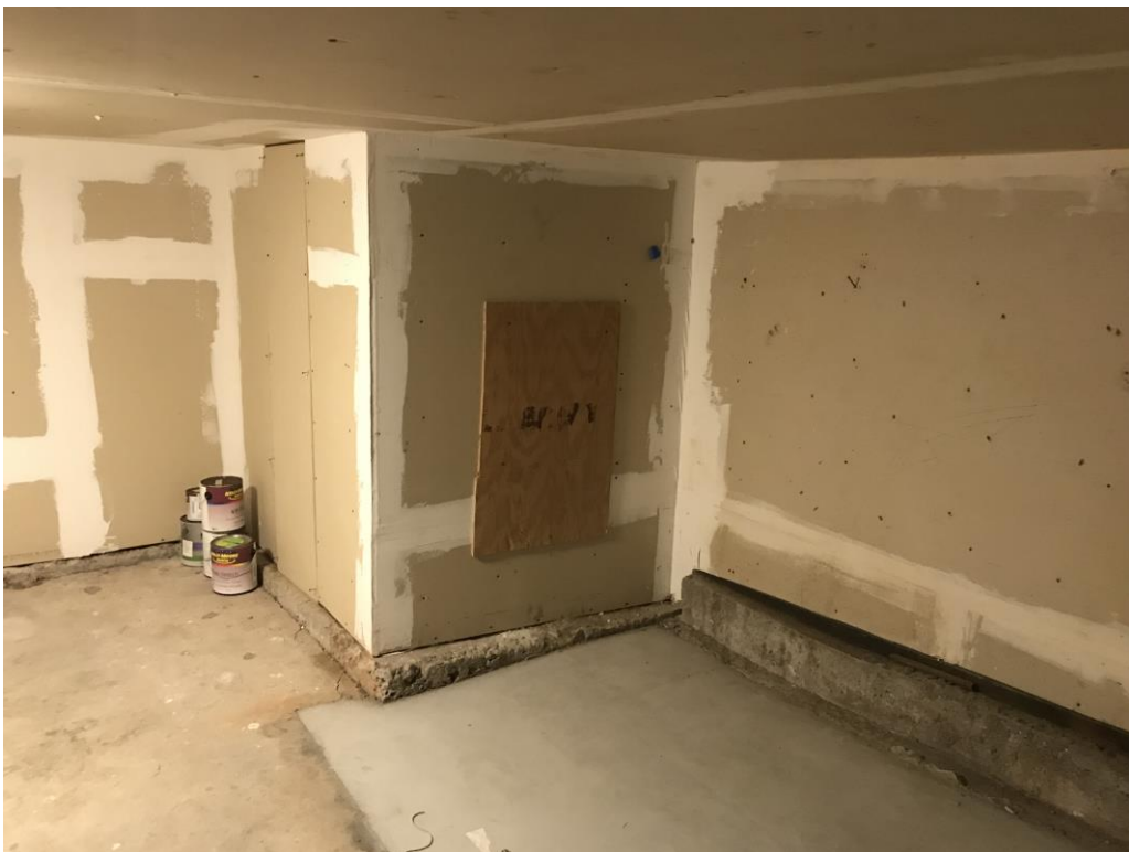
Figure 7 – Storage Area of Basement with Gyp Board
