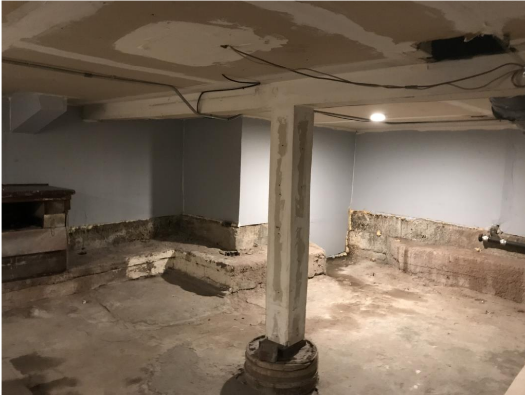
Figure 10 – Interior Basement Post
