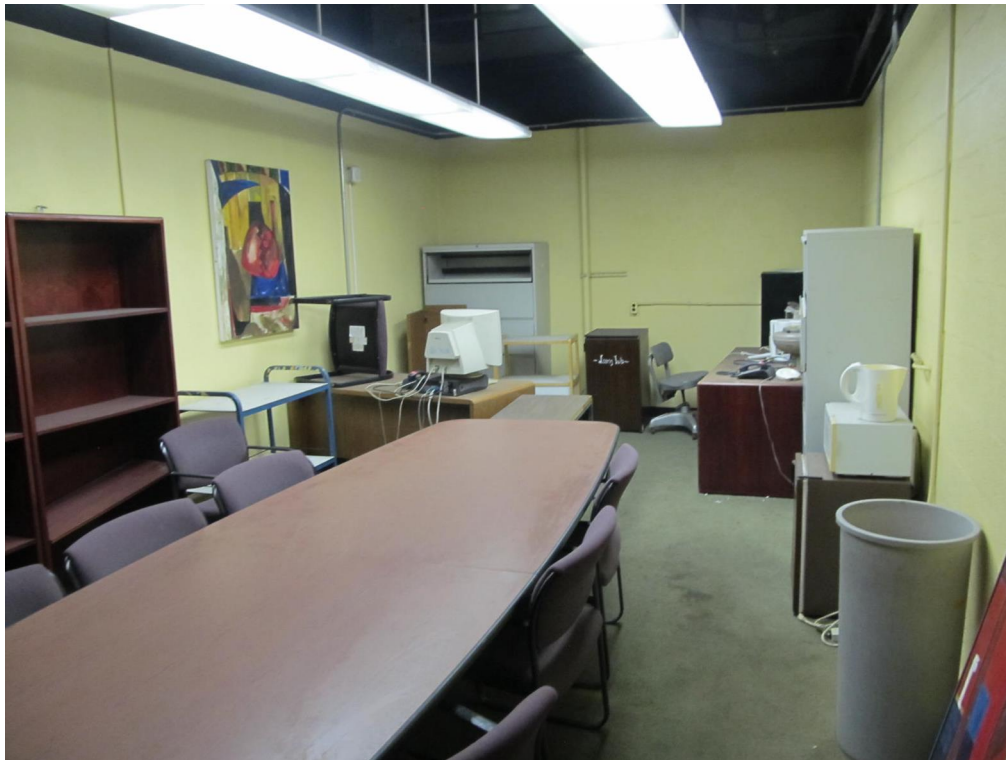
South wing of Building E (looking northeast)
