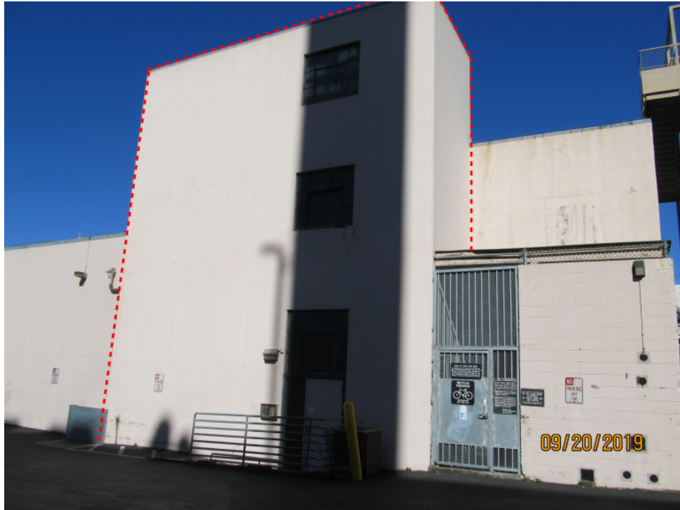
Stair tower within dashed redlines on west elevation added after the 1962 alterations (looking northeast)
