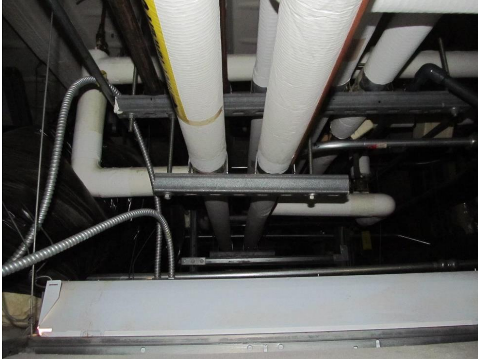
MEP bracing at first story above the lay-in ceiling (looking west)
