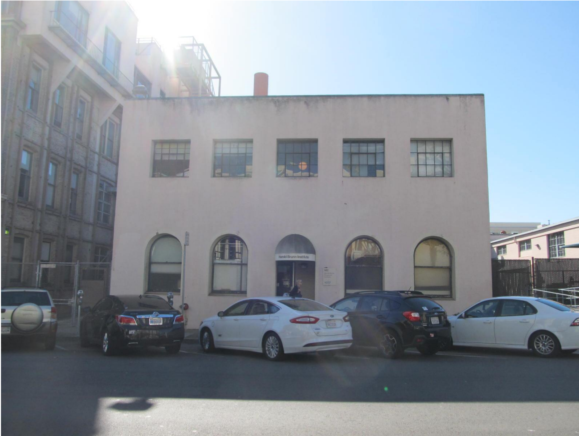
East elevation (looking west)
