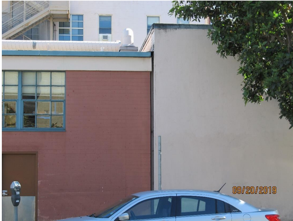
Seismic joint between Building G and Building E (looking south, Building G on the left and Building E on the right)
