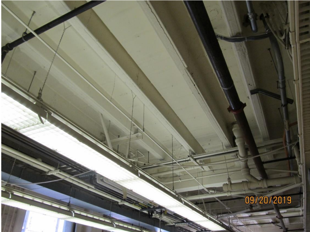
Typical concrete framing on the underside of second floor
