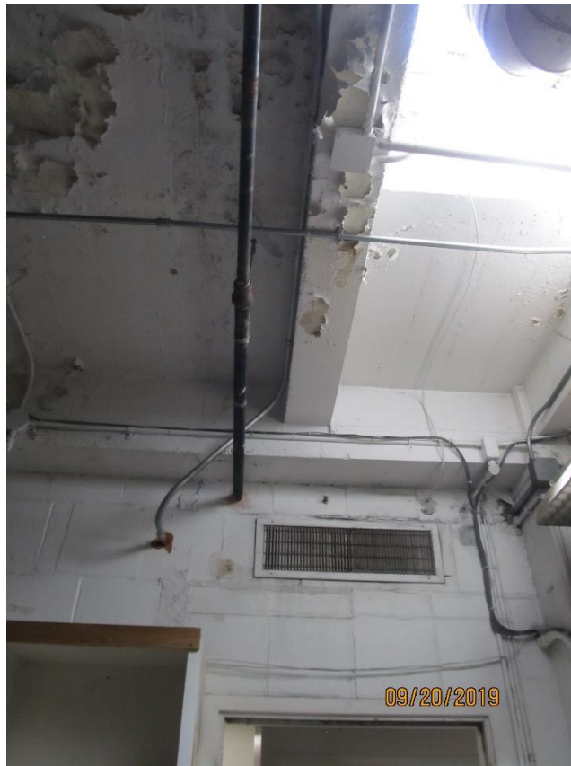
Hollow clay tile partitions at second story (looking north)
