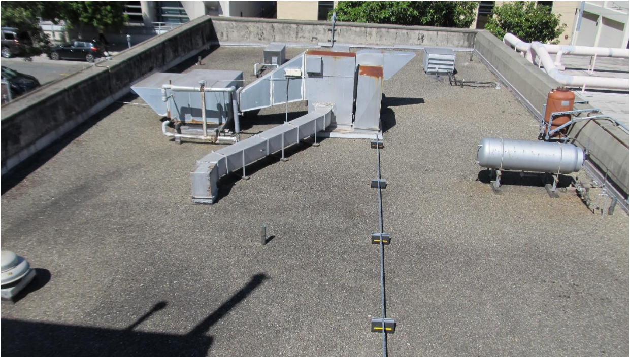
Roof at north wing of Building E (looking north)
