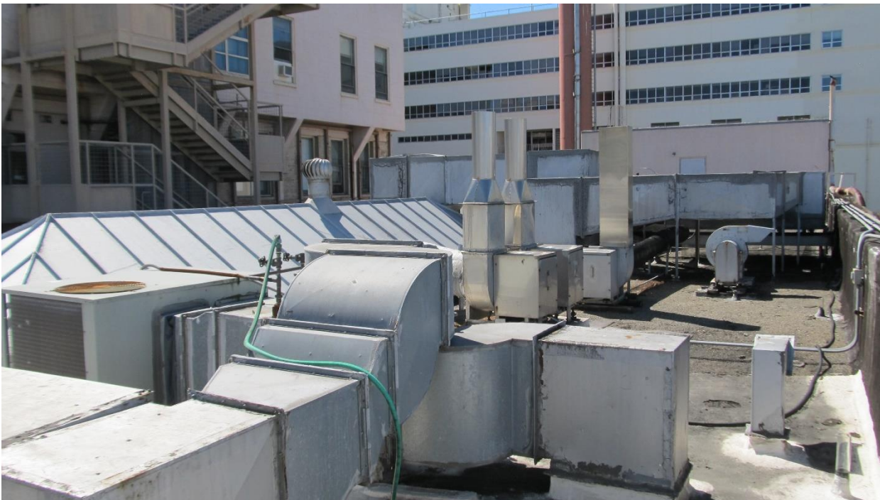
Roof at south wing of Building E (looking southwest)
