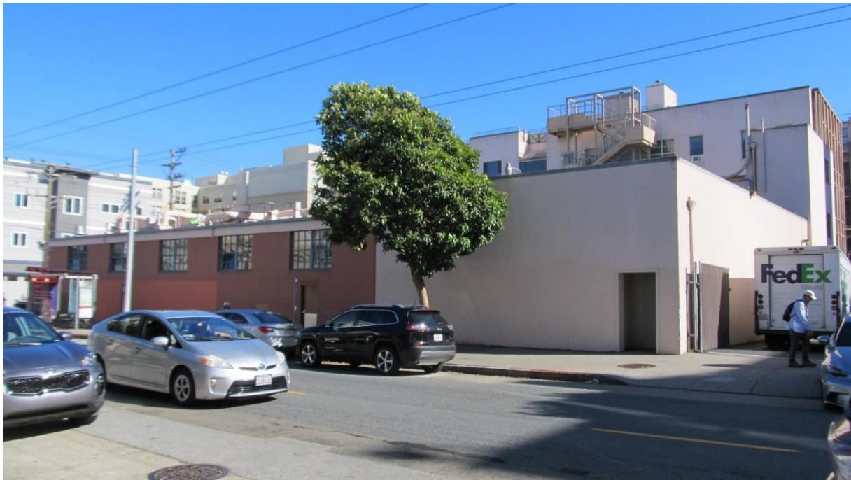
North elevation (looking southeast on Sutter Street)
