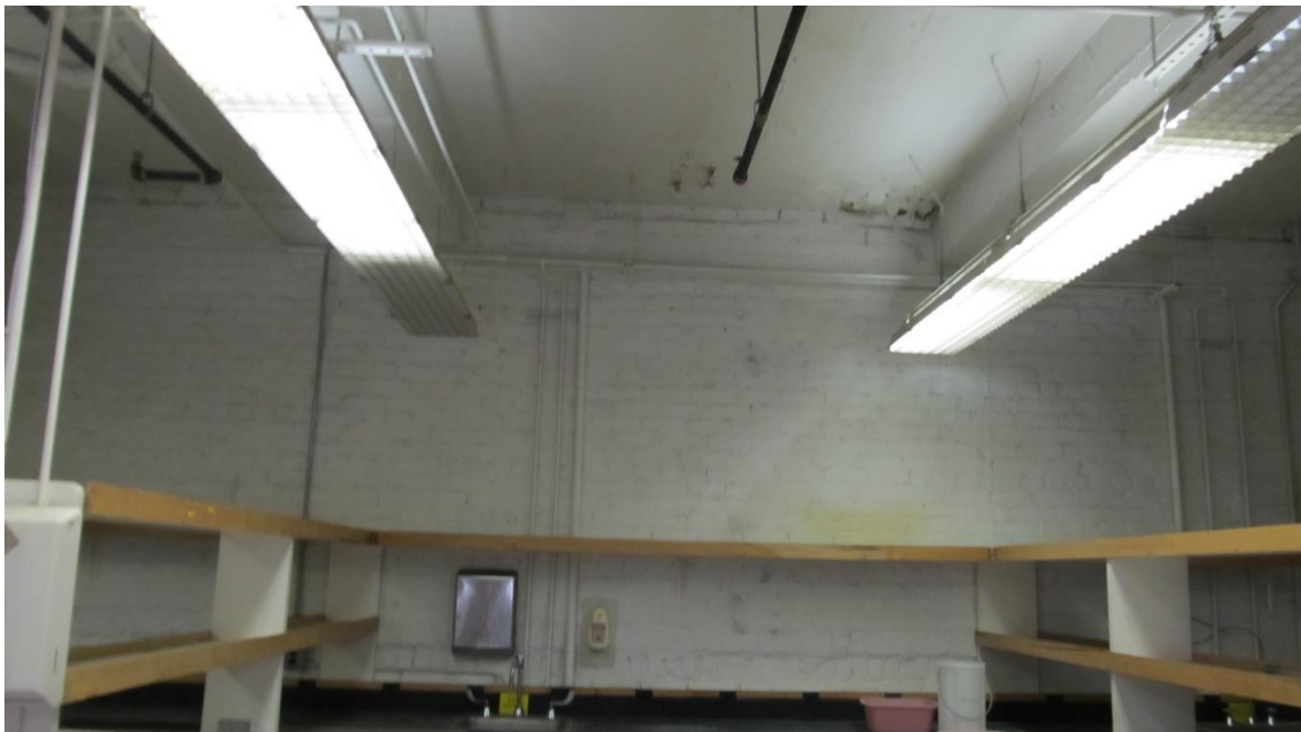
Concrete slab over beams with URM infill wall at second floor
