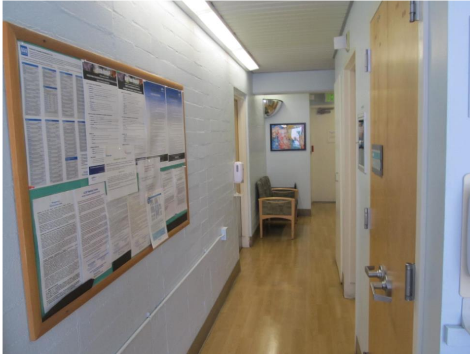
Offices below the east mezzanine (looking north)
