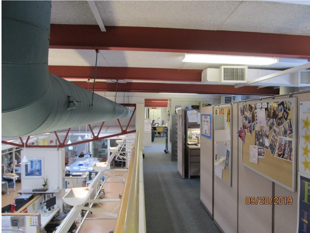
Interior looking west (mezzanine on the right and first floor on the left)
