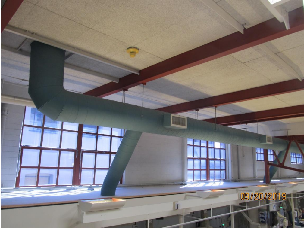
Interior of south elevation with soffit (looking southwest)
