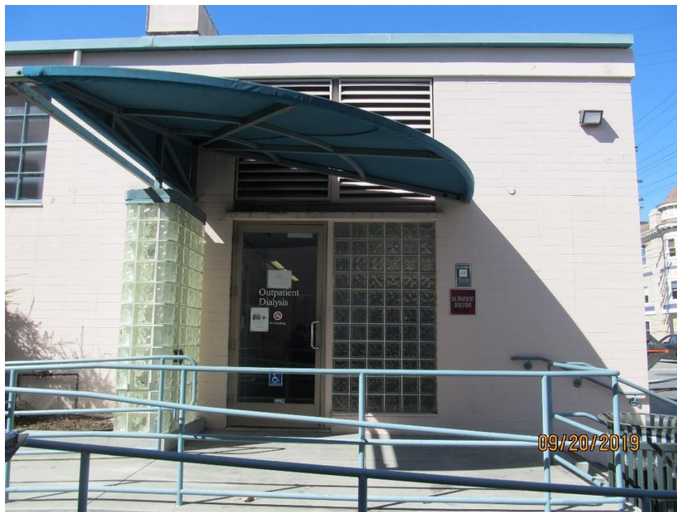
Main entrance on south elevation (looking north)
