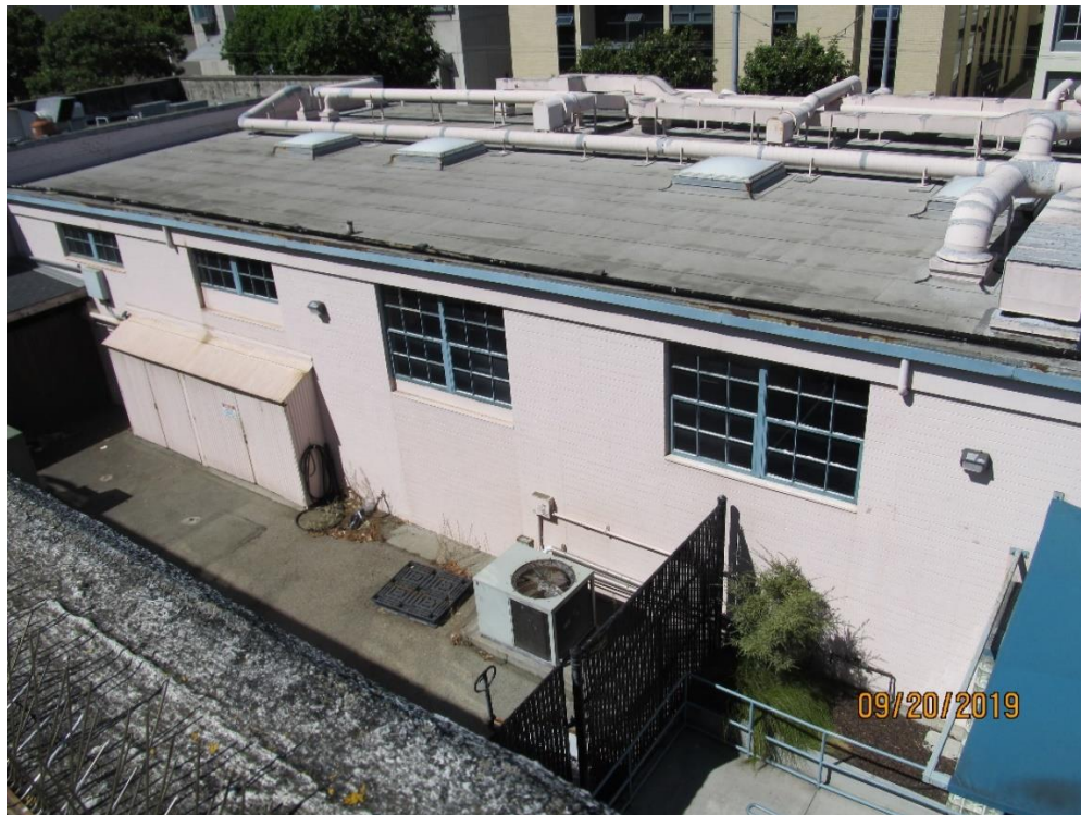
South elevation and courtyard (looking northwest)
