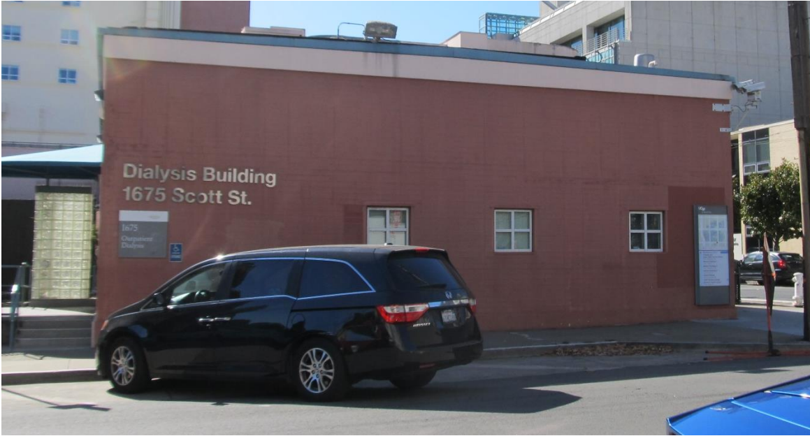
East elevation (looking west)
