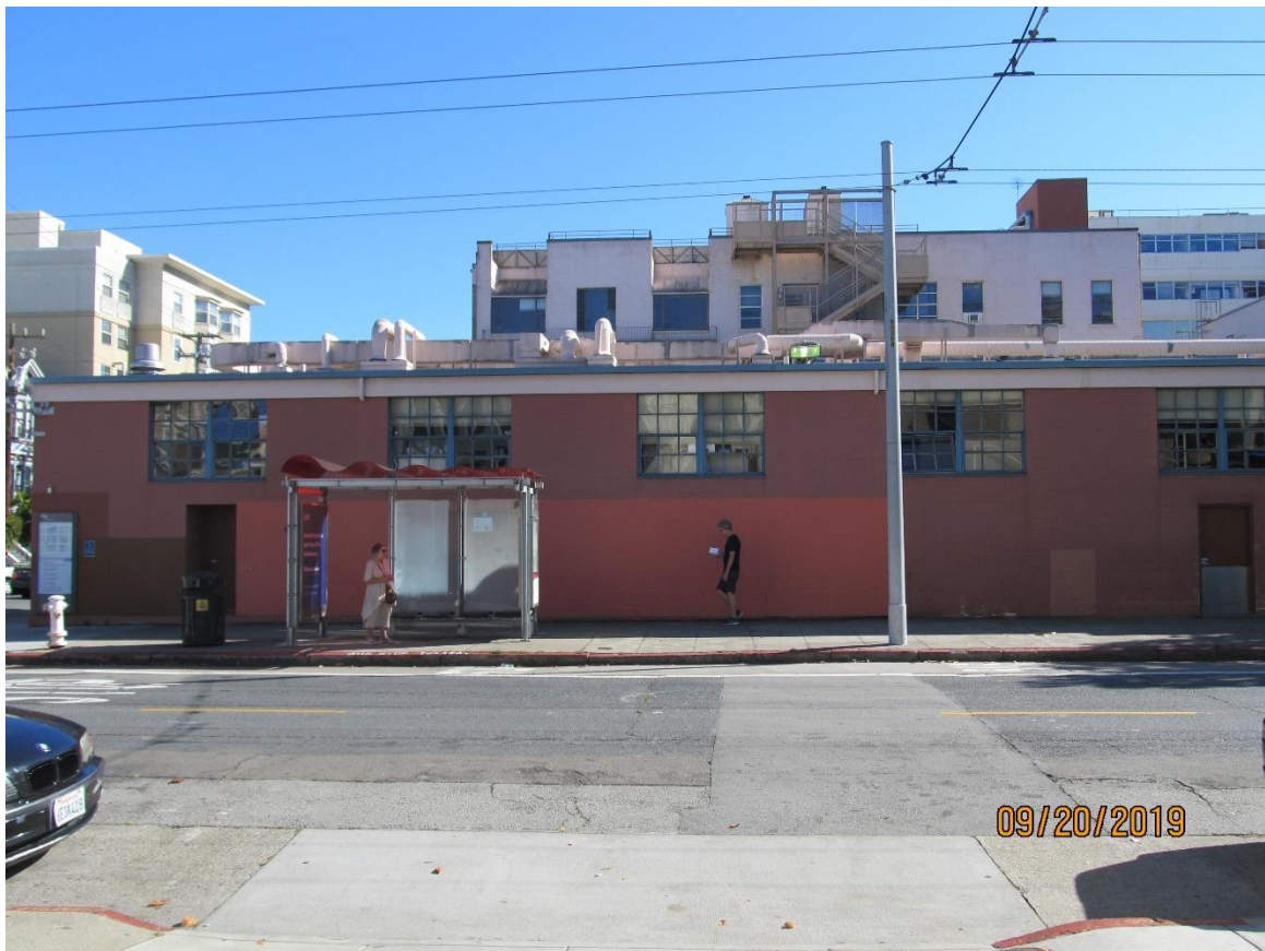
North elevation (looking south)
