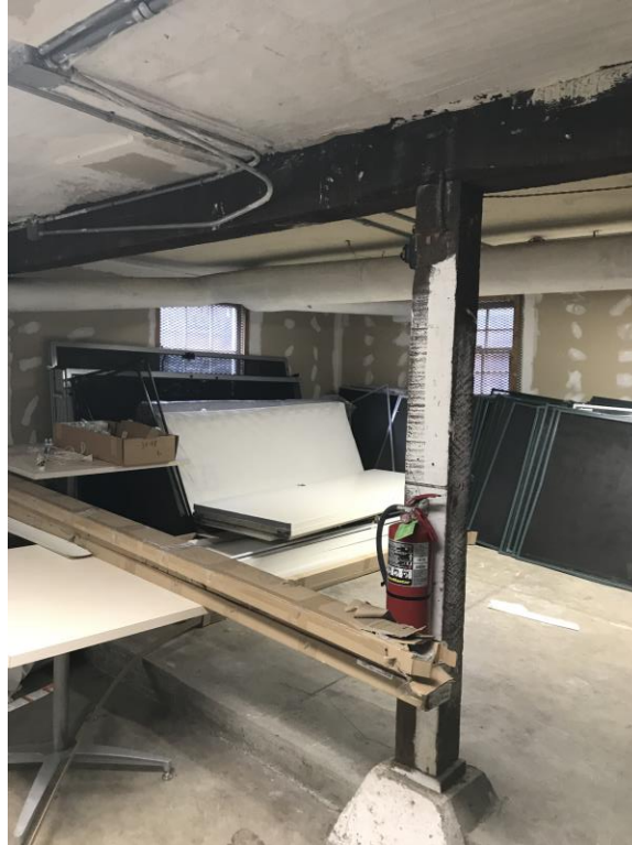
Figure 10 – Typical Interior Basement Post Without Connectors
