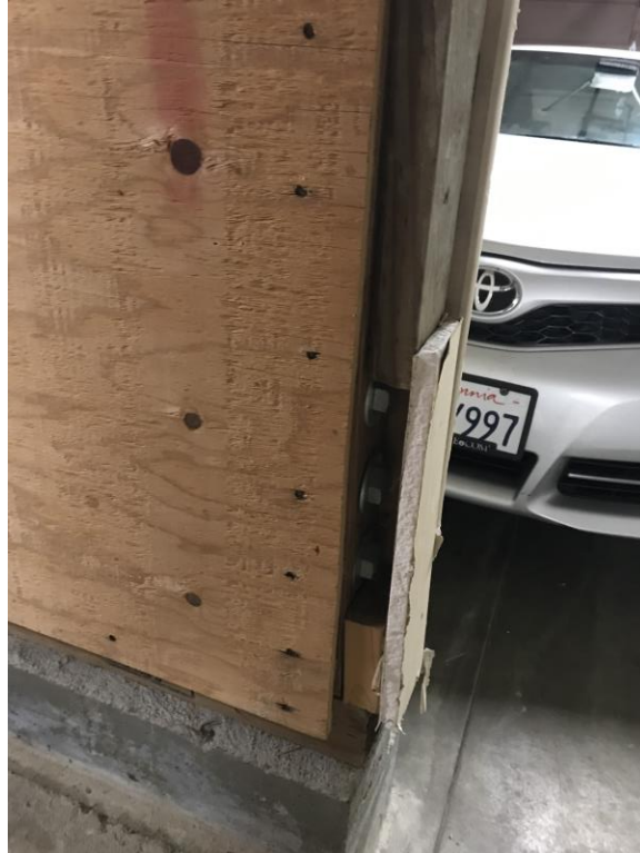
Figure 8 – New Transverse Plywood Shearwall Holddown Hardware
