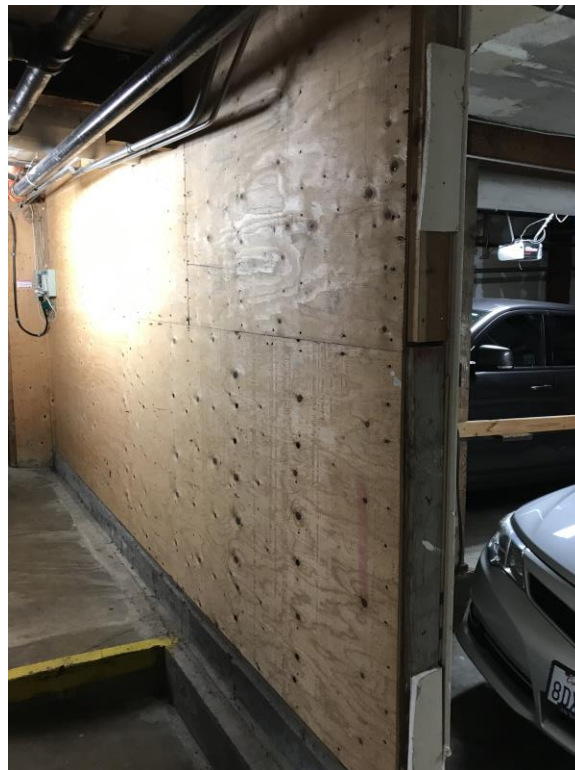
Figure 7 – New Transverse Plywood Shearwall
