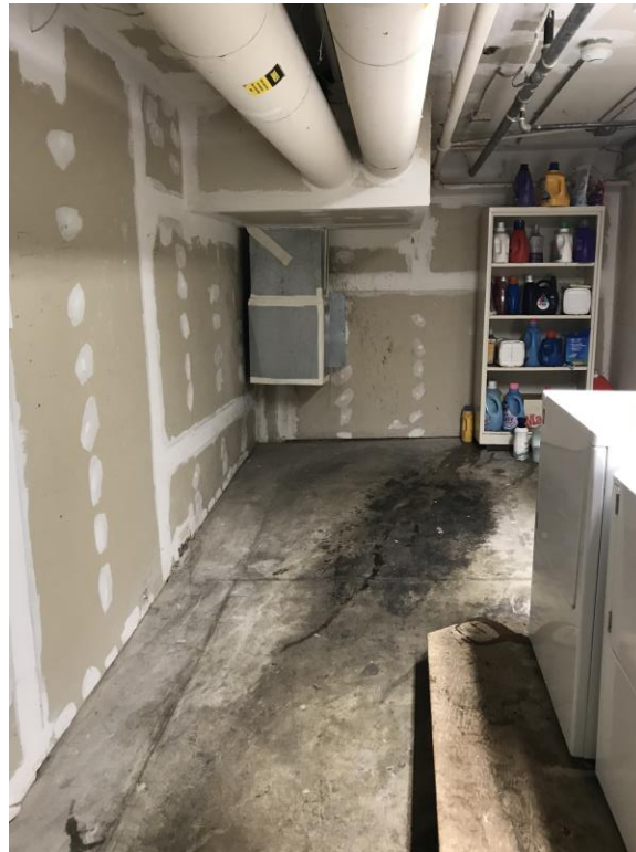
Figure 6 – Basement Laundry Room
