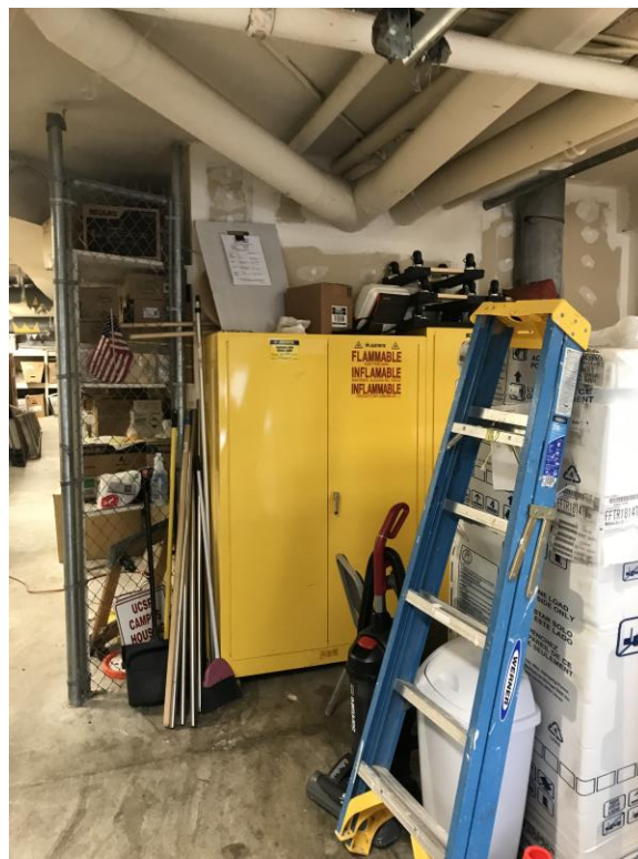
Figure 7 - Flammable Material Storage in Garage
