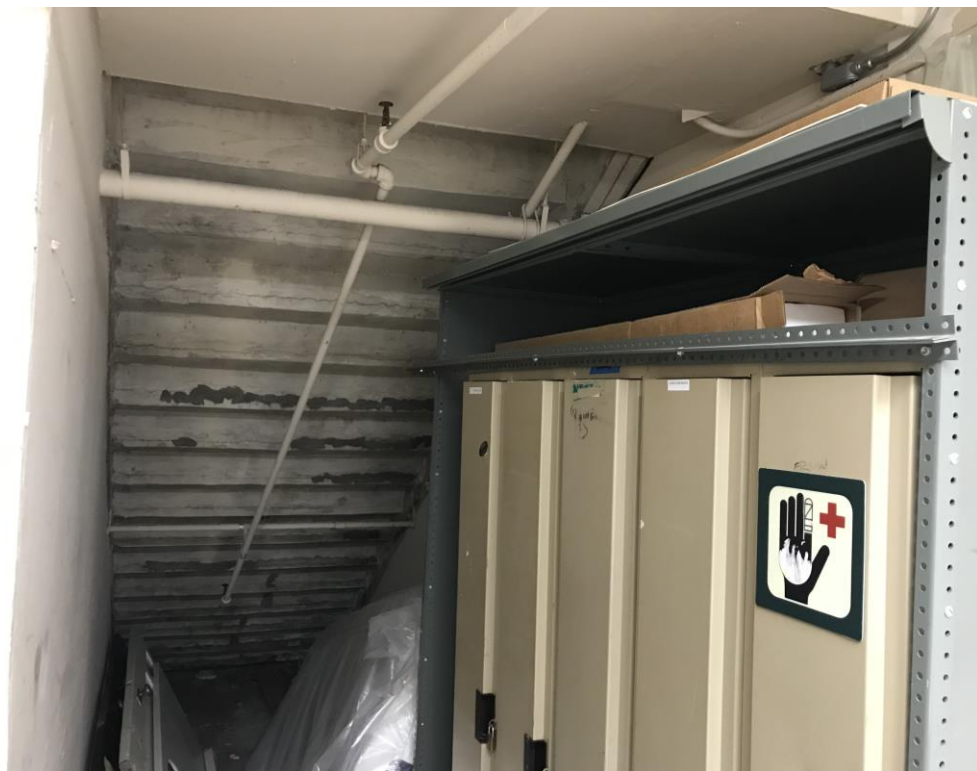
Figure 9 – Underside of Main Entry Stairs
