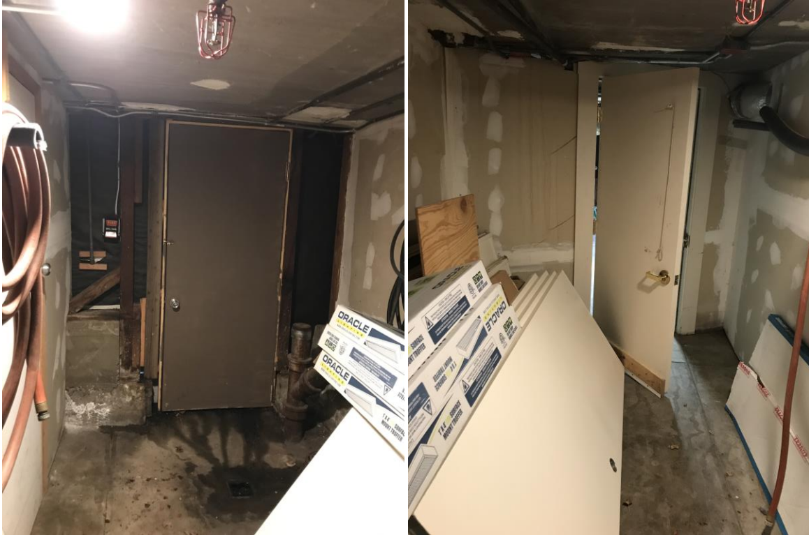
Figure 11 – Rear Hallway. Left: Looking East. Right: Looking West
