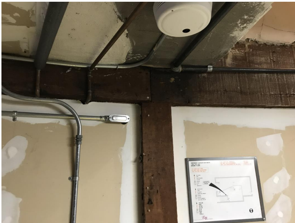
Figure 12 – Top of Basement Post
