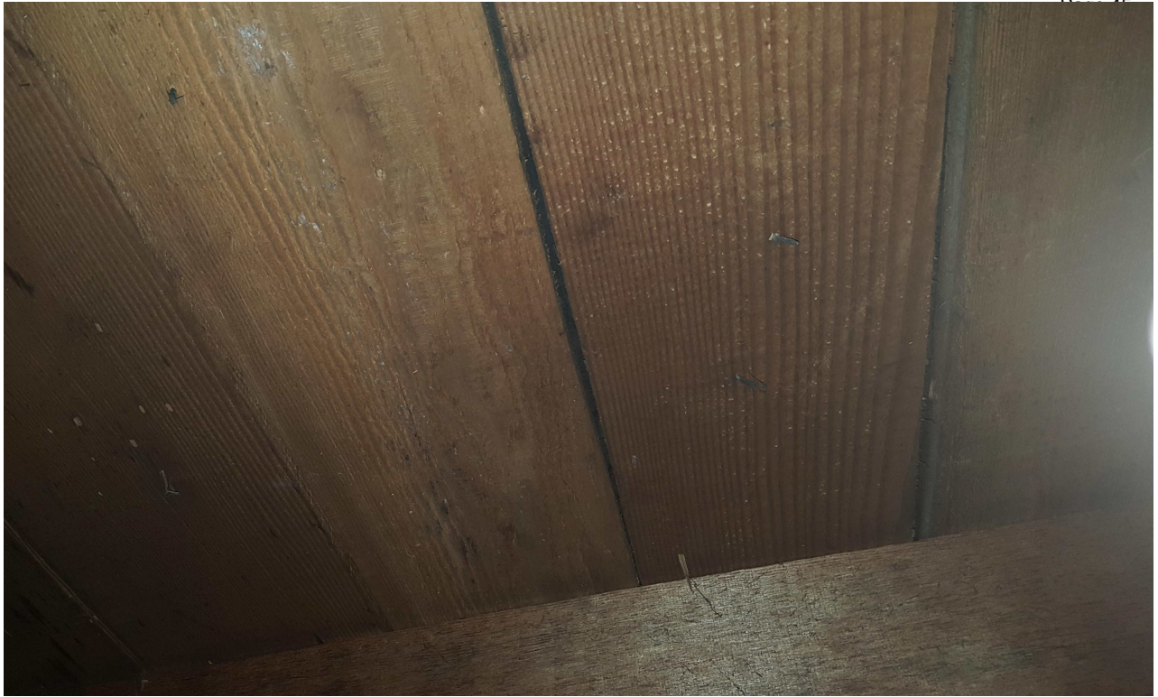
PHOTO - Roof 1" Horizontal Sheathing
