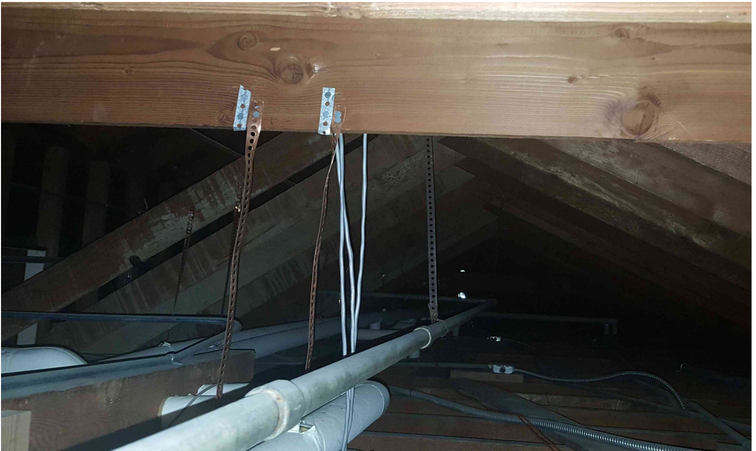
PHOTO - Observed Roof Structure
