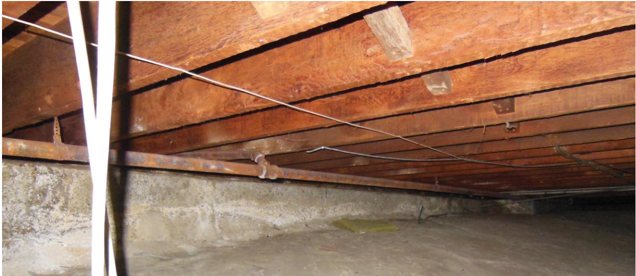
Figure 2 - Crawl Space Prior to Interim Seismic Retrofit
