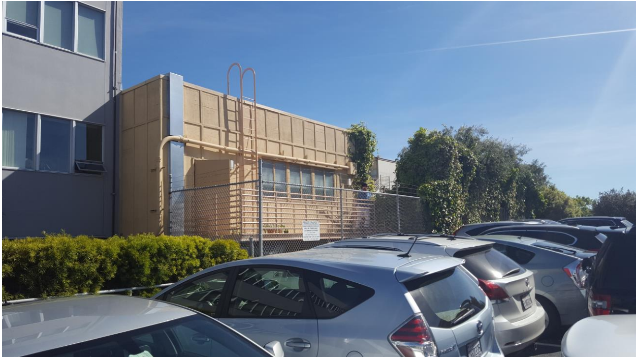
Figure 6 - Building Exterior (South Elevation)
