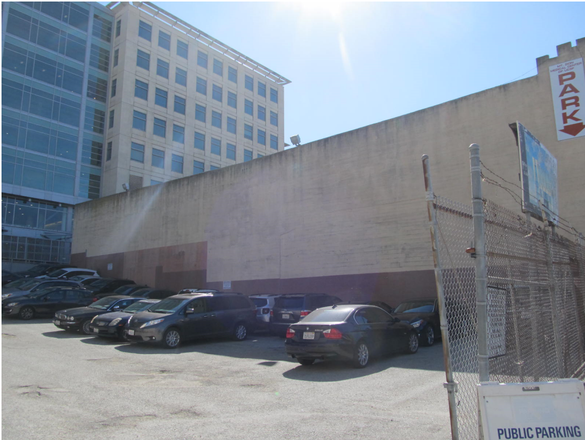
East elevation (looking southwest)
