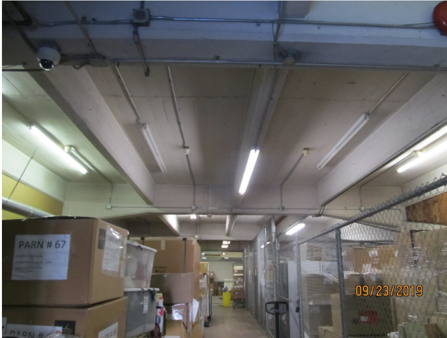
Concrete framing at underside of the second floor (looking south)
