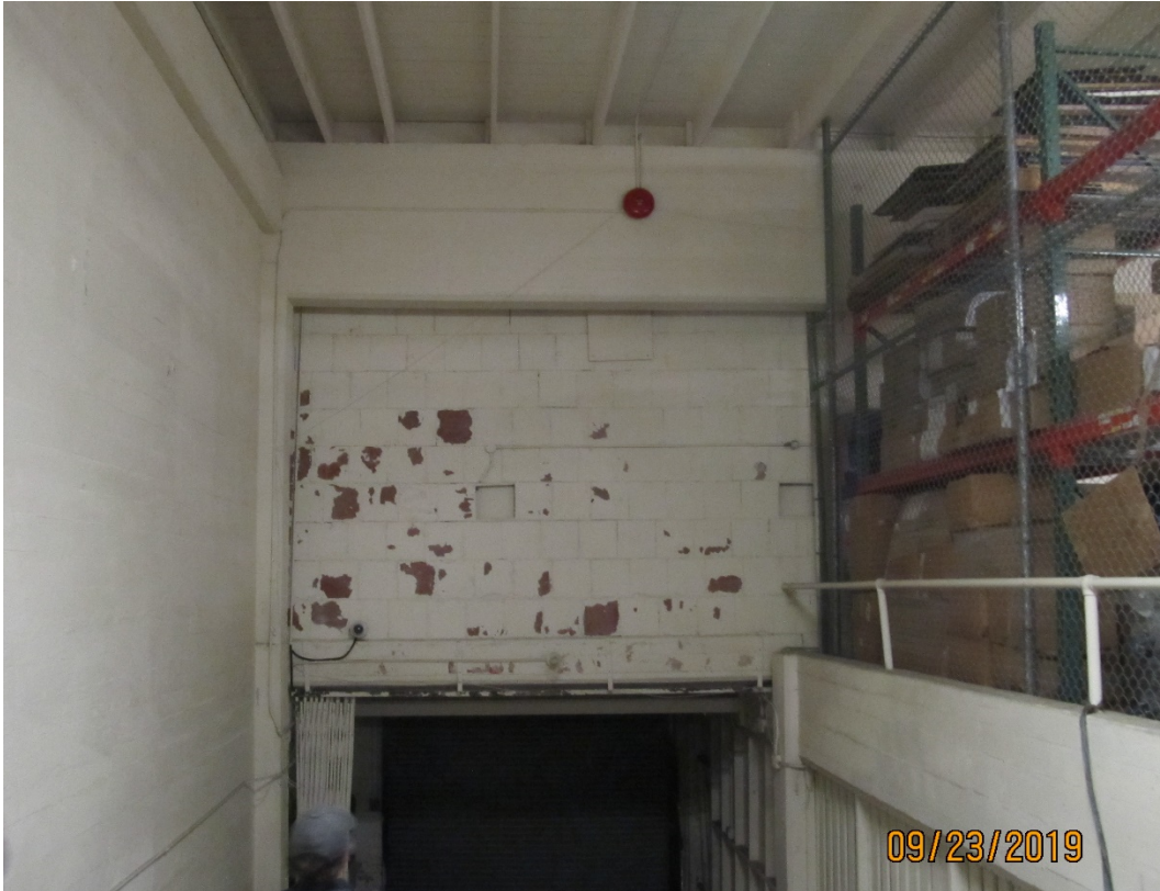
Hollow clay tile partition above ramp (looking north)
