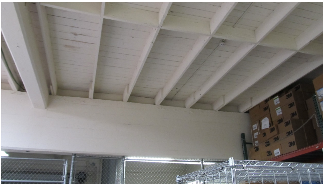
Wood roof framing bearing on concrete girders
