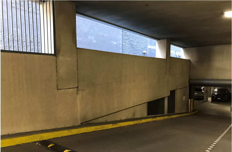
Vehicle ramp to Level B1
