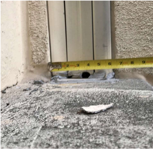
Covered seismic gap at NW corner of building
