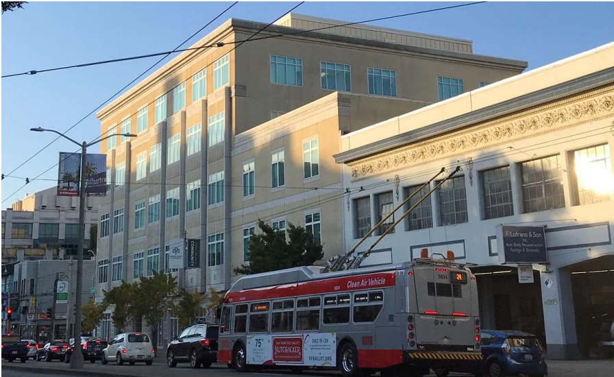
East and north façades
