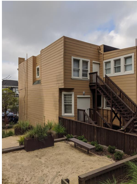
Figure 6 – South Exterior Wall and Rear
