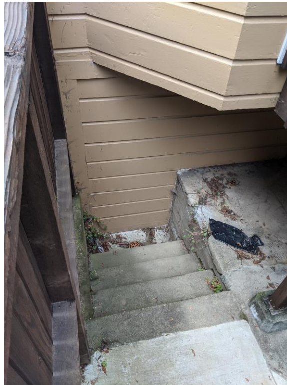
Figure 11 – Infill of Original Rear Basement Egress Door per 1988 Drawings
