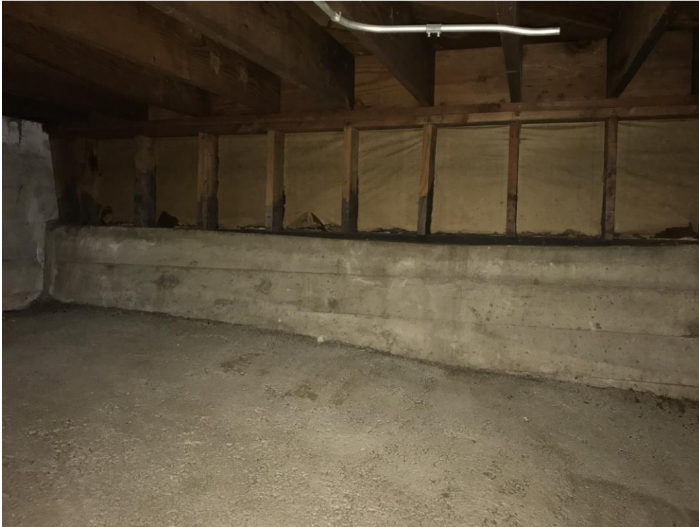
Figure 12 – Southeast Corner of Crawlspace
