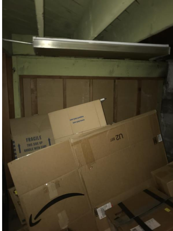
Figure 13 – North Partition Wall of Crawlspace with Diagonal Sheathing Visible
