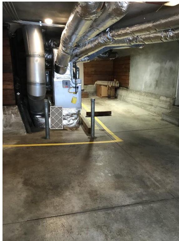
Figure 5 – Garage Interior, Looking East
