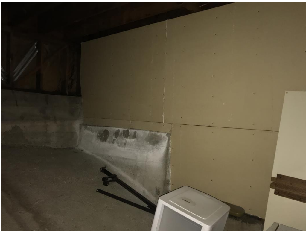
Figure 15 – Southwest Corner of Crawlspace
