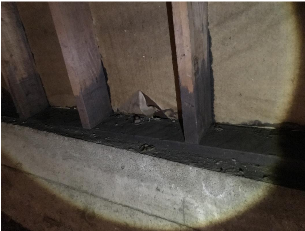
Figure 13 – Existing Mudsill Anchor at Crawlspace Cripple Wall
