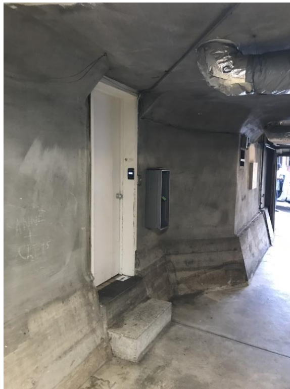
Figure 7 – Garage Wall Opposite Entry and Interior Stairwell
