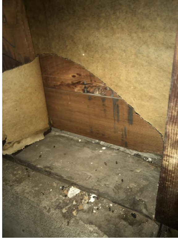
Figure 14 – Straight Sheathing at South Cripple Wall
