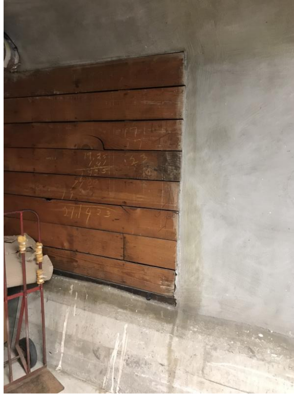
Figure 6 – Southeast Corner of Utility Space with Stucco and Straight Sheathing
