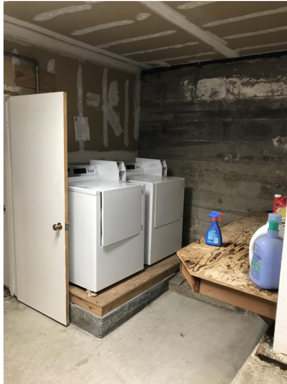
Figure 10 – Laundry Room Looking Northeast
