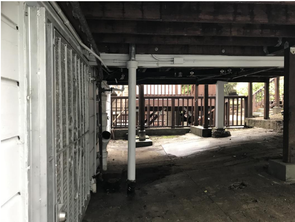
Figure 8 – Underside of Deck and Rear Addition
