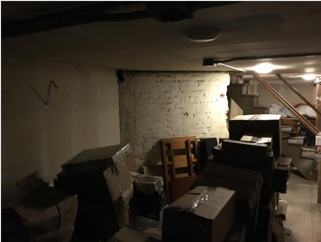
Figure 7 – Masonry Wall Under Living Room Fireplace Above
