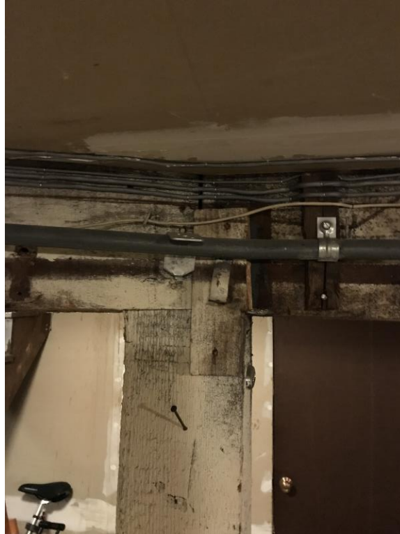
Figure 10 – Top of Basement Post
