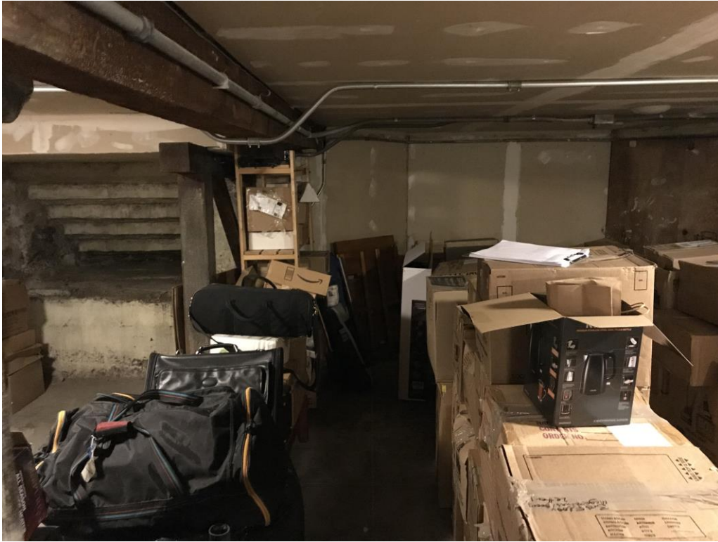
Figure 5 – West (Front) Basement Wall
