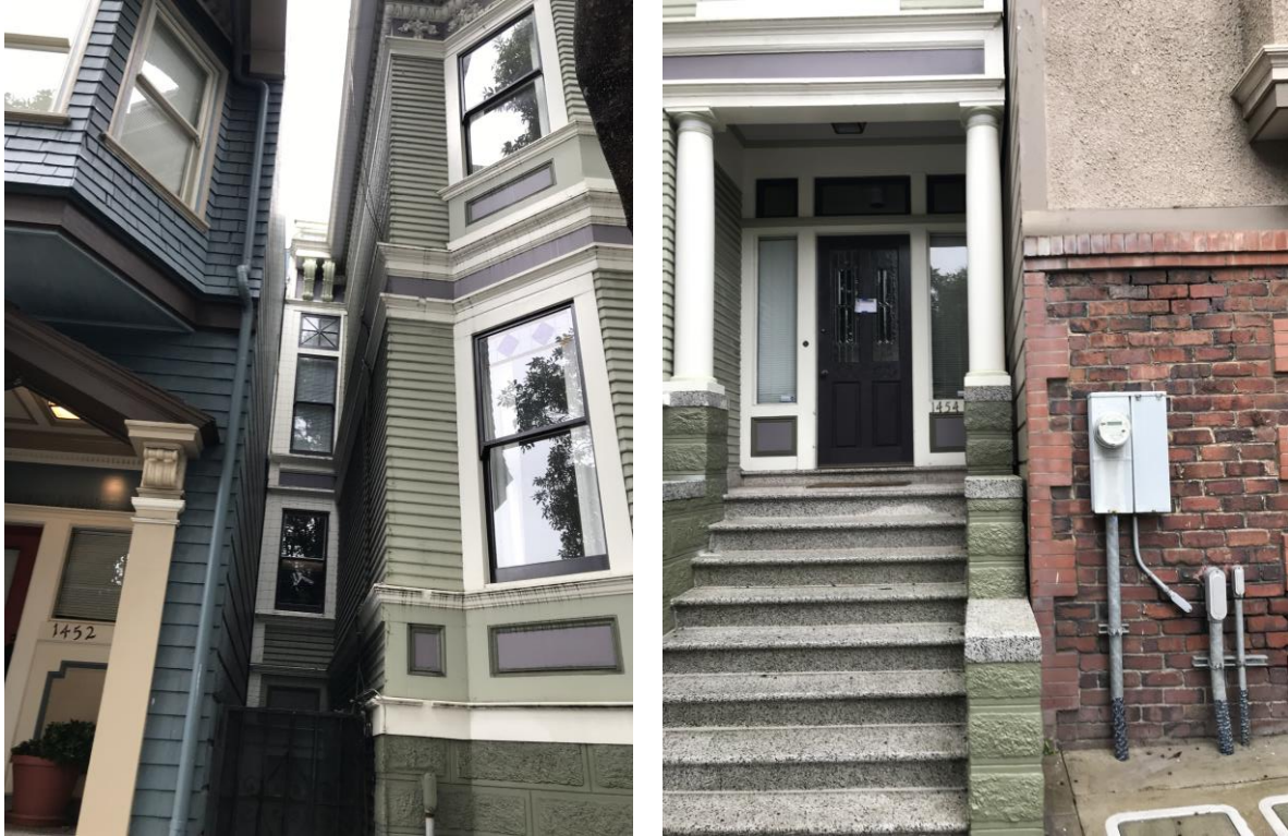
Figure 4 - Building Separation to the North (Left) and South (Right)
