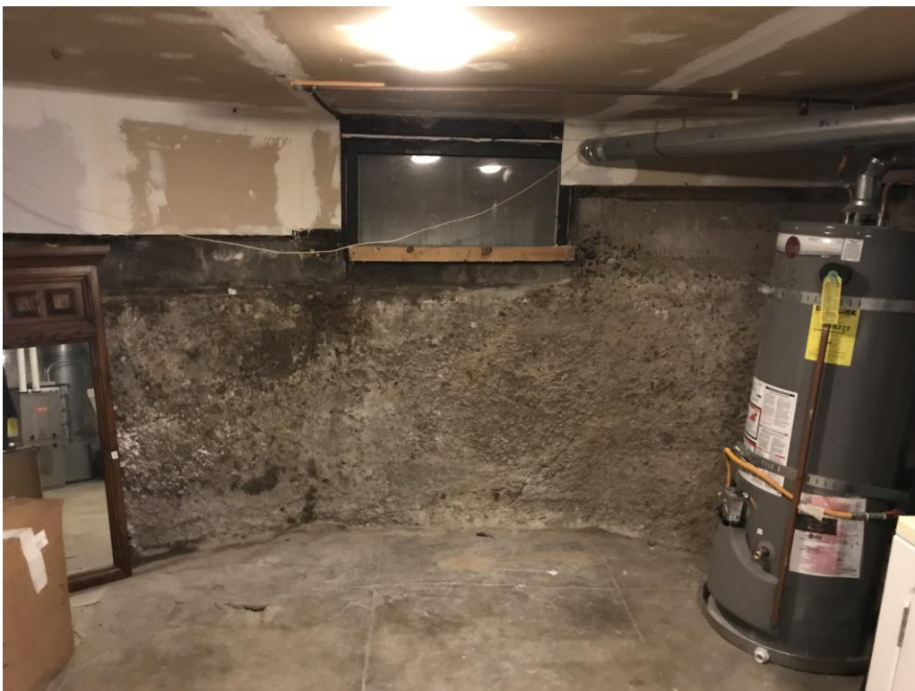
Figure 8 – East (Rear) Basement Wall
