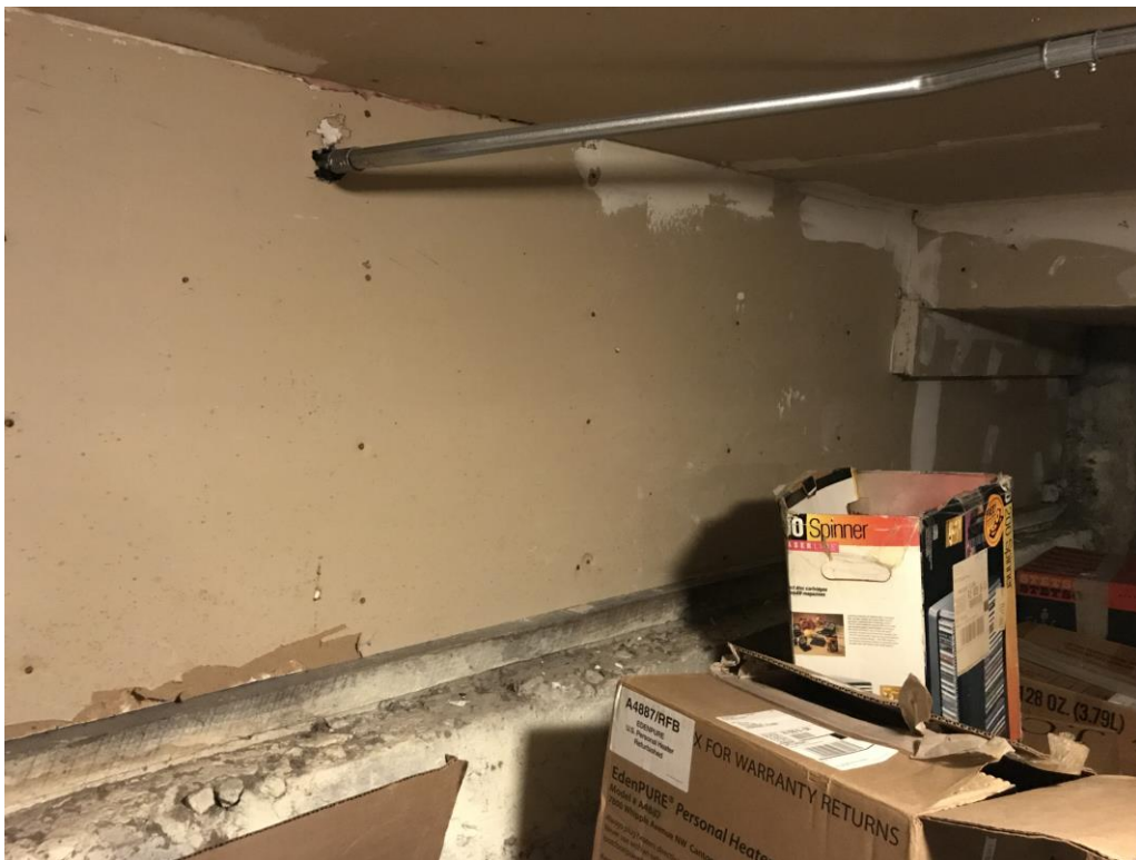
Figure 6 – South Basement Wall
