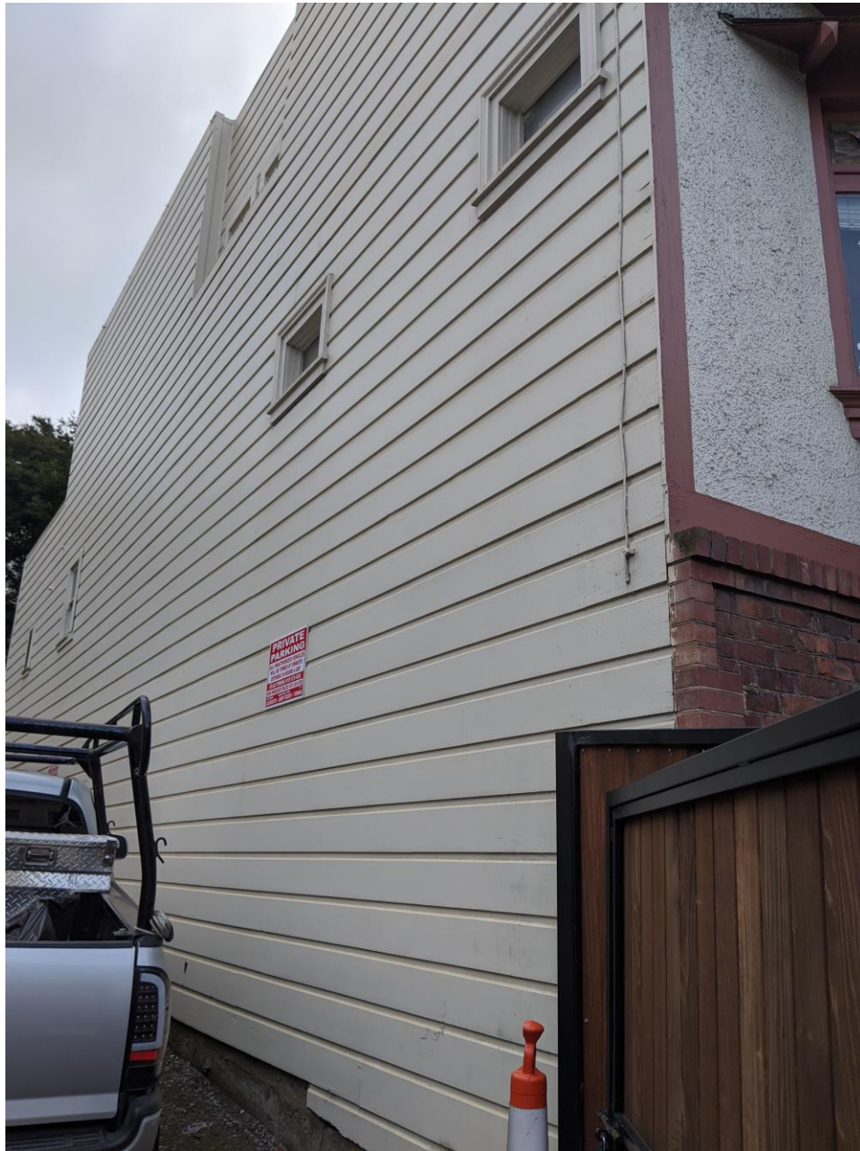
Figure 6 – North Exterior Wall
