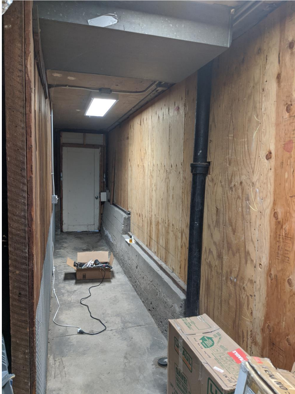
Figure 11 – New Sheathing at South Exterior Wall
