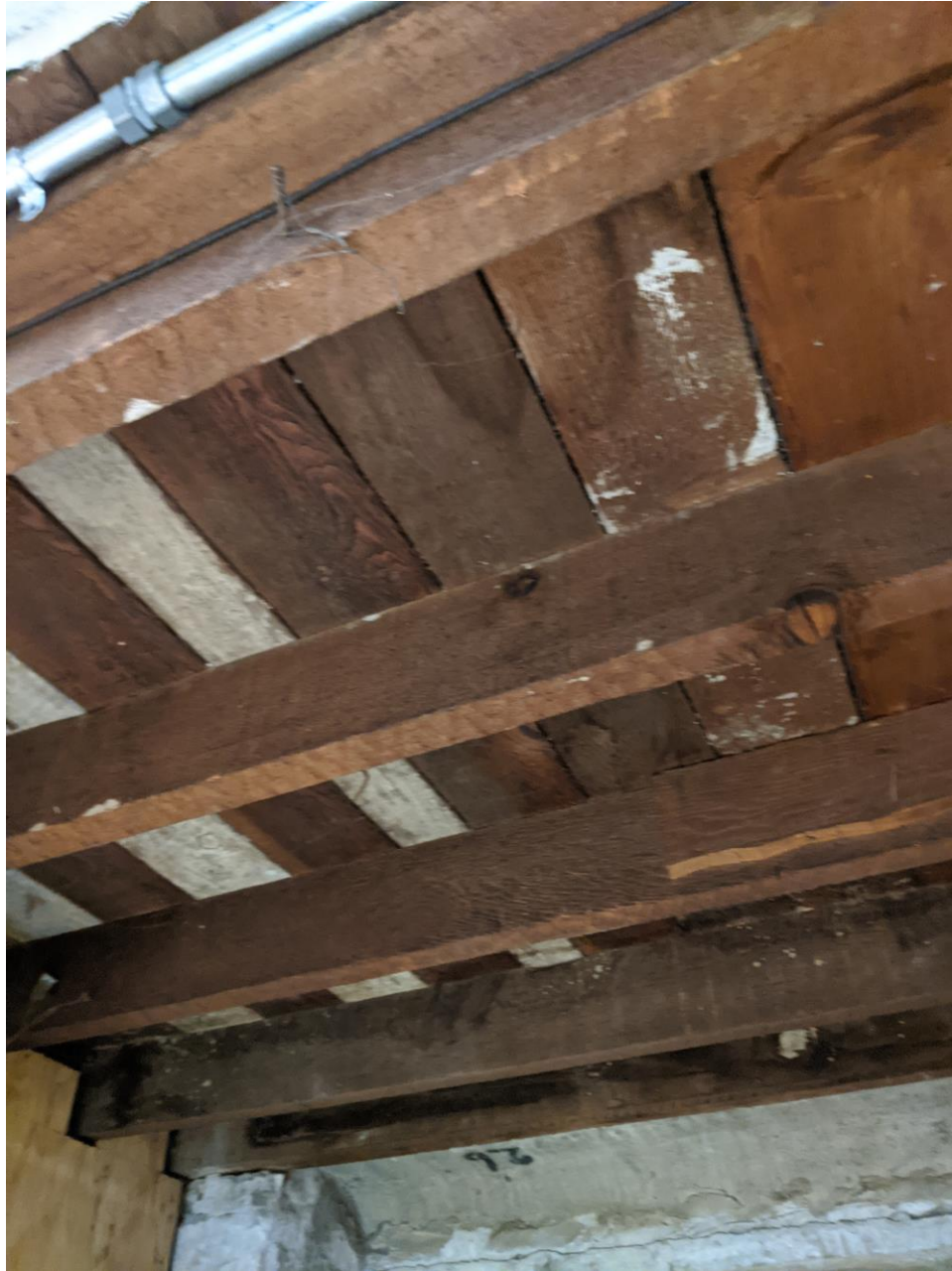
Figure 12 – First Floor Straight Sheathing
