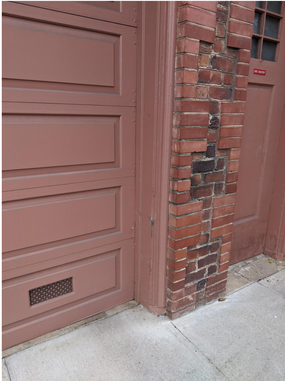
Figure 7 – West (Front) Wall Pier Between Garage Doors
