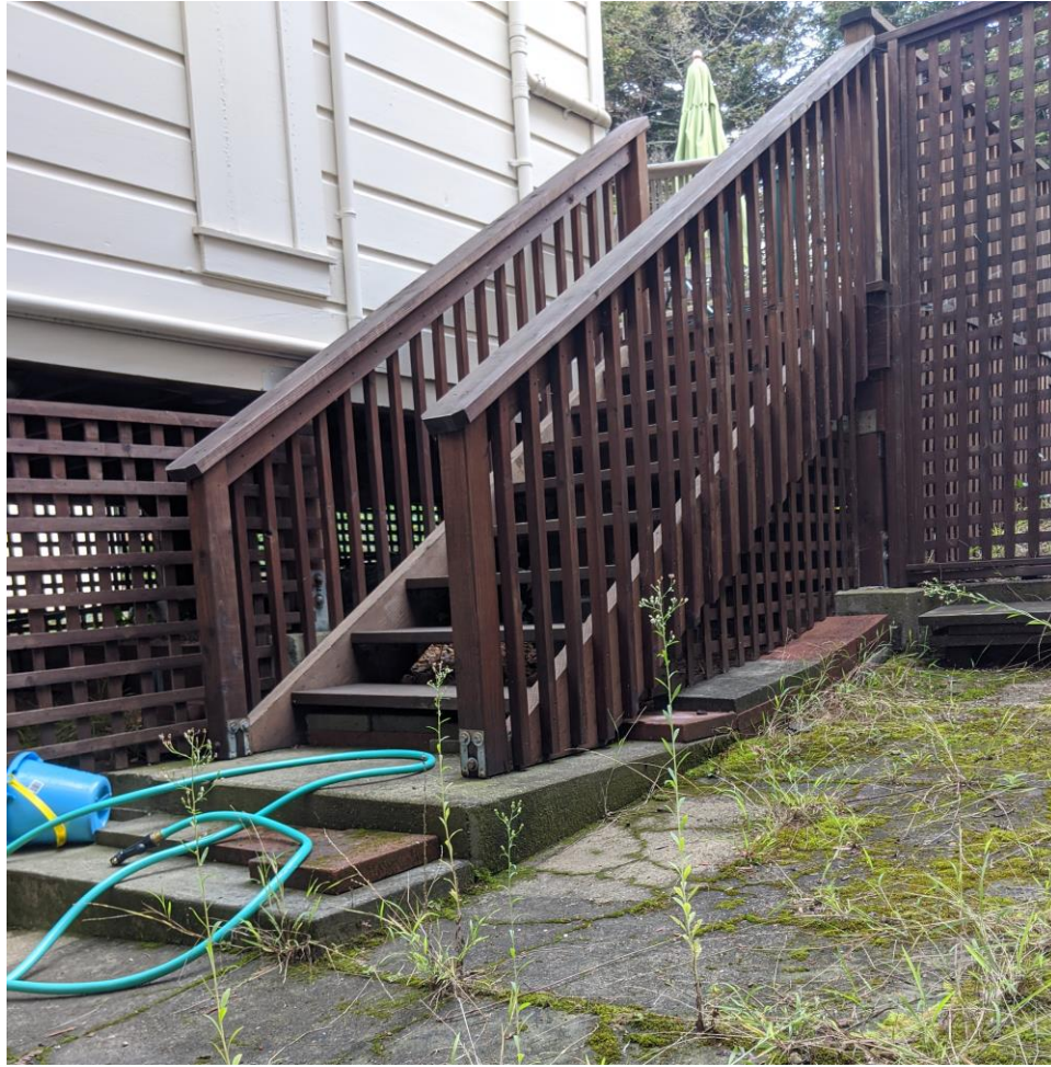
Figure 15 – Deck Stairs Adjacent to Elevated Porch
