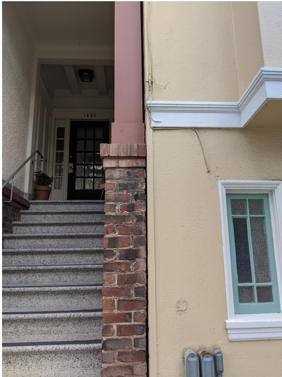
Figure 5 - Building Separation to the South (1420 is Left)
