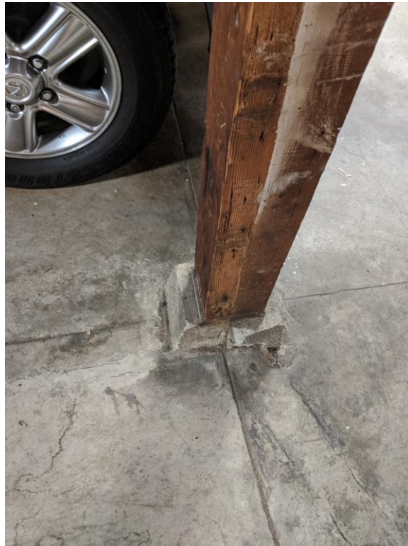
Figure 13 – Top and Bottom of Interior Post
