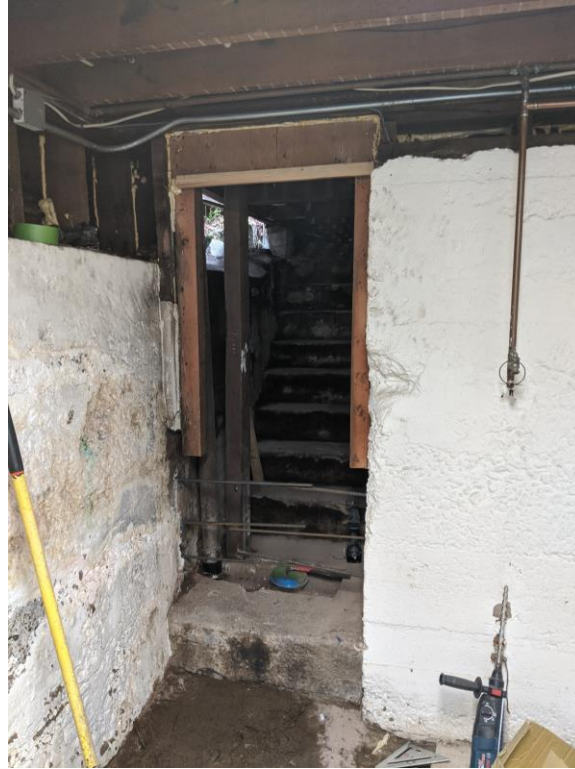
Figure 12 – Work in Progress at Former East Egress Door
