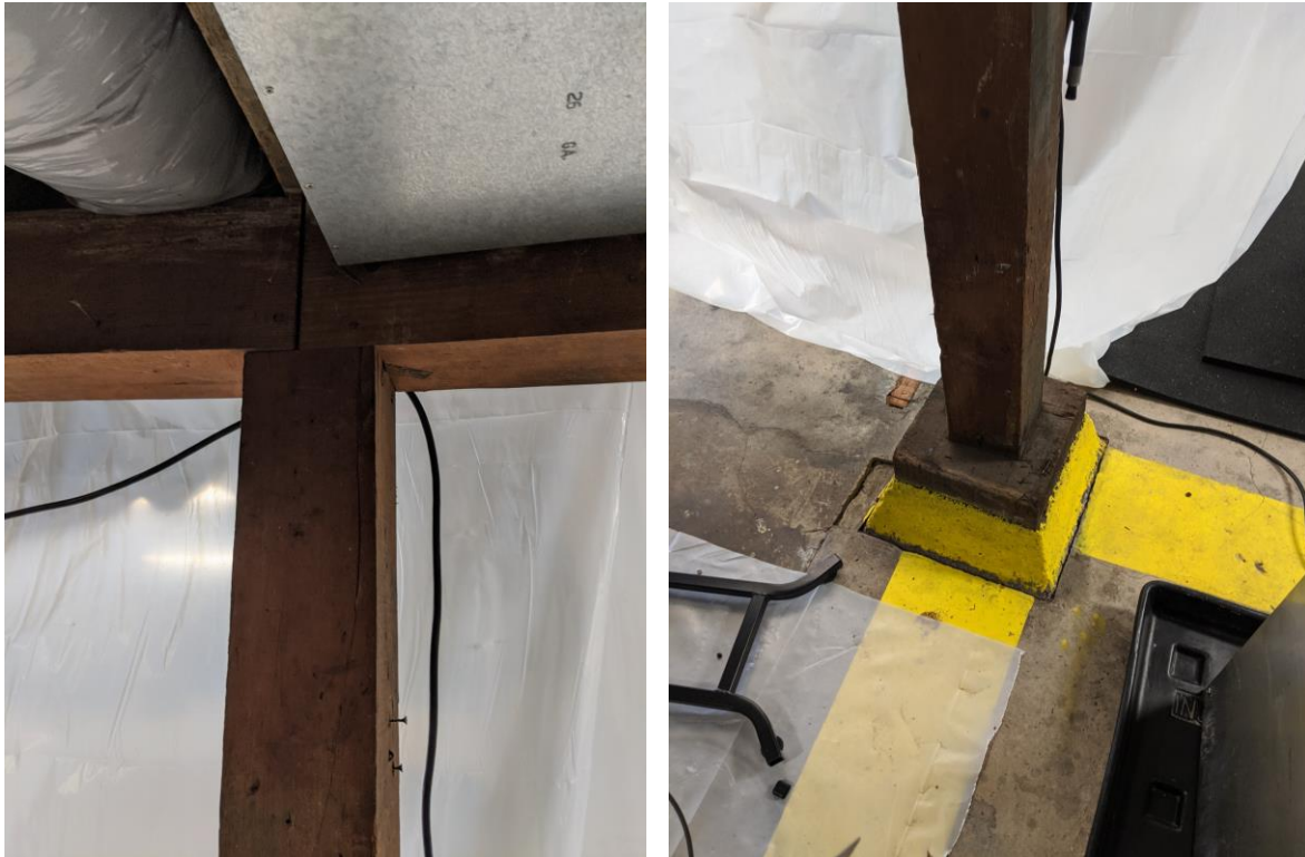
Figure 10 – Interior Basement Post without Connections
