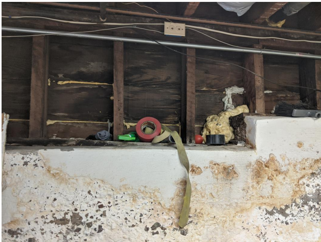
Figure 11 – North Cripple Wall with Straight Sheathing
