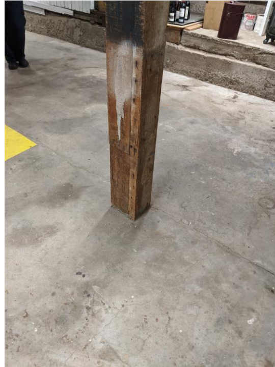
Figure 10 – Interior Basement Post on Blocking with 2x Splint
