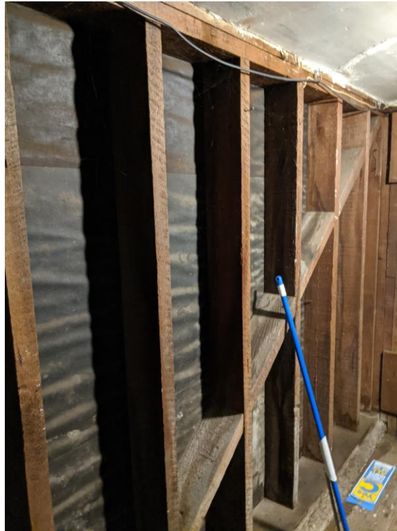
Figure 13 – Let-In Bracing at Basement Exterior Wall
