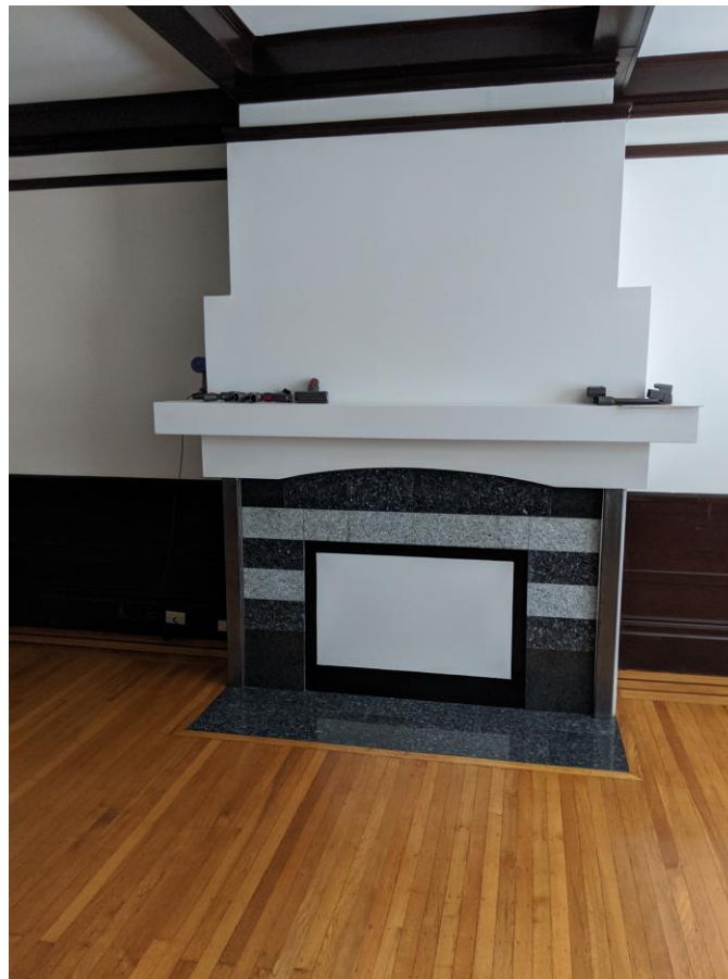
Figure 7 – Closed Off Fireplace at First Floor
