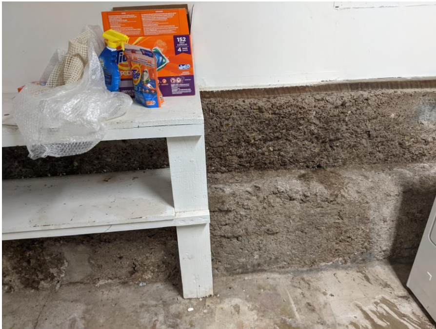
Figure 8 – Foundation Benching Along East Exterior Wall
