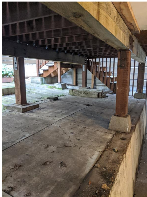
Figure 16 – Support of Rear Deck
