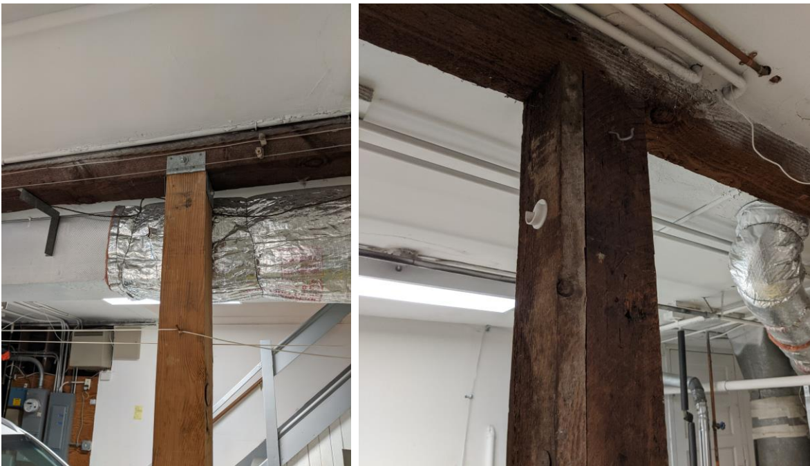
Figure 11 – Top of Interior Basement Posts
