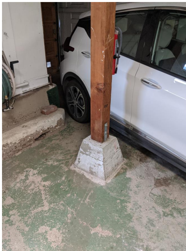
Figure 9 – Interior Basement Post on New Concrete Pedestal
