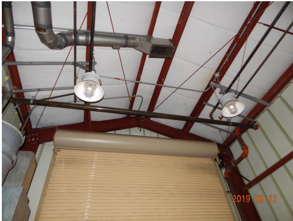
Photo 2. Moment Frame and Roof Framing.
