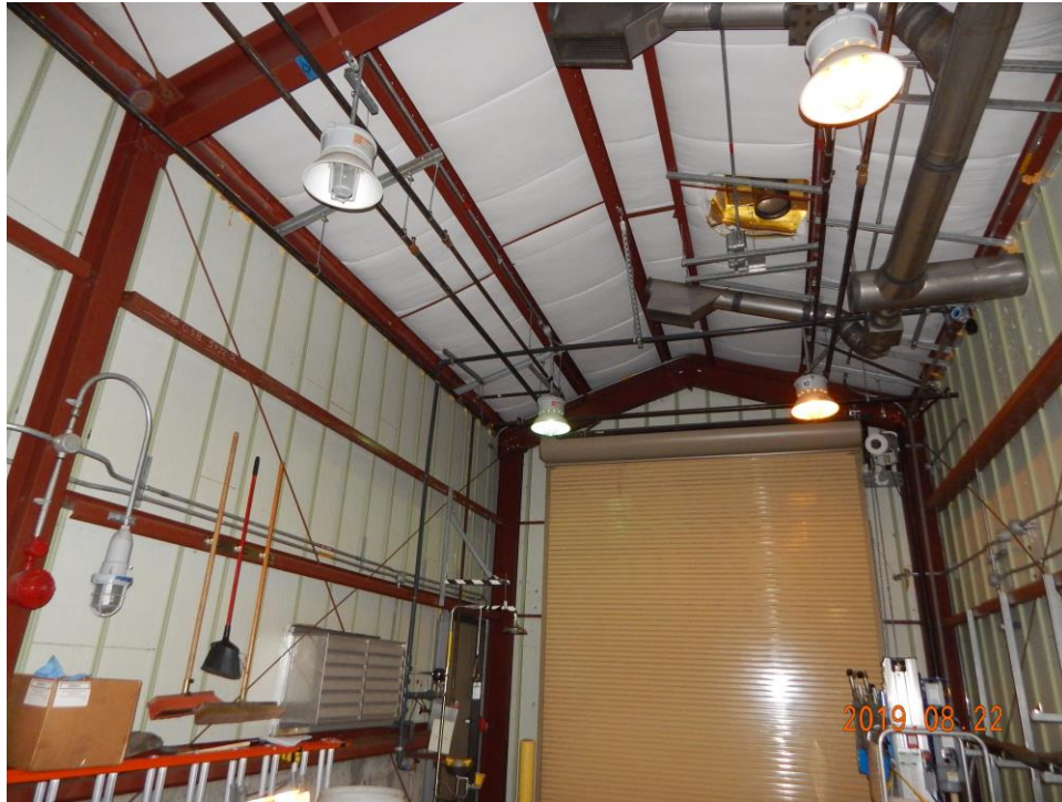
Photo 5. Interior showing rod bracing and moment connection.
