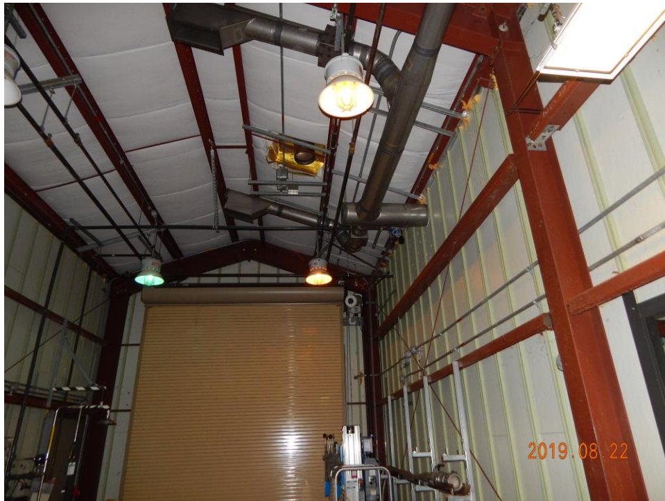
Photo 4. Interior showing rod bracing.
