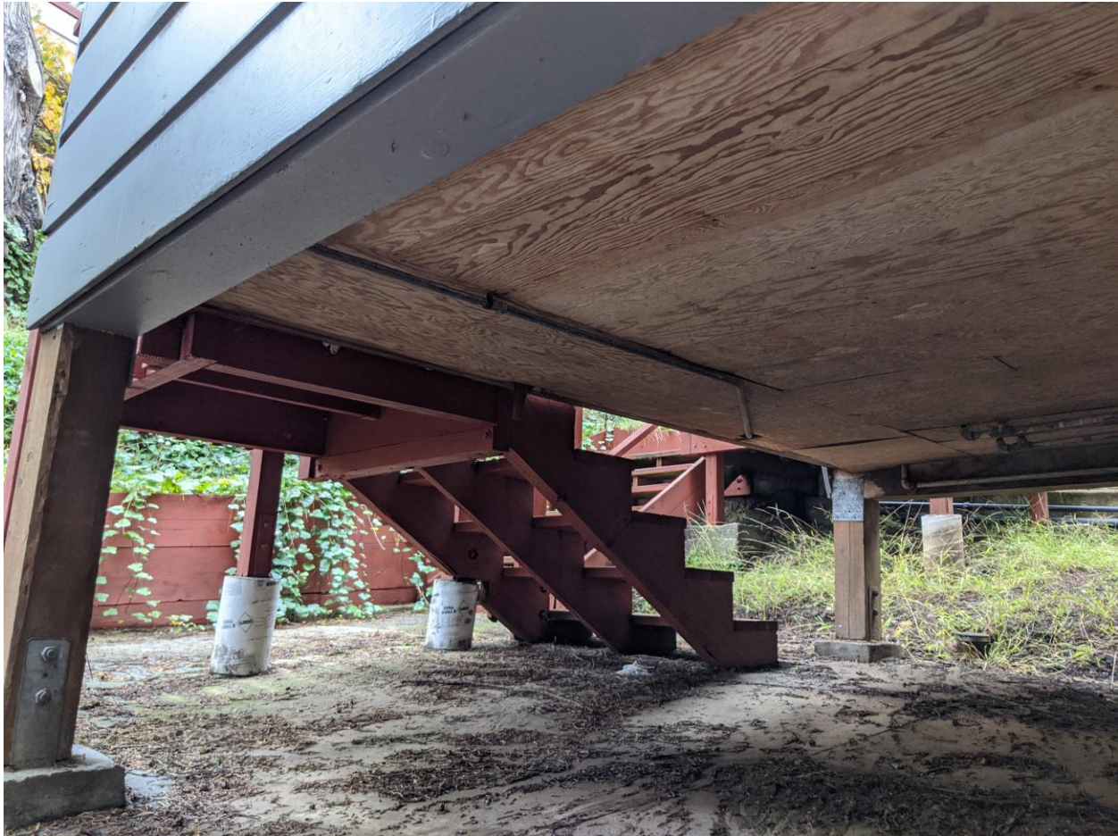
Figure 10 – Underside of First Floor Dining Room
