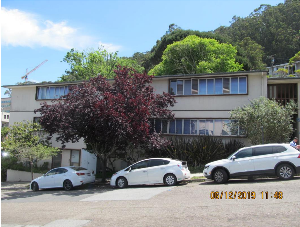
West elevation (looking northeast)
