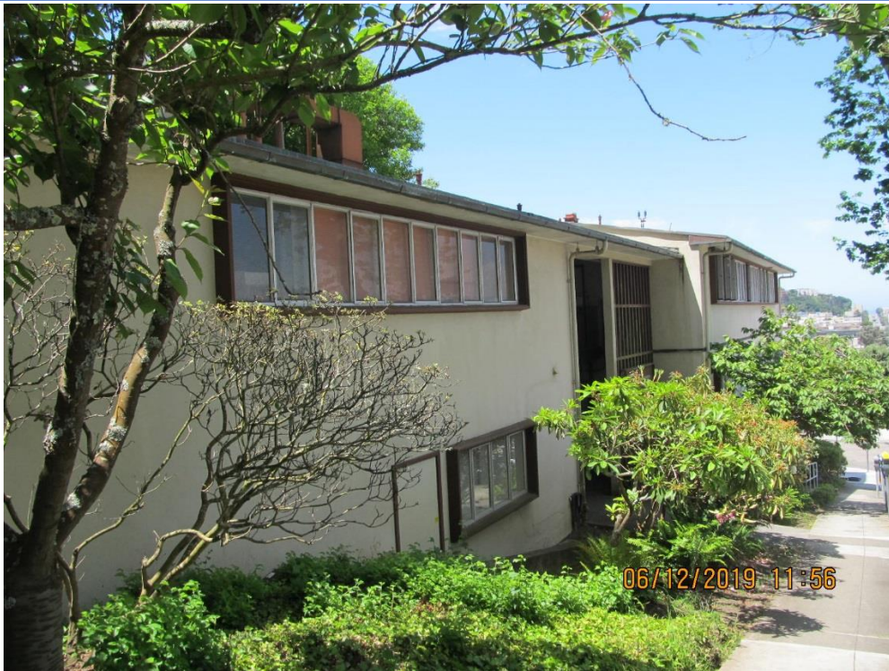
North elevation of lab 1964 addition (looking southwest)
