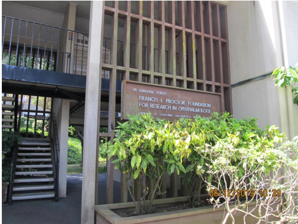
North elevation of stair between original 1954 structure and the 1964 lab addition (looking southwest)
