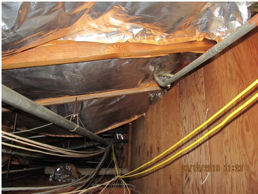
Interior shear wall at underside of roof
