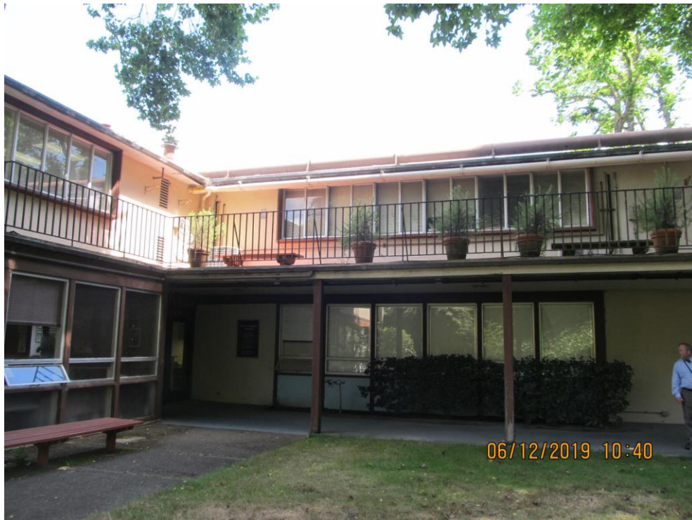
South elevation of east wing (looking northwest)
