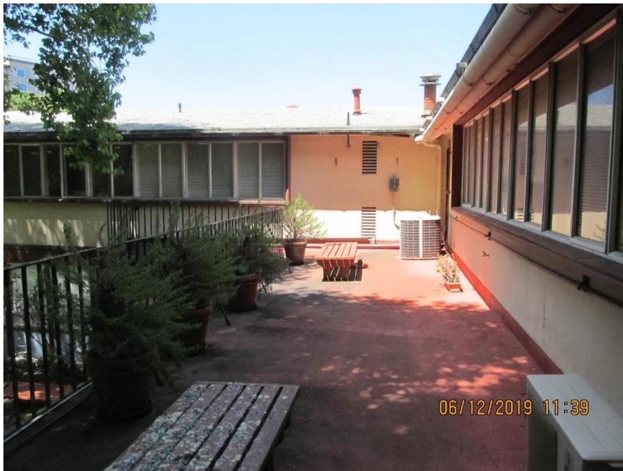
Terrace on the south elevation
