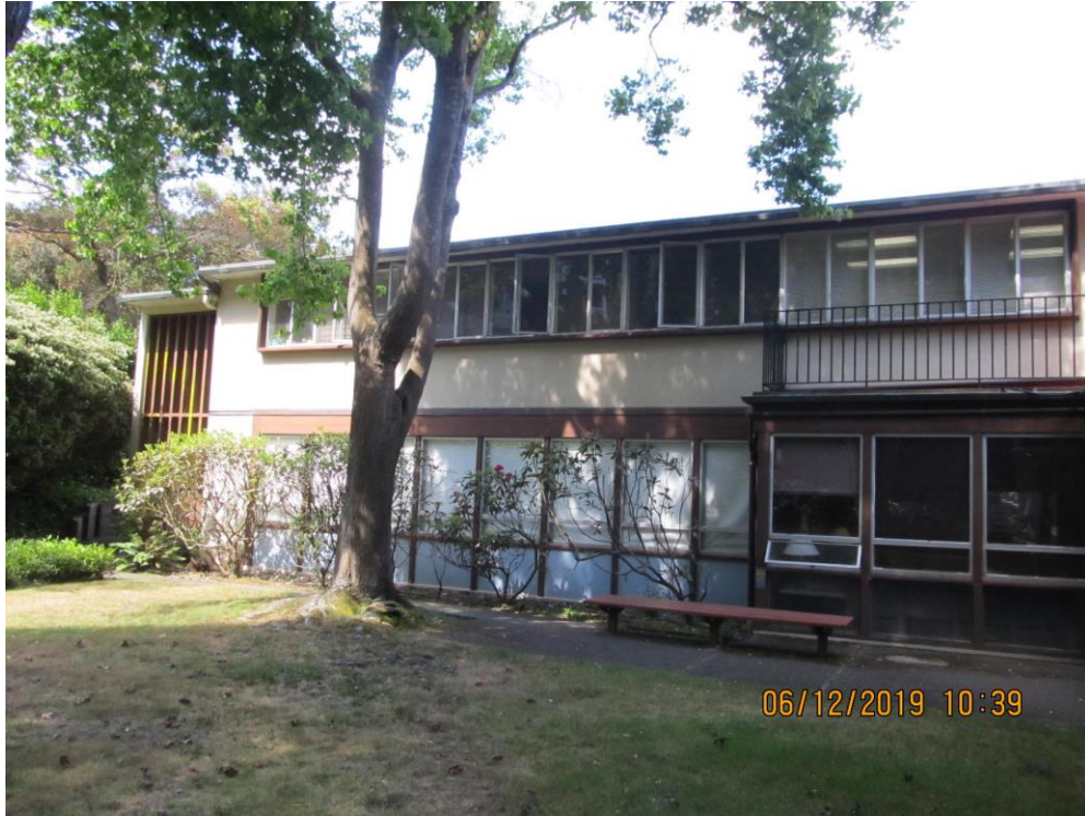
East elevation of west wing (looking southwest)
