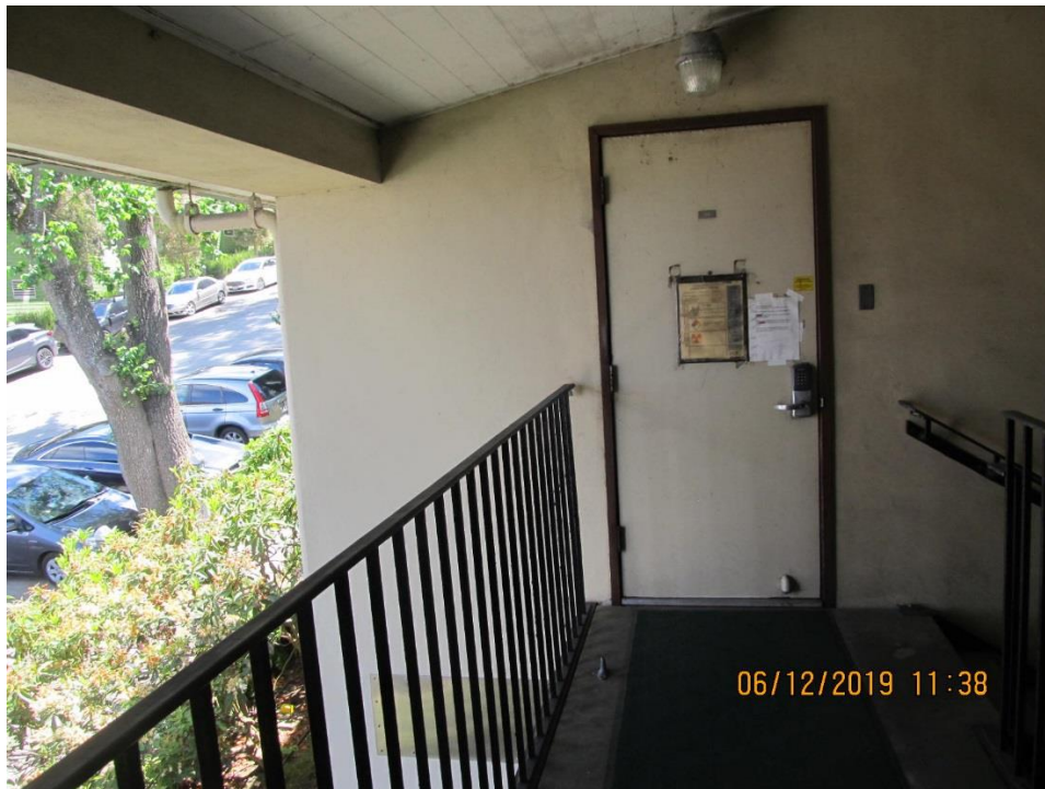
Stair between original 1954 structure and 1964 lab addition (looking east at west elevation of the addition)
