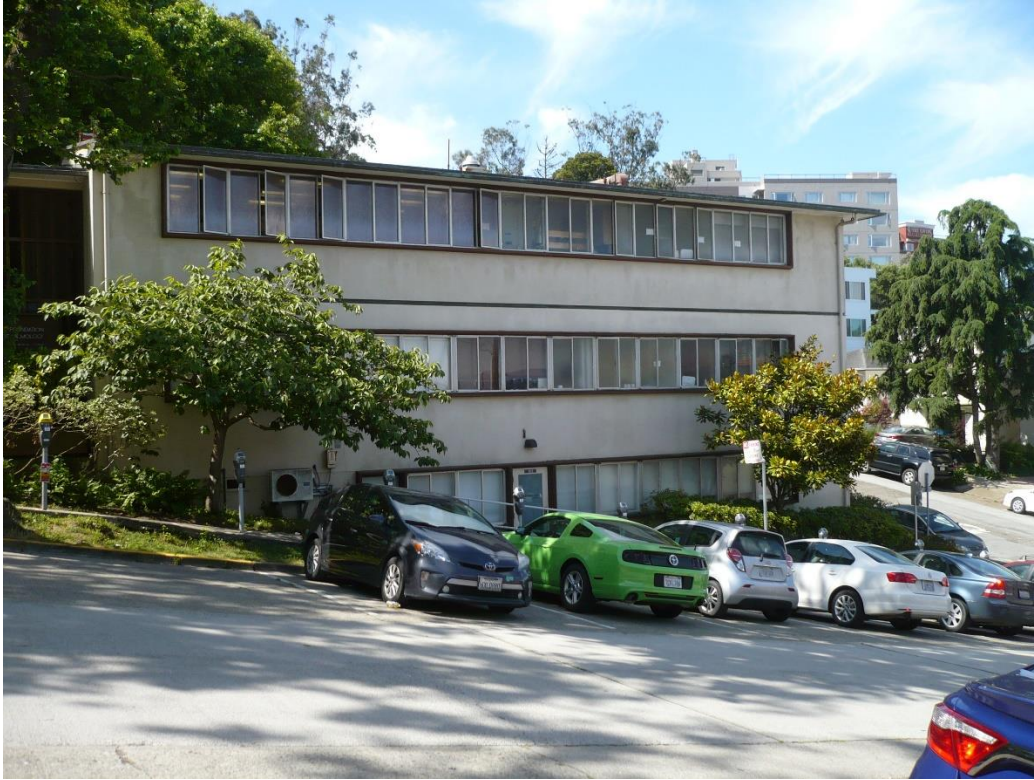
North elevation (looking southwest)
