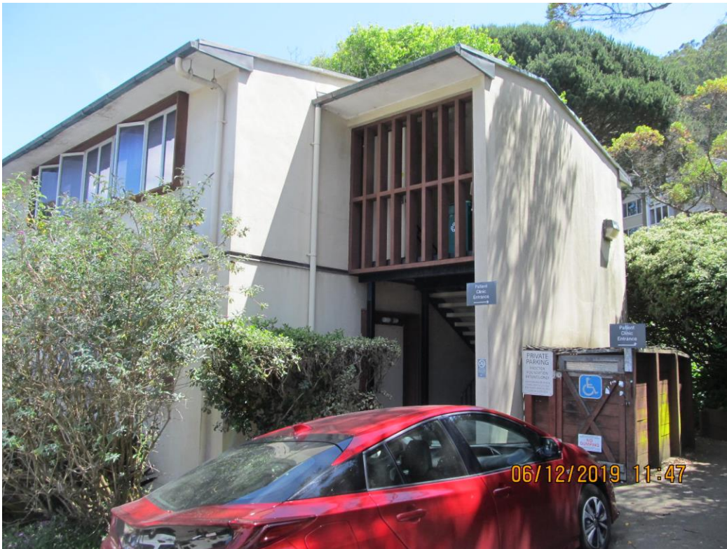
Exterior stair on south elevation (looking northeast)
