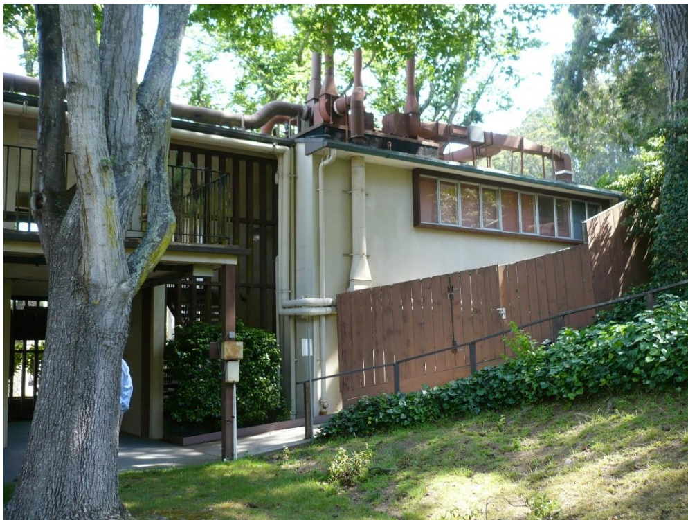
South elevation of 1964 lab addition (looking northwest)
