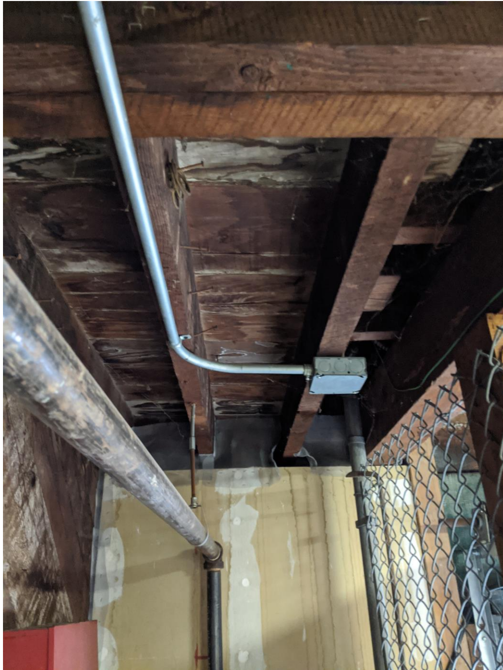
Figure 12 – First Floor Sheathing and Framing
