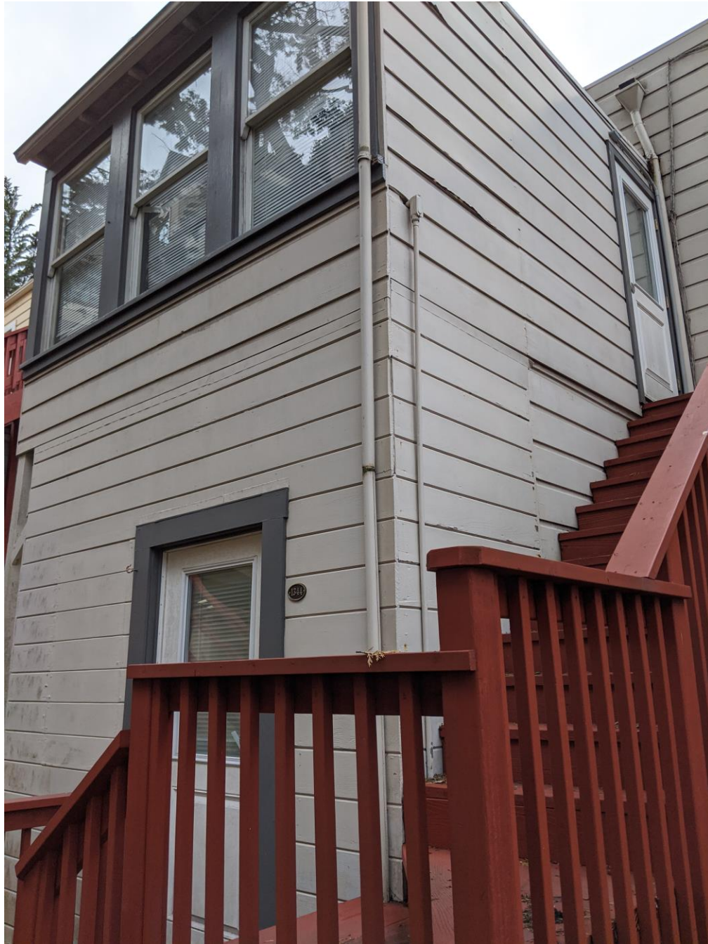
Figure 13 – Rear Bedroom (Second Floor), Bathroom (First Floor), and Stair
