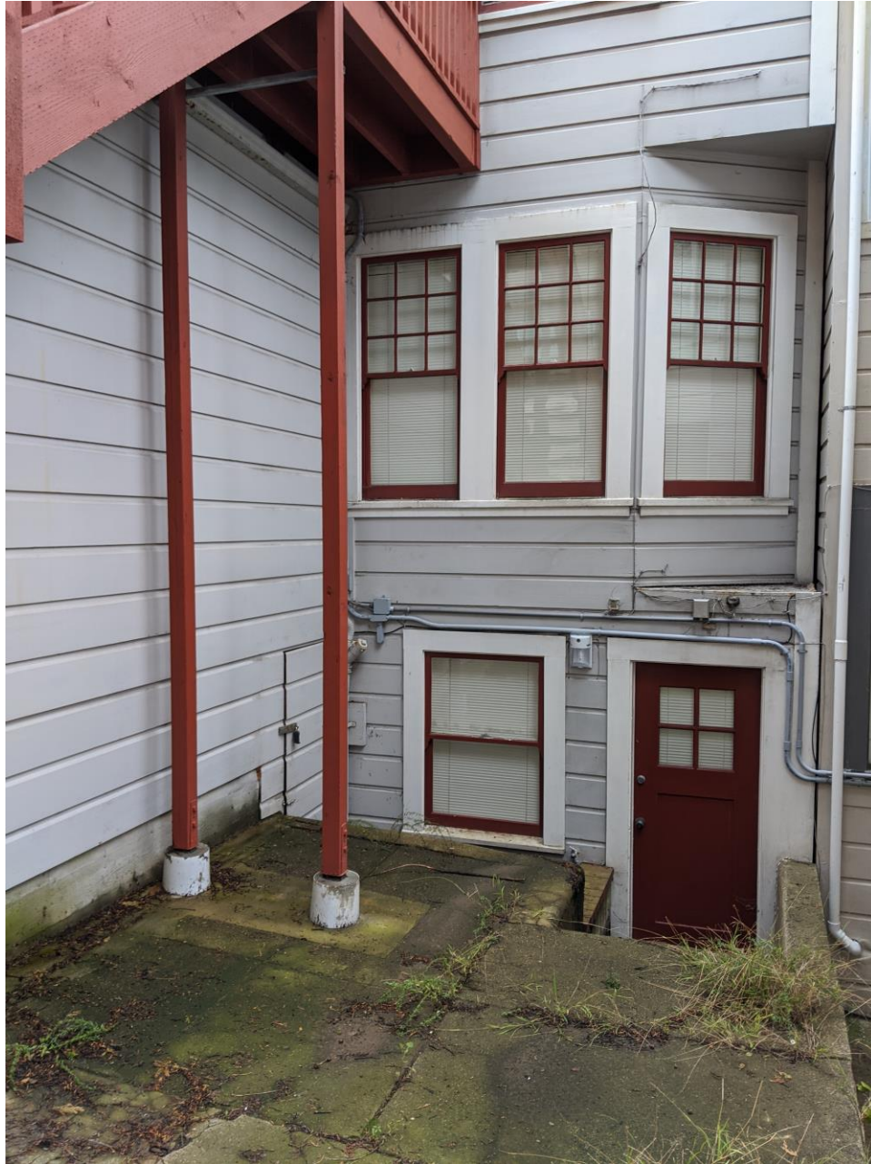
Figure 11 – Rear Ground Floor Door and Exterior Stairs
