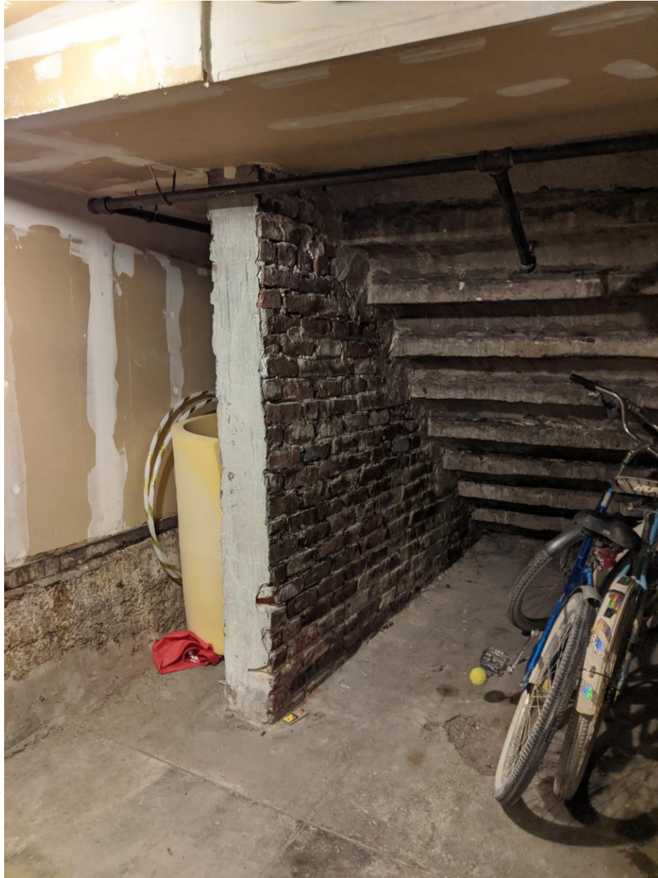
Figure 10 – Area Under Upper Unit Entrance Stairs
