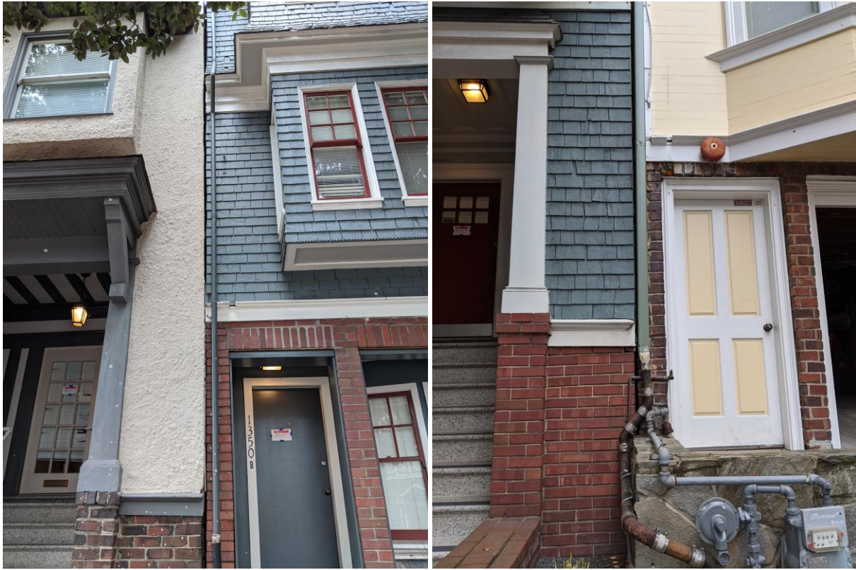
Figure 5 - Building Separation to the North (Left) and South (Right)
