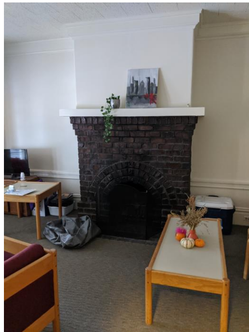
Figure 6 – Closed Off Existing Fireplace
