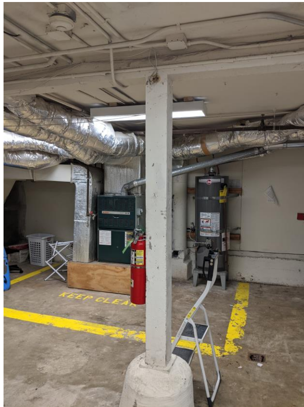
Figure 10 – Basement Post and Beam without Connector Hardware
