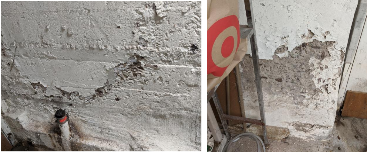
Figure 9 – Concrete Condition in Basement
