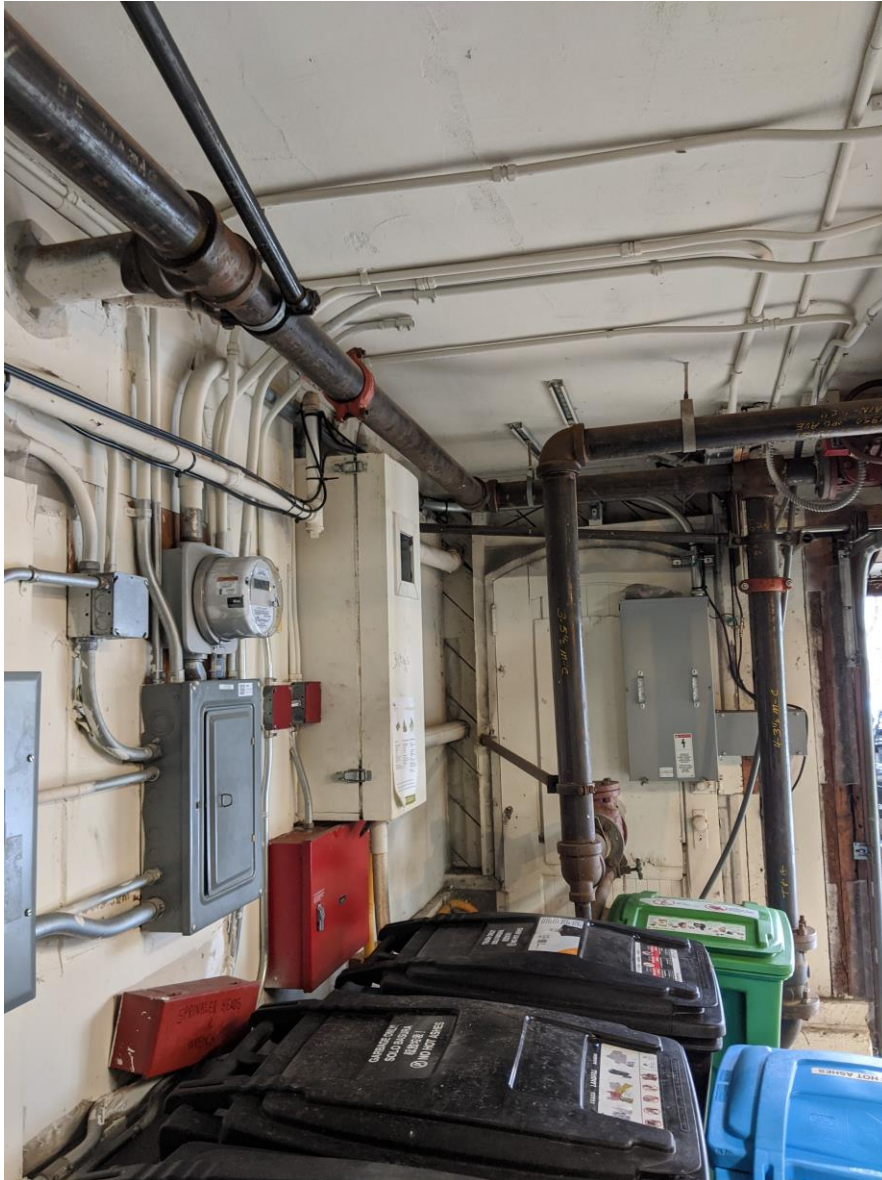
Figure 6 -Diagonal Sheathing at West (Front) Wall
