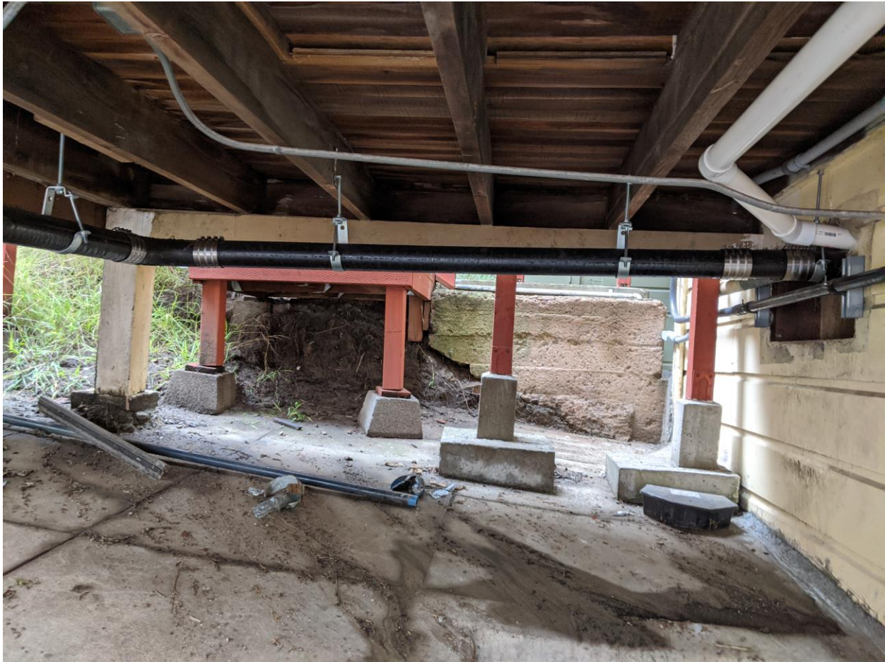
Figure 10 – Underside of Rear Hall
