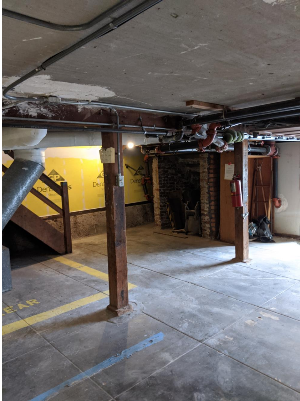
Figure 8 – Post and Beams in Basement
