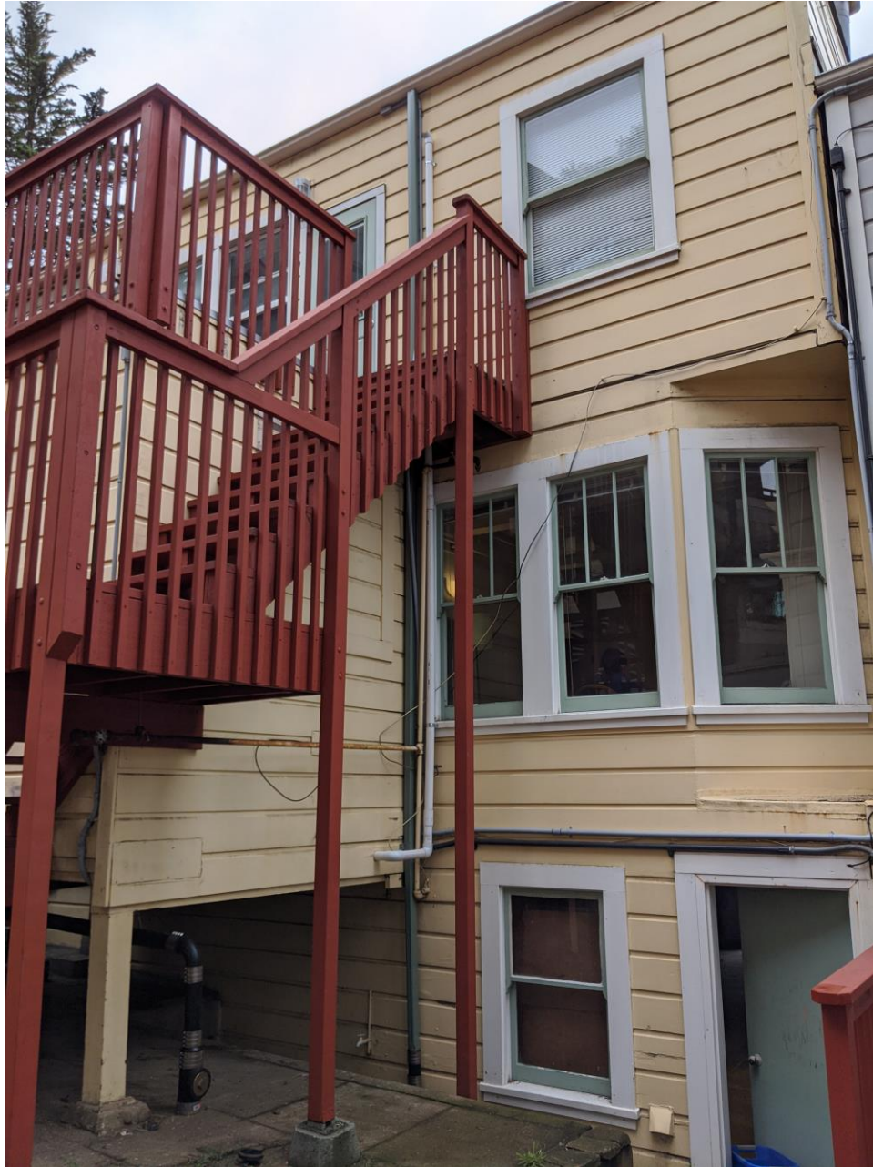
Figure 9 – Building Rear and Stairs
