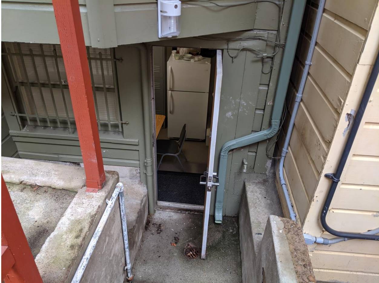
Figure 10 – Basement Rear Egress and Retaining Walls
