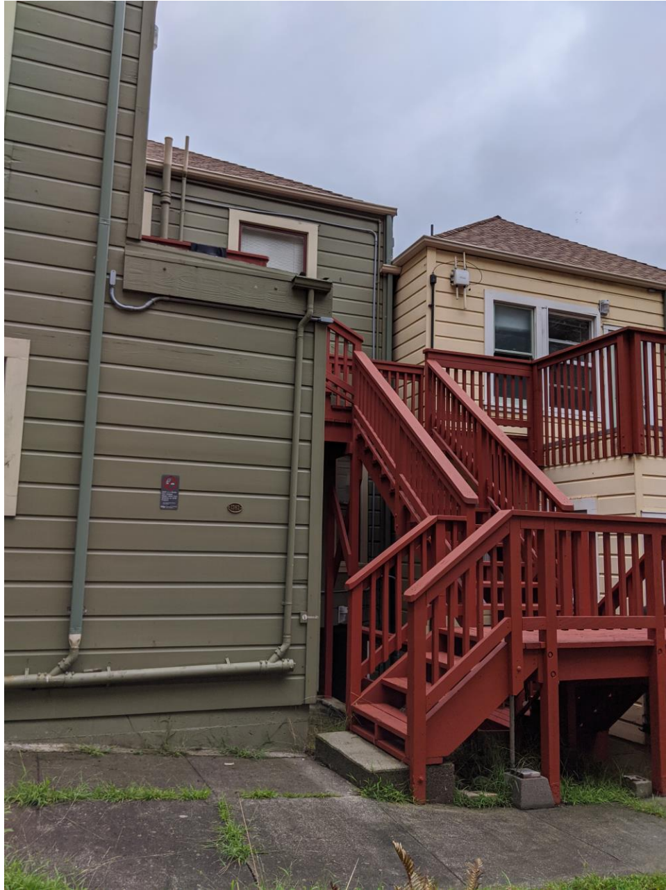
Figure 11- Rear of Building and Exterior Stair
