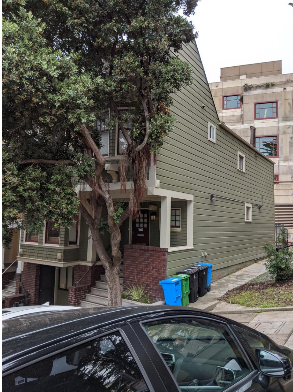
Figure 6 – South Exterior Wall
