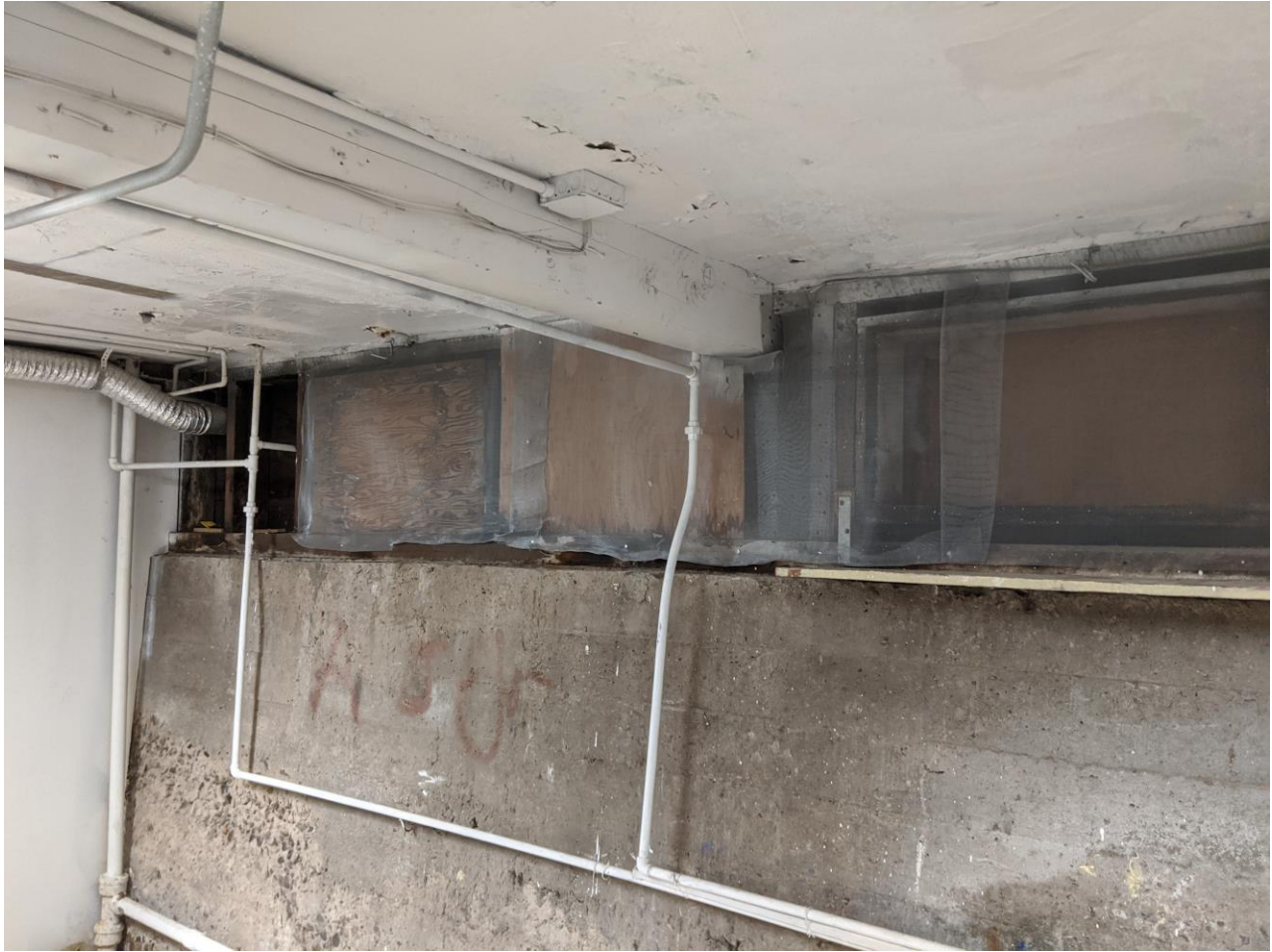
Figure 9 – Sheathing at Rear (East) Cripple Wall
