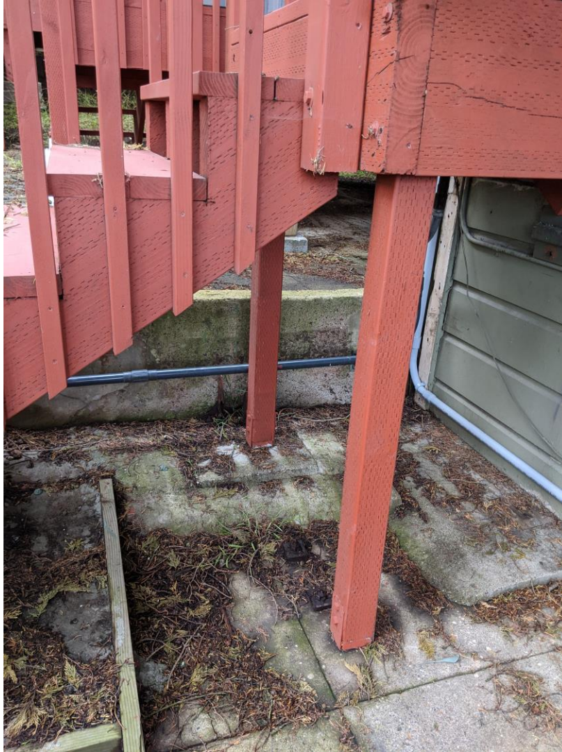
Figure 12 – Rear Exterior Stairs
