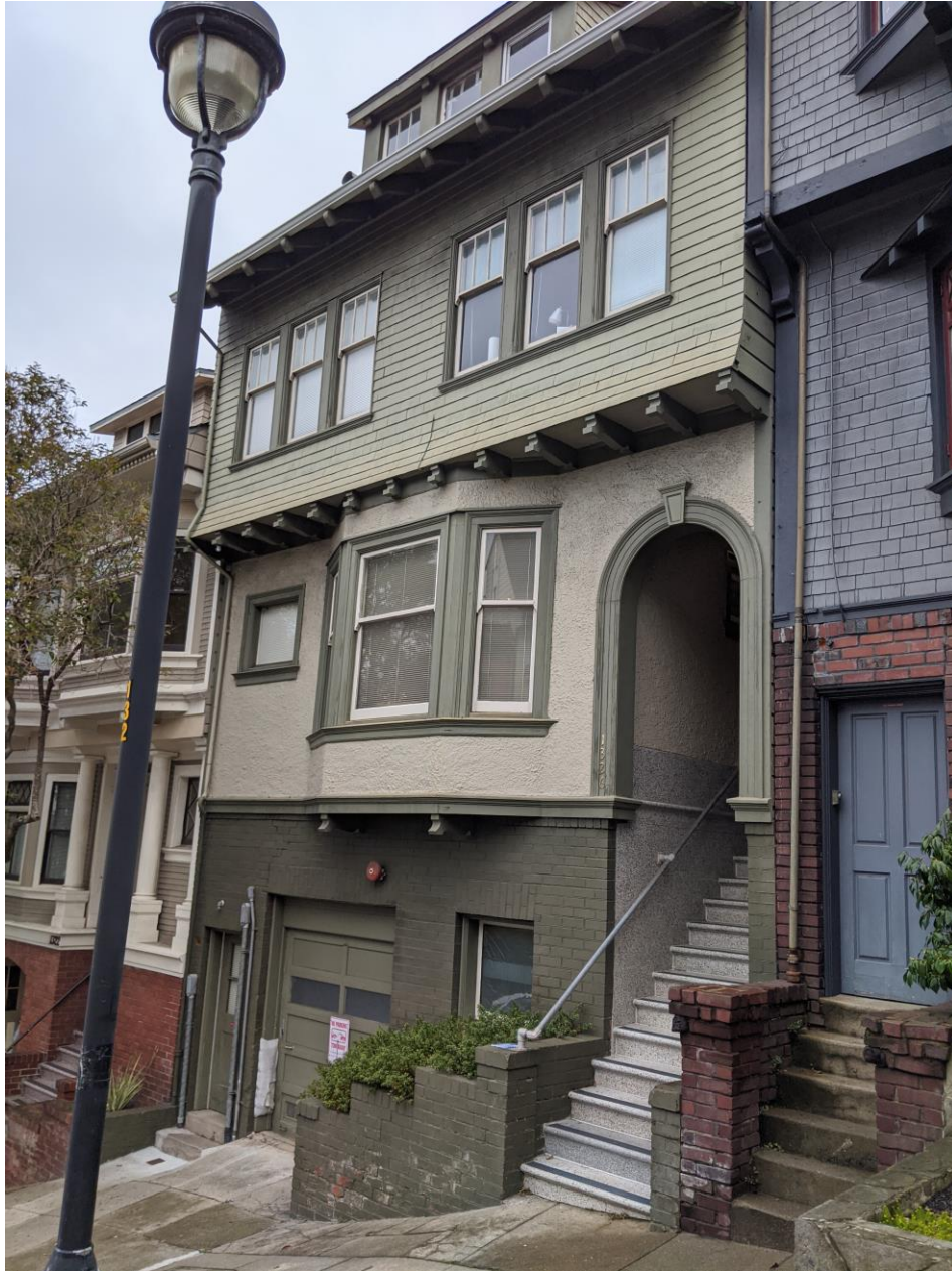
Figure 5 – Front (West) of Building
