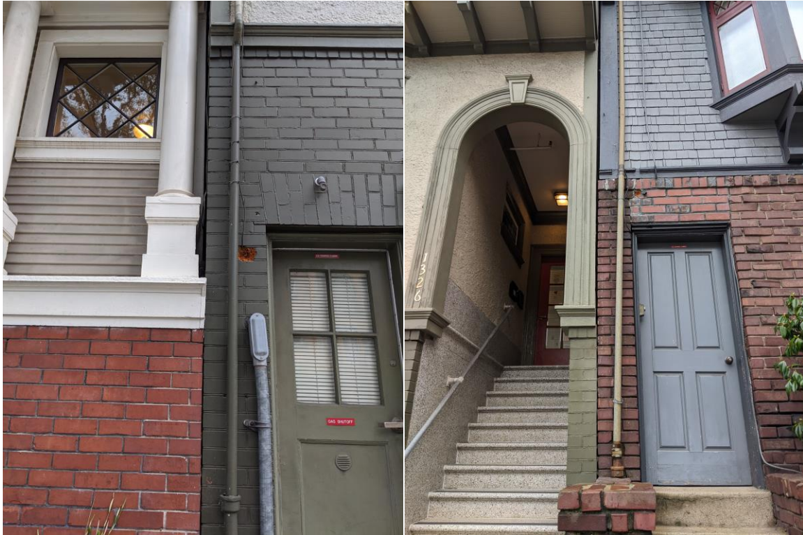
Figure 6 - Building Separation to the North (Left) and South (Right)
