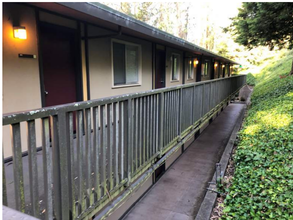
Figure 6. – Second Floor Balcony
