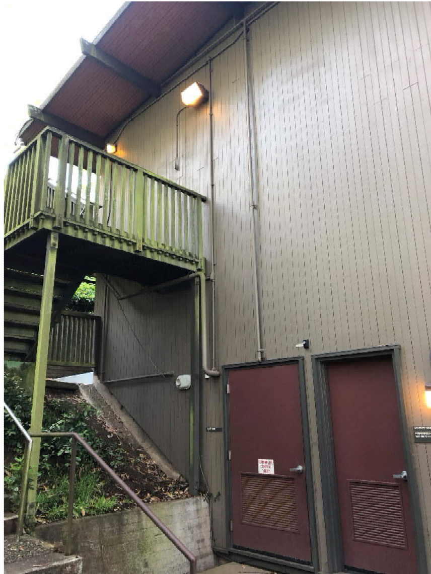
Figure 9. – Exterior Stairway on West Side
