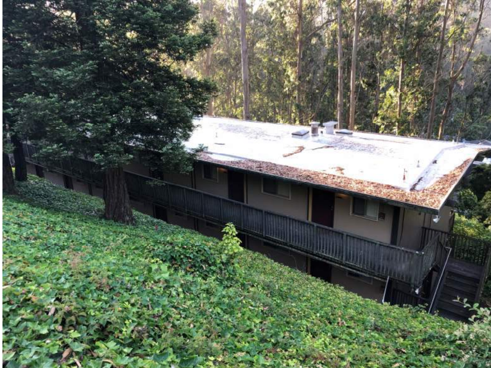
Figure 5. –Exterior of Building Facing East
