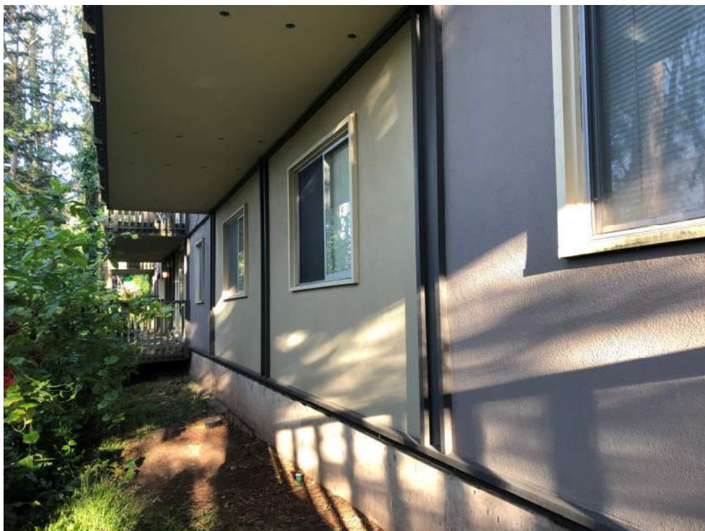
Figure 8. – Basement Exterior on South Side
