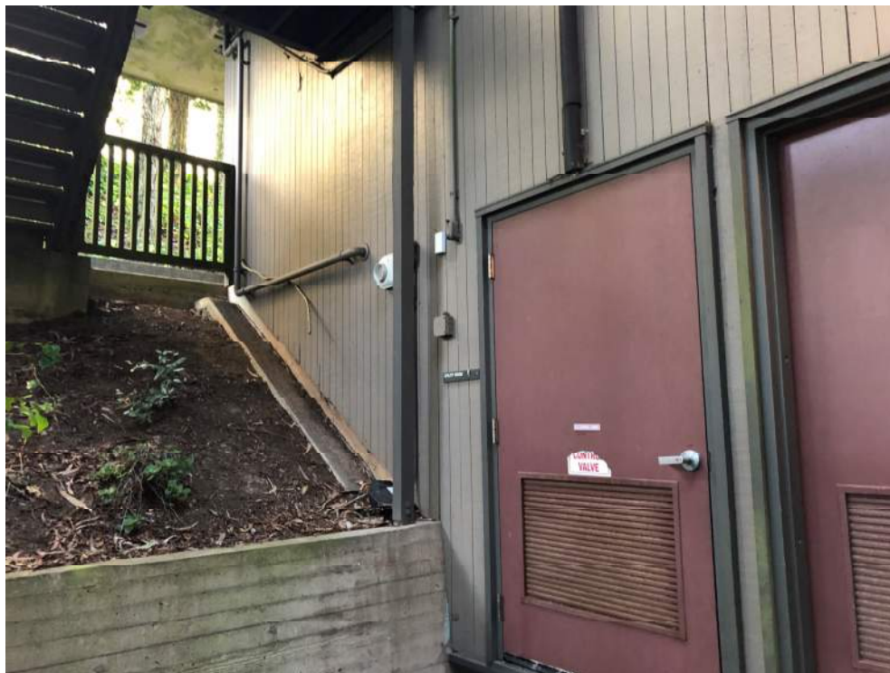
Figure 8. – Exterior Under Stairway on South Side
