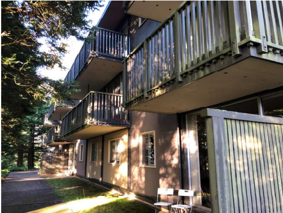
Figure 9. – Balconies on East Side
