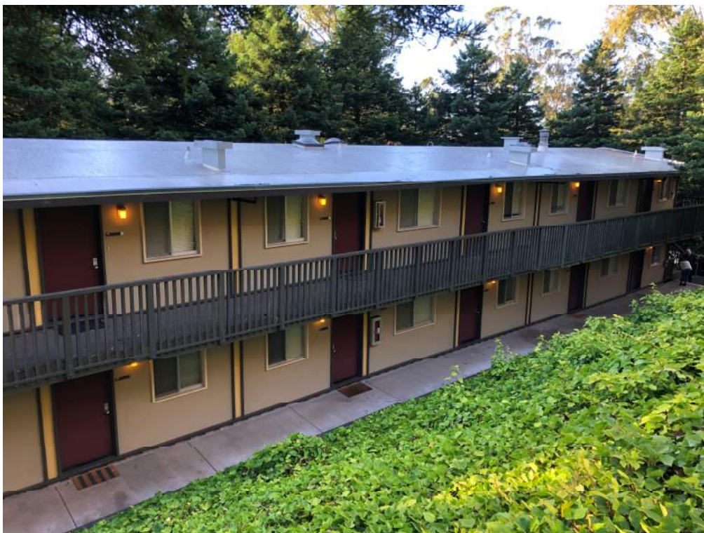
Figure 6. – Exterior of First and Second Floors on West Side
