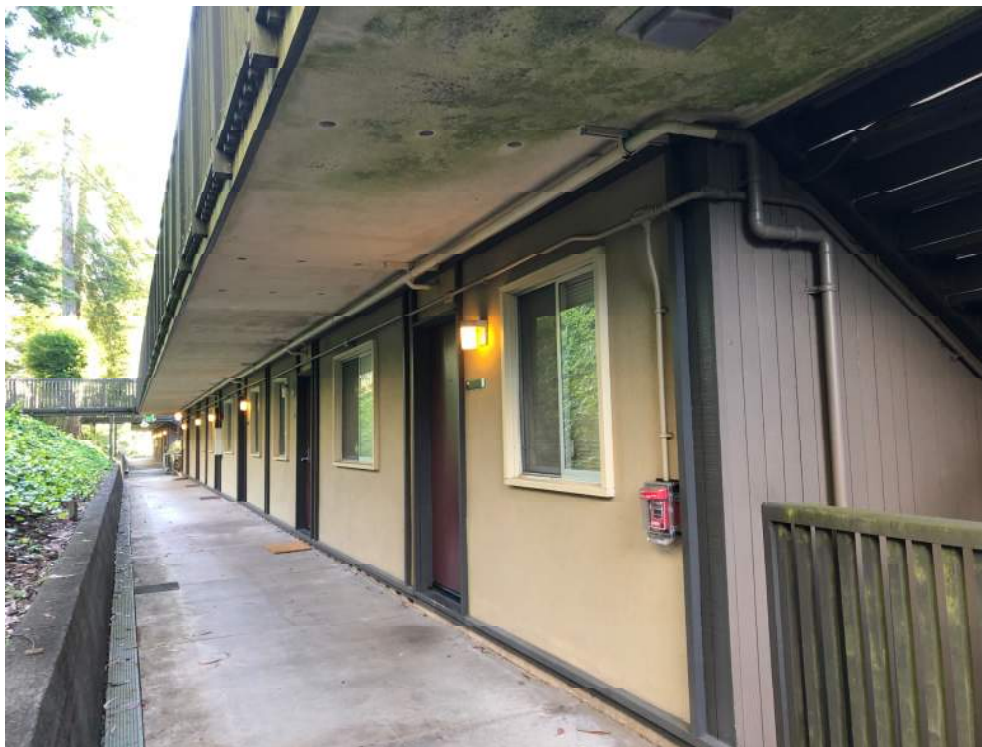
Figure 10. – First Floor Balcony on West Side
