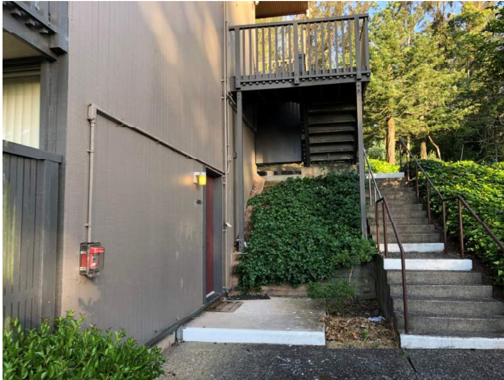
Figure 9. – Stairway on North Side
