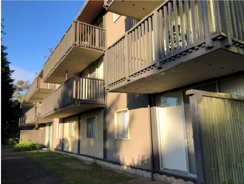
Figure 11. – Balconies on East Side
