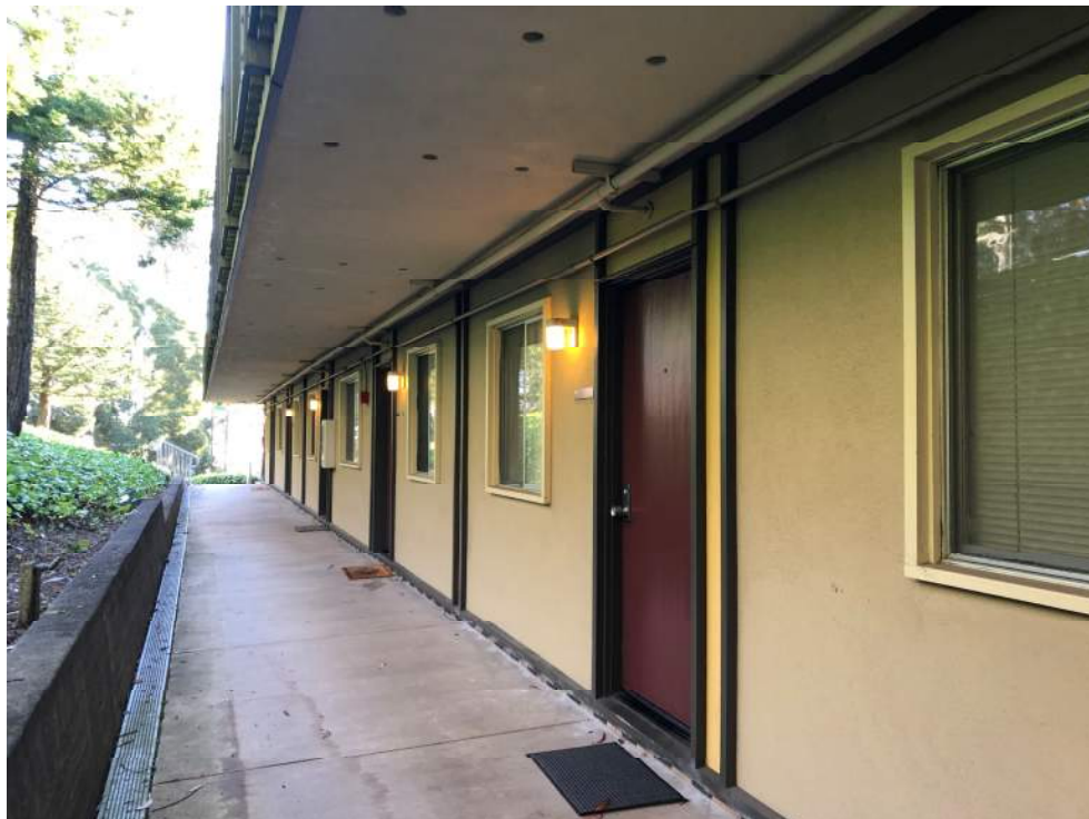
Figure 8. – First Floor Balcony on West Side
