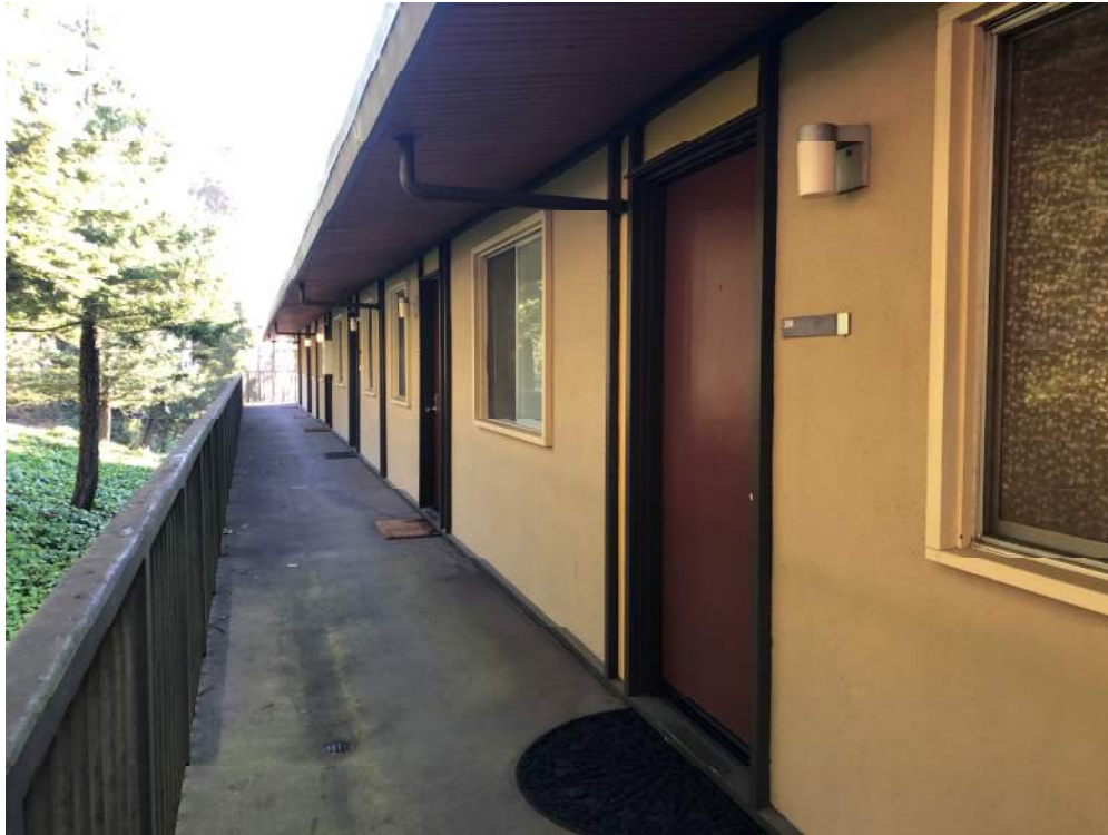
Figure 7. – Second Floor Balcony on West Side
