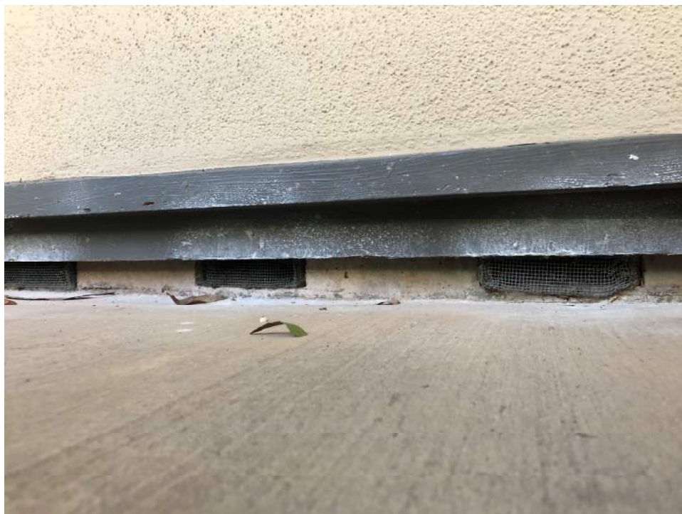
Figure 14. – Vents on Base of First Floor on West Side
