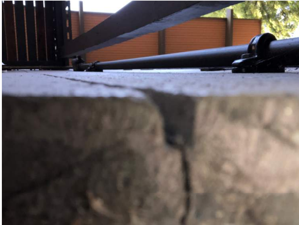
Figure 13. – Underneath Stairway on South Side
