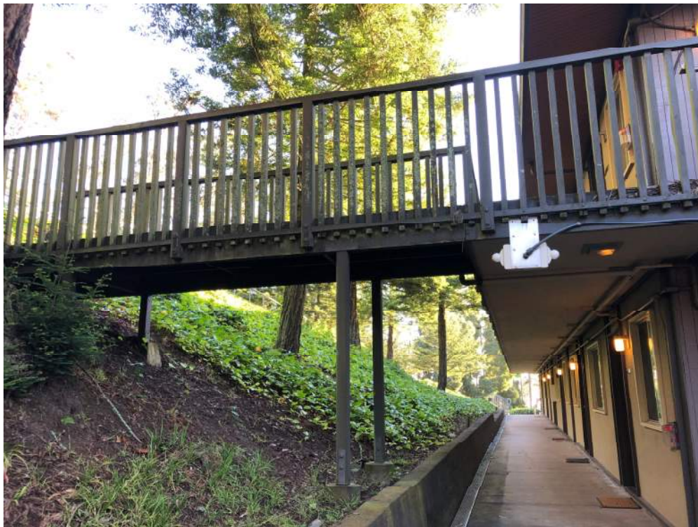
Figure 12. – Balconies and Walkway on West Side
