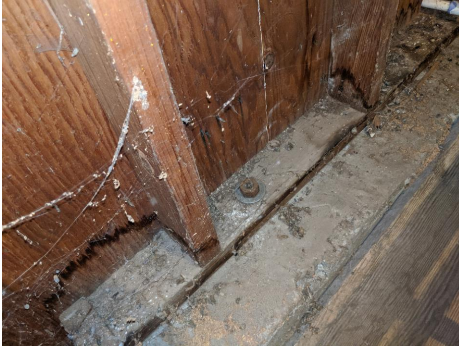
Figure 10 - Crawl Space Anchor Bolts, Plywood Sheathing
