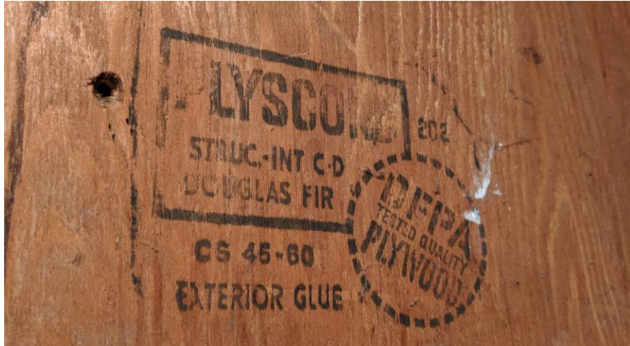
Figure 8 - Plywood Grade Stamp in Crawl Space
