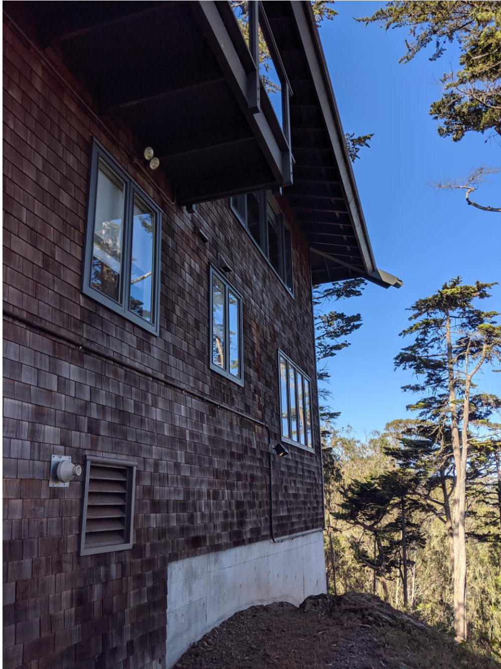
Figure 11 - North Building Elevation (Looking South)
