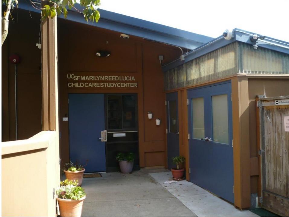
Partial south elevation (looking northeast)
