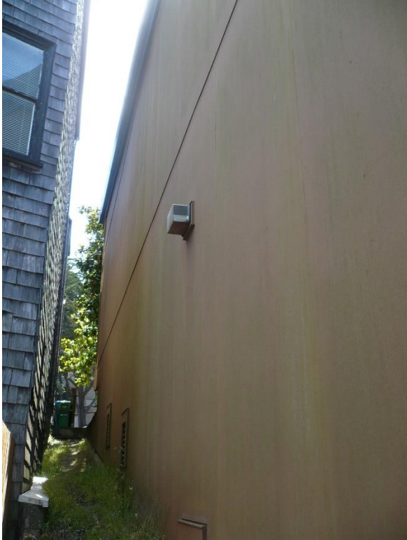
North elevation (looking east)
