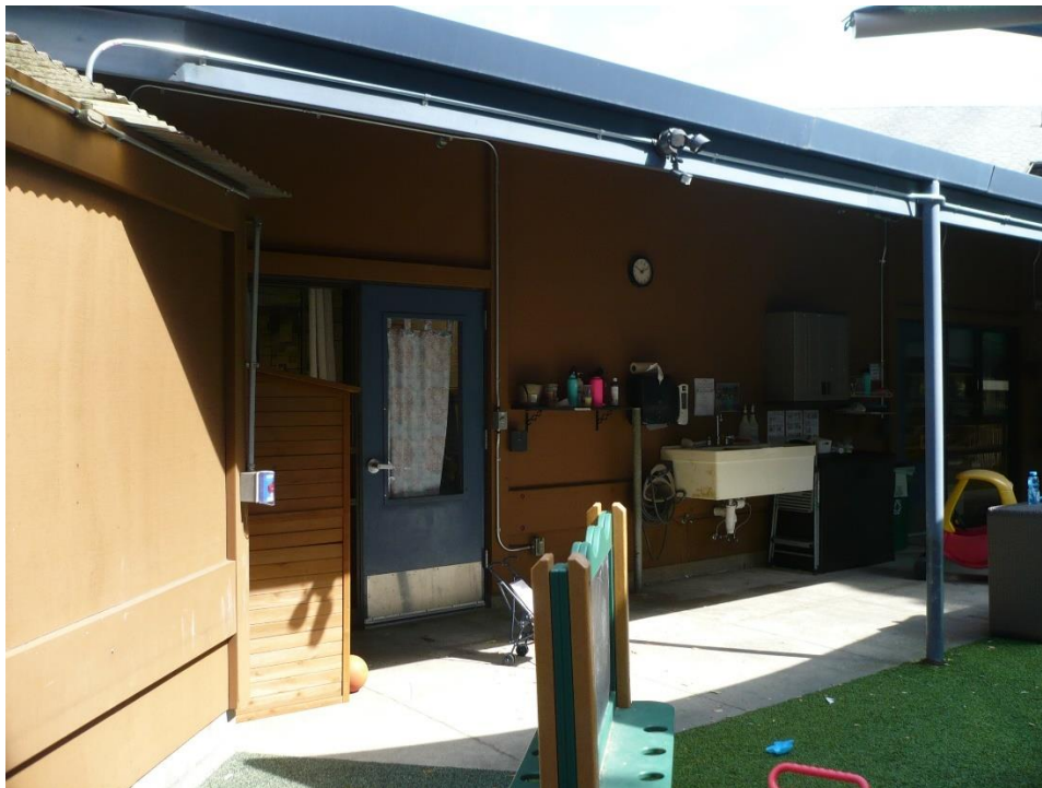
Partial east elevation (looking north)
