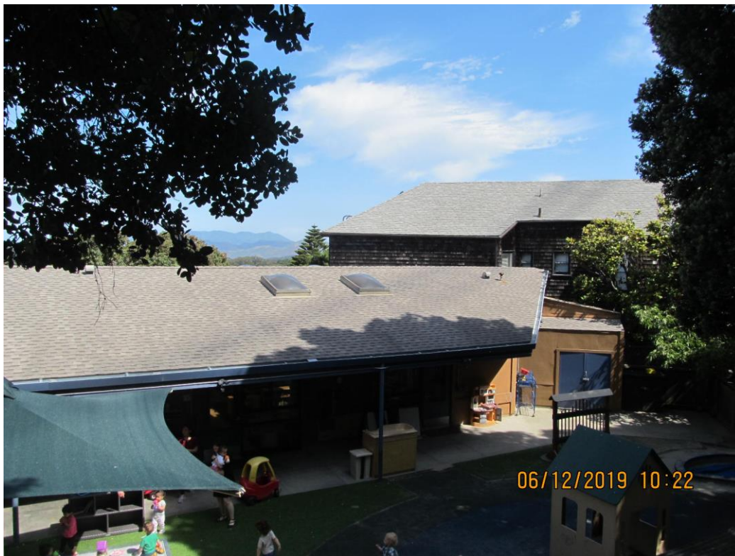
Roof (looking northeast)
