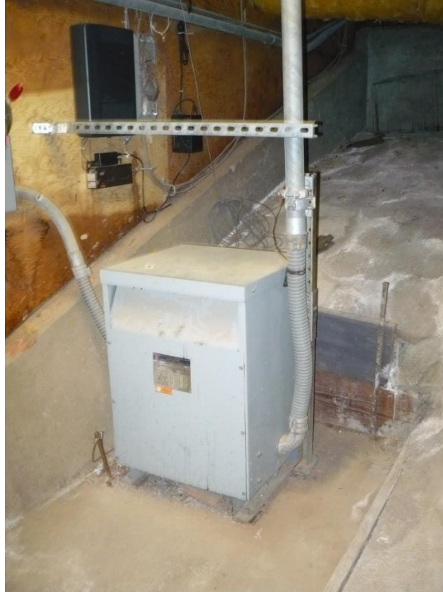
Basement mechanical area with rat slab beyond (looking east)
