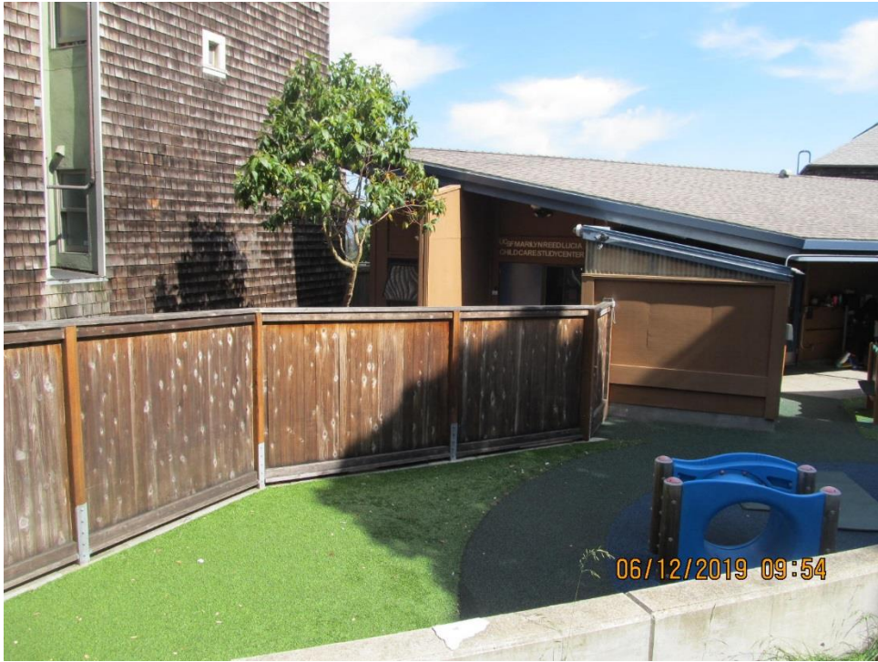
South elevation (looking north)
