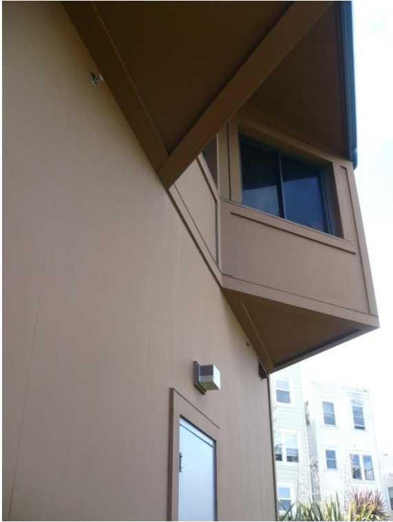
West elevation (looking southwest)
