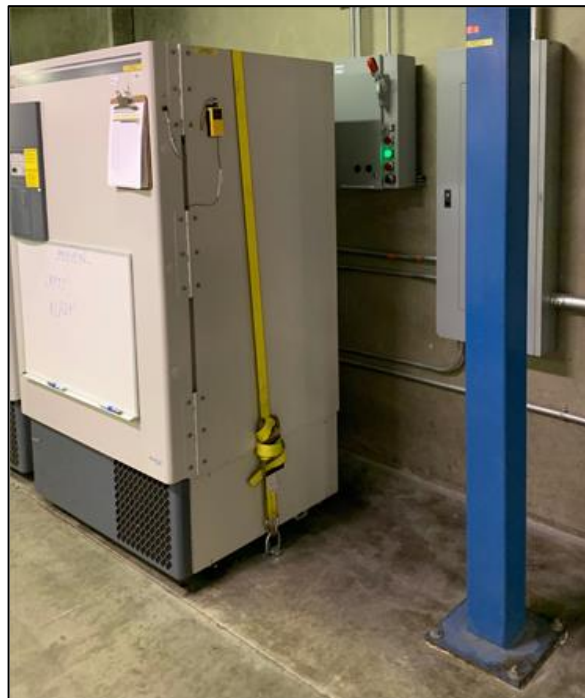
Figure 20 - Freezer Anchorage
