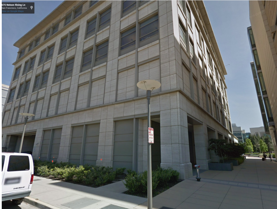
Northwest Corner (Google Street View, looking south)
