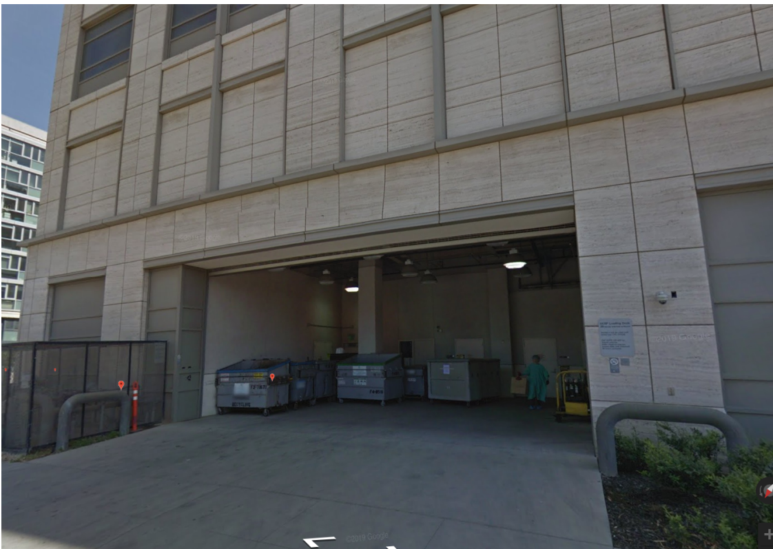
North Elevation at Loading Dock (Google Street View, looking south)
