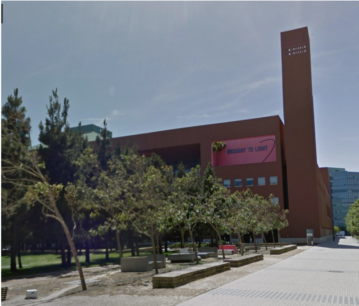
East Elevation with Tower at Northeast Corner (Google StreetView, looking south)
