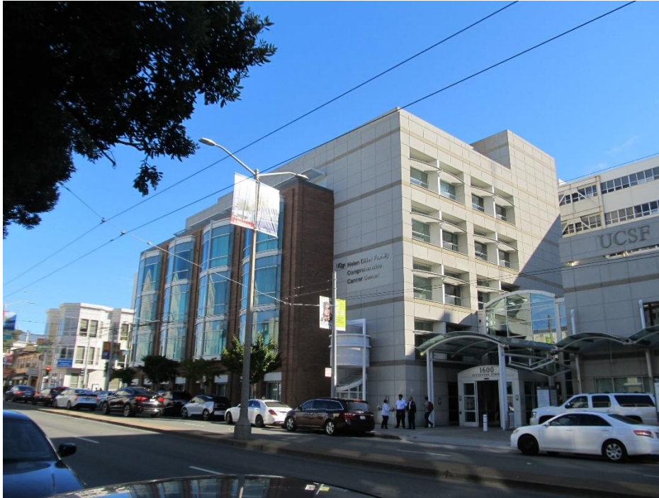
West and south elevation (looking northeast)
