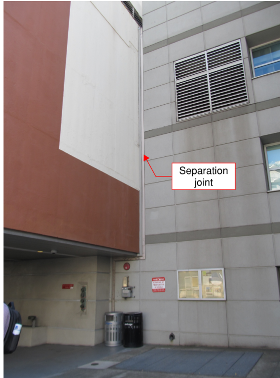
Separation joint between the Cancer Center and Building 'B' (looking southeast)
