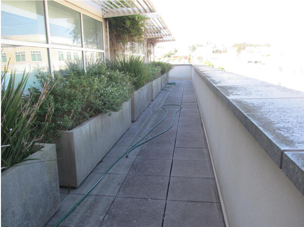
Balcony at the fifth floor (looking west)
