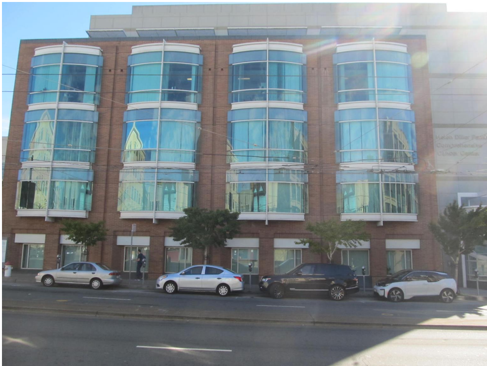
West elevation (looking east)
