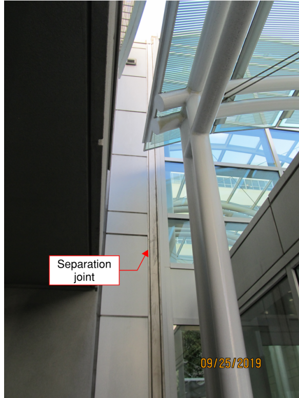
Separation joint between the Cancer Center and Building 'R' (looking east)
