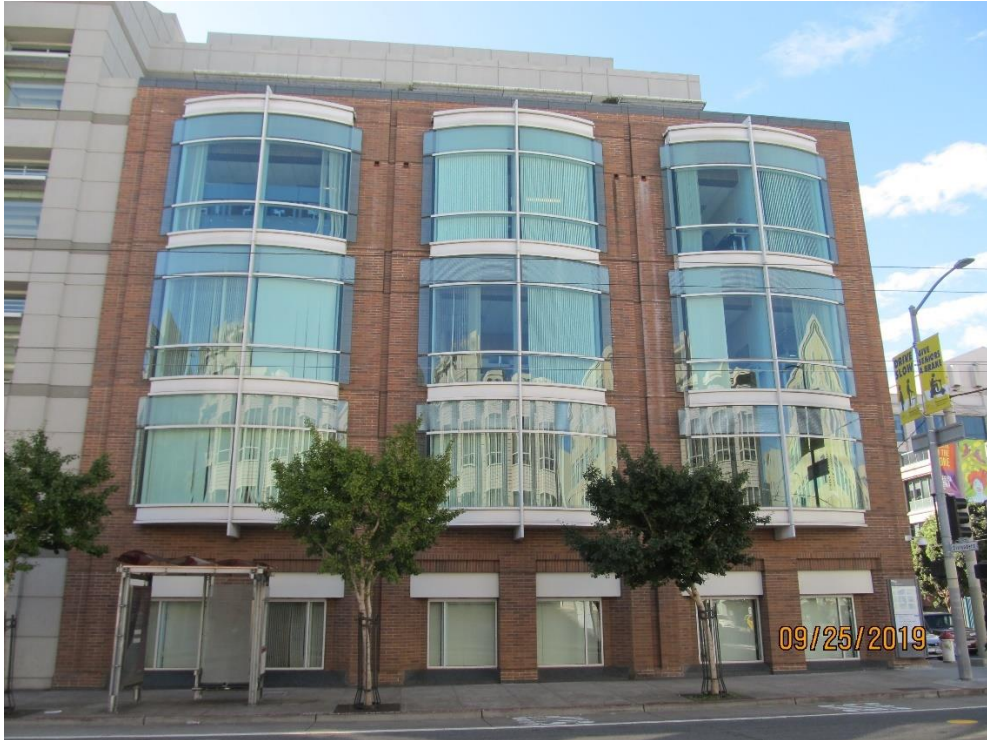
North elevation (looking south)
