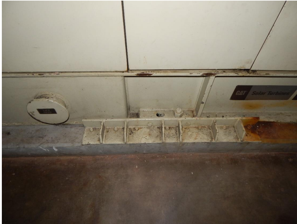
Photo 1. Gas Turbine Anchorage
