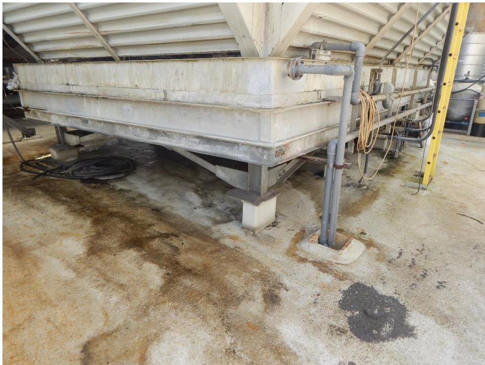
Photo 18. Auxiliary Cooling Tower Base
