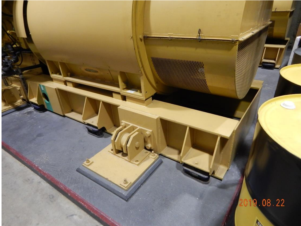
Photo 11. Diesel Generator Anchorage
