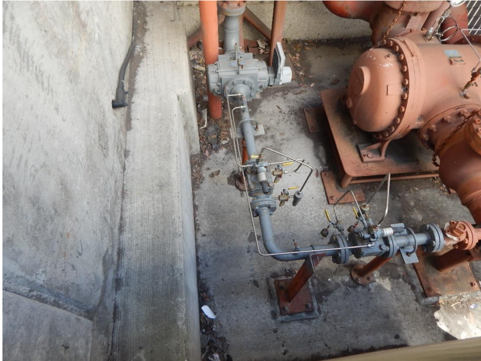
Photo 9. Gas Pump Anchorage
