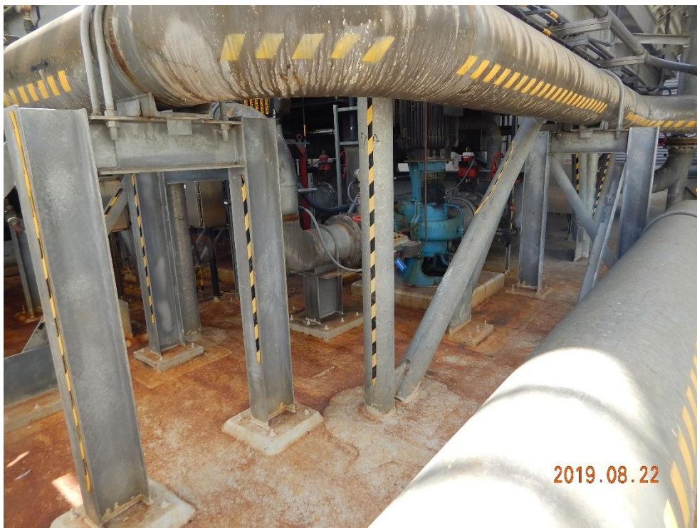
Photo 20. Pipe Bracing Frames
