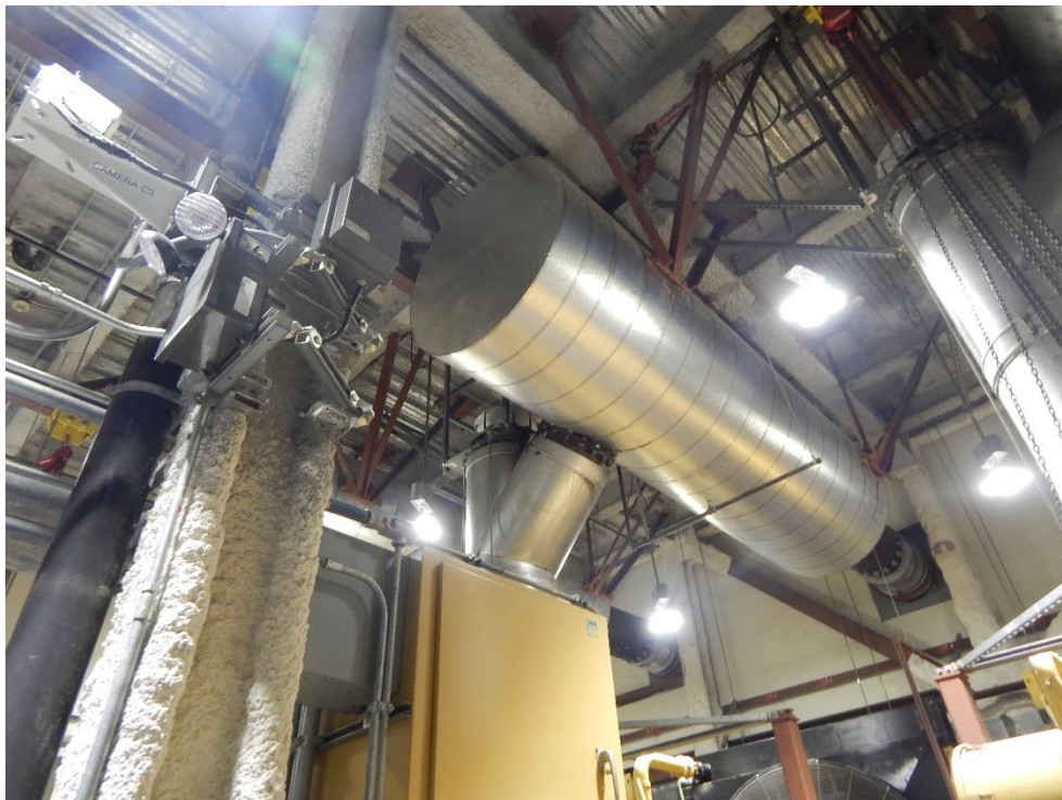
Photo 12. Generator Duct Bracing
