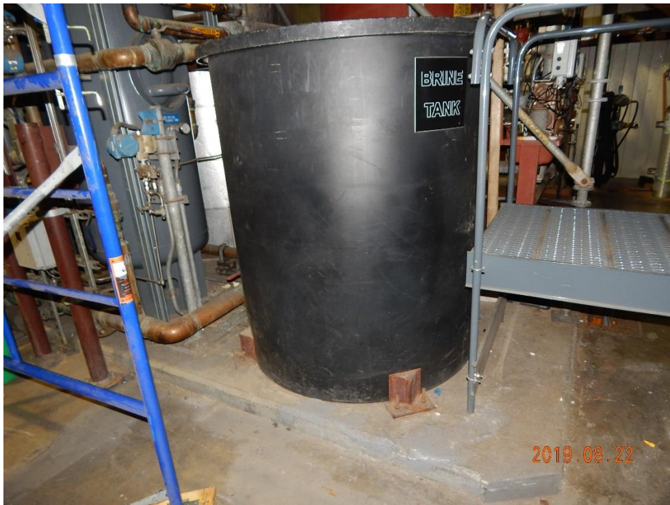
Photo 14. Brine Tank Anchorage
