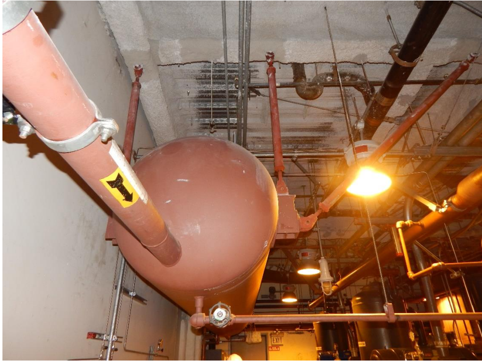
Photo 7. Tank Bracing
