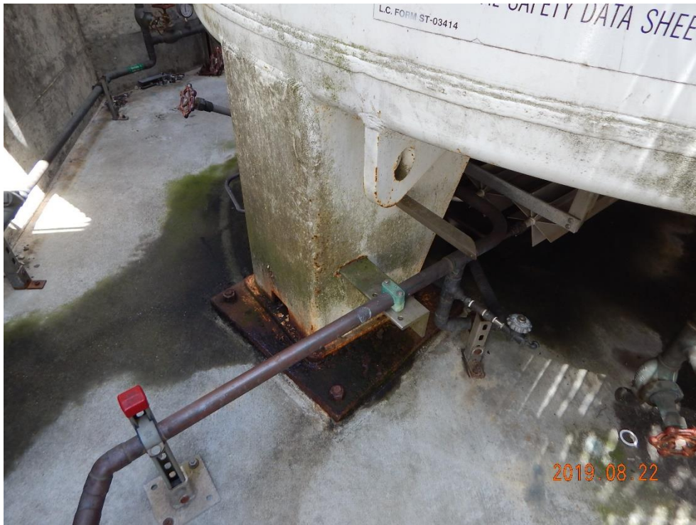
Photo 10. Oxygen Tank Anchorage
