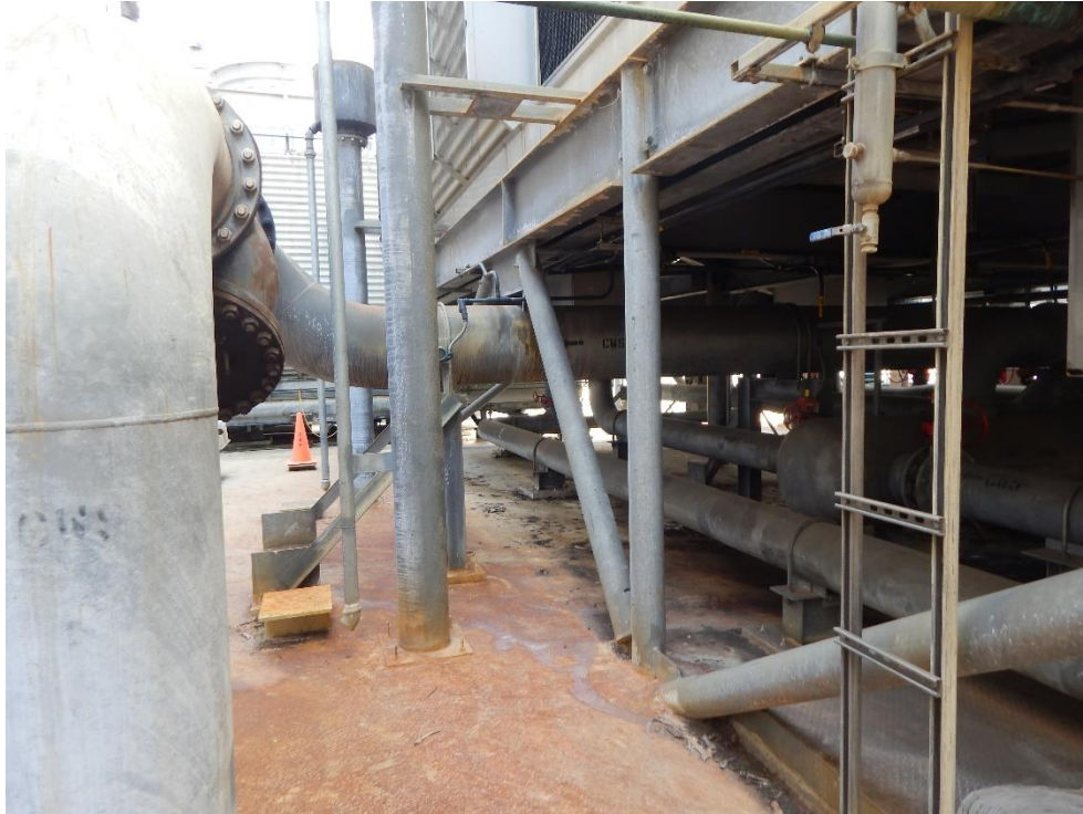
Photo 25. Cooling Tower Base
