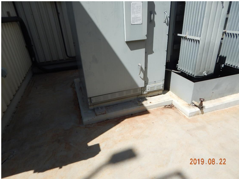
Photo 24. Transformer Anchorage
