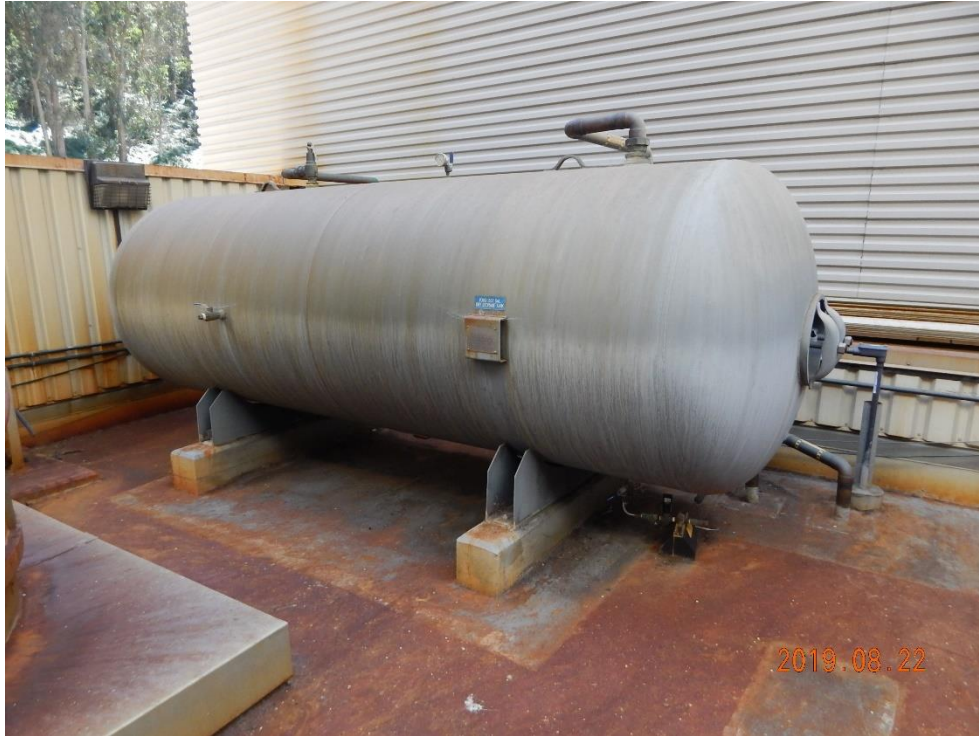
Photo 23. Storage Tank Anchorage
