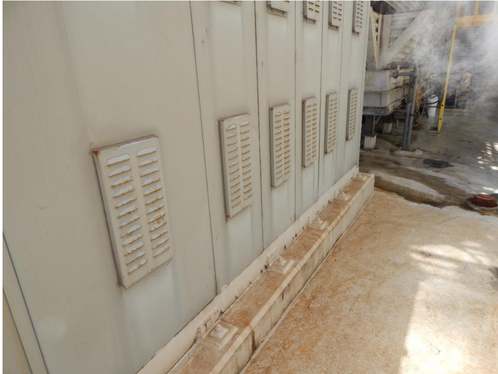
Photo 17. Substation Anchorage
