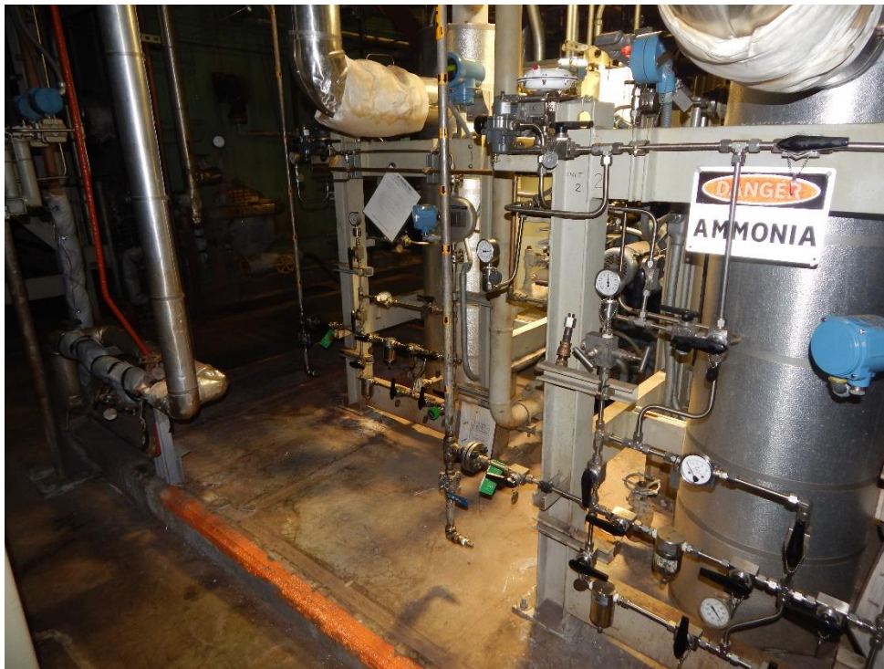
Photo 2. Ammonia Tank Anchorage
