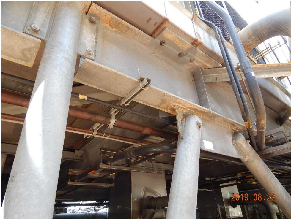
Photo 26. Cooling Tower Base
