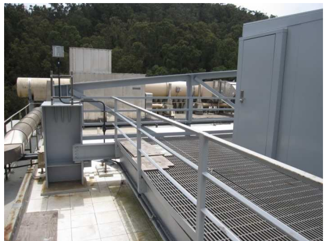
Figure 27: HSE roof equipment bridge column support.
