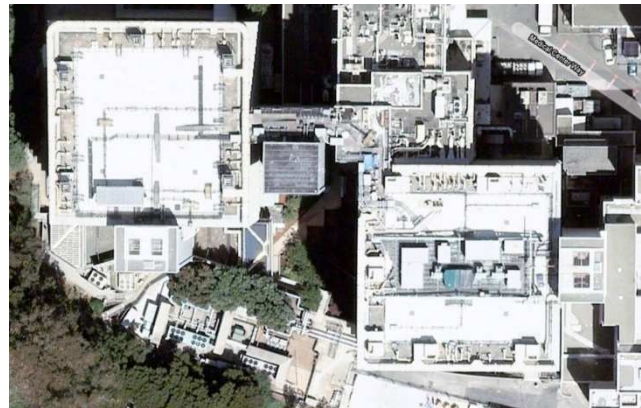
Figure 5: HSIR building satellite view. ©2009 Google, ©2009 GeoEye
