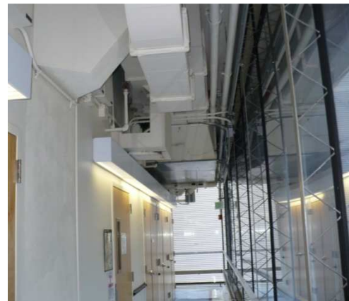
Figure 98: Typical interior view of laboratory building window glazing.
