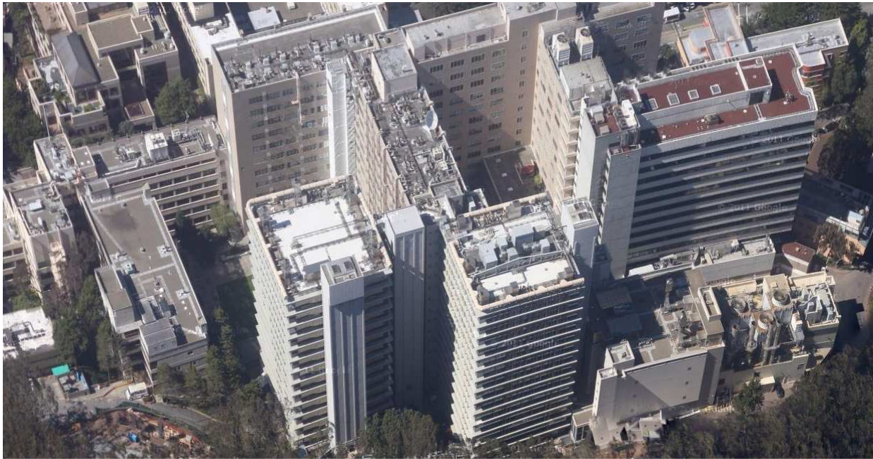
Figure 6: View of Health Sciences building complex and adjacent buildings. © 2011 Google
