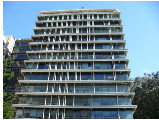
Figure 83: Typical exterior fume exhaust duct risers – HSW north face.
