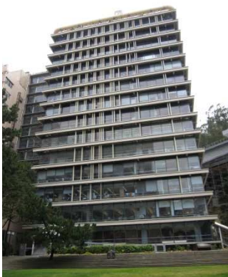
Figure 96: Exterior view of laboratory building window glazing.
