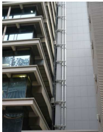
Figure 97: View of window glazing a laboratory building corner
