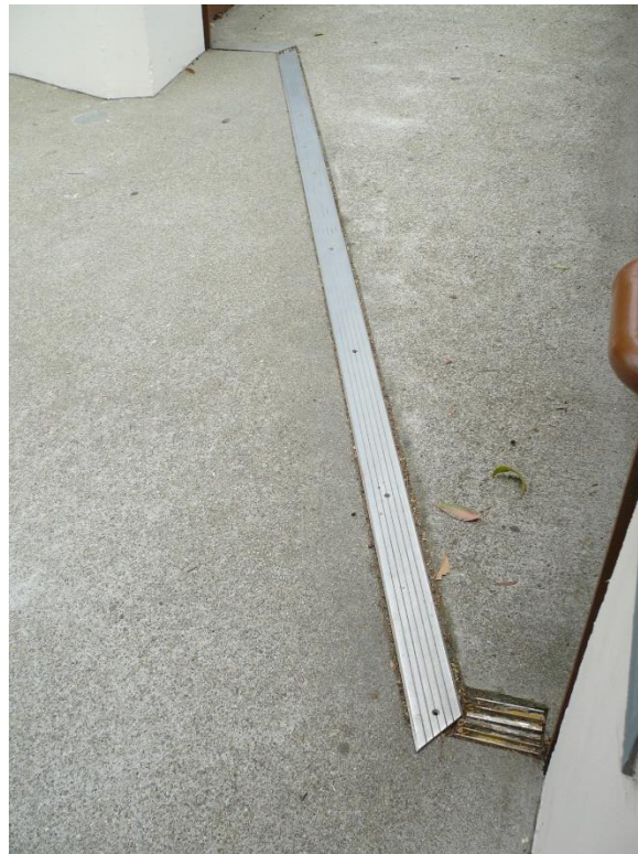
Seismic joint cover on the west end of the pedestrian bridge
