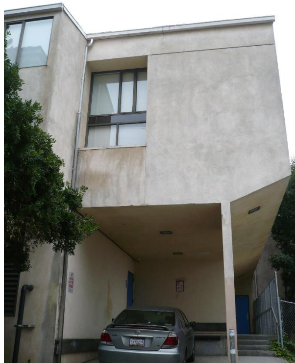
Partial south elevation (looking north)
