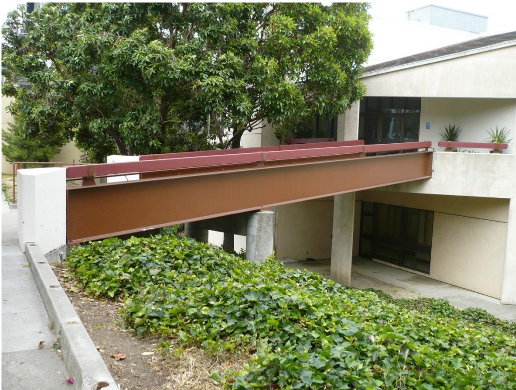
Pedestrian bridge at main entry (looking northeast)
