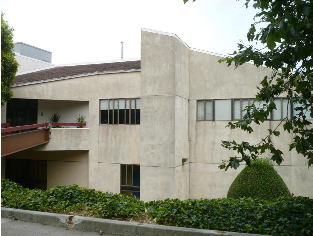
West elevation (looking northeast)
