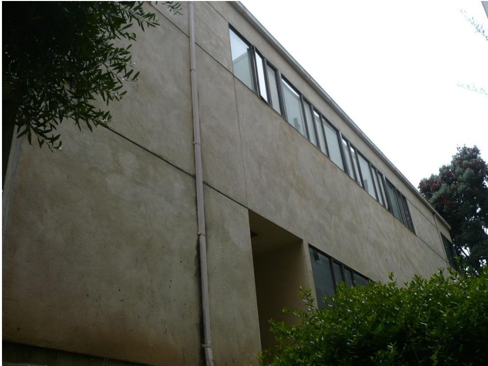
North elevation (looking northwest)
