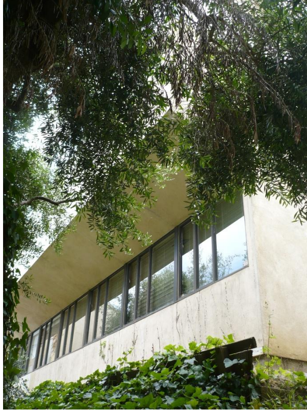
Overhang on east elevation
