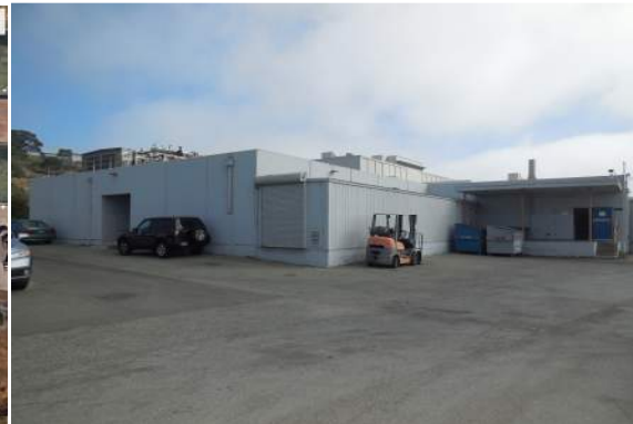
West elevation (looking northeast)
