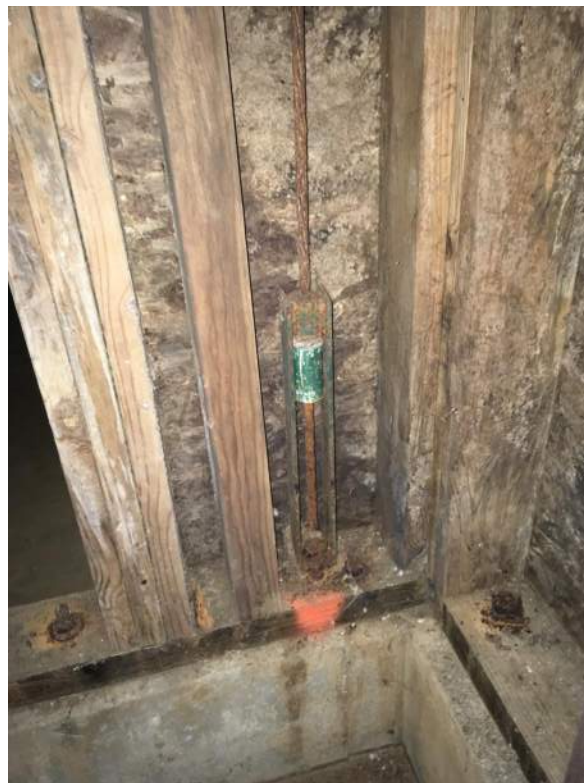
Figure 9. – Typical holdown in crawlspace
