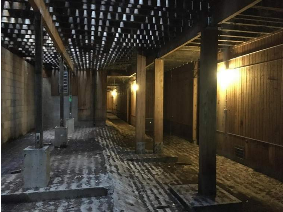
Figure 8. – Walls in crawlspace
