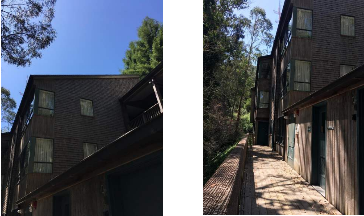
Figure 7. – Northern elevation and walkway on eastern side
