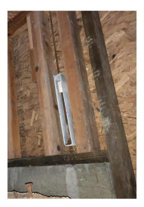
Figure 9. – Typical holdown in crawlspace
