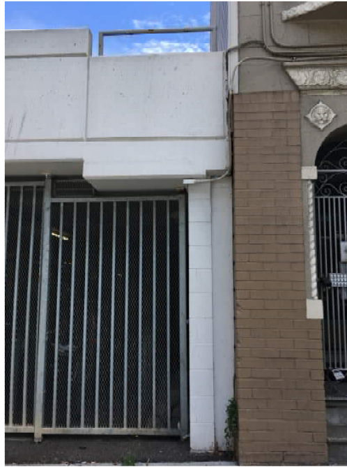
Figure 1. – 3-story wood building adjacent to parking garage.
